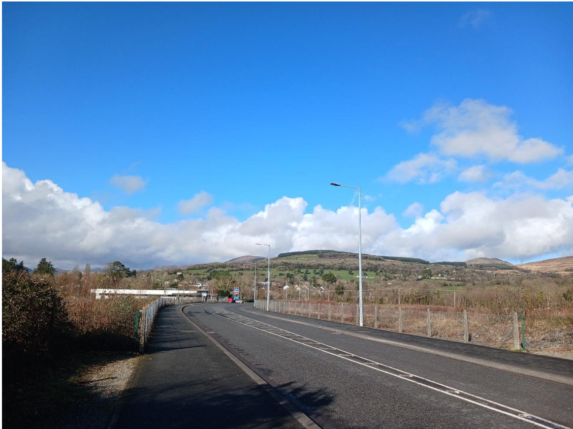
Photo A3: Existing Public Lighting on Pat Scarteen Road
