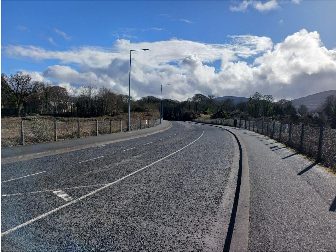
Photo A5: Existing Road marking on Pat Scarteen Road
