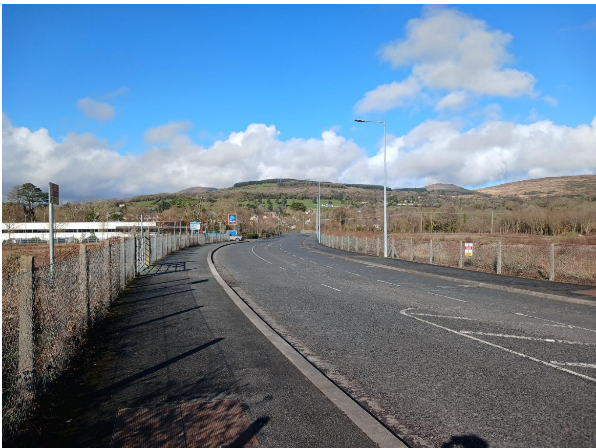
Photo A4: Existing Road marking on Pat Scarteen Road
