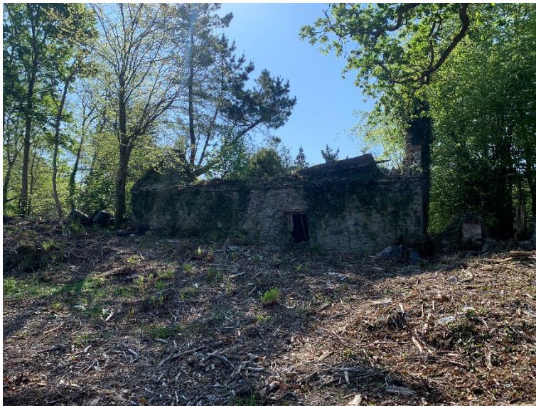
Plate 3-2: Ruinous Dwelling at the Southeast of the Study Area
