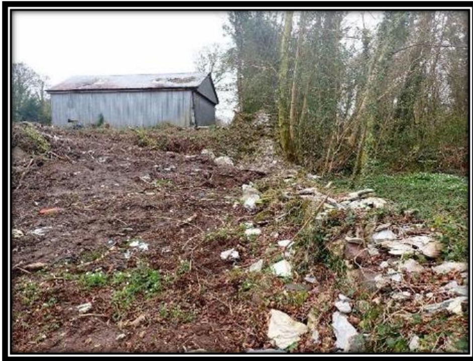
Plate 7: Stone Wall and Other Stonework (BL1) along the Southwestern Boundary.
