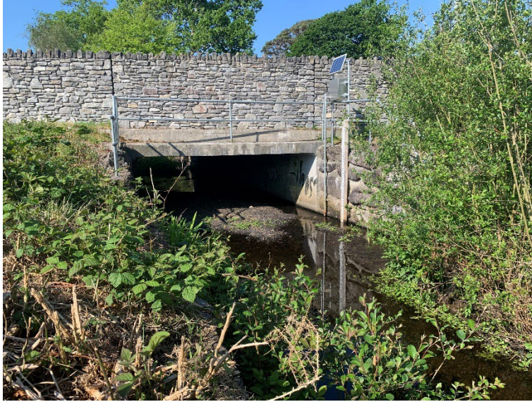
Plate 3-1: Concrete Slab Bridge over Lissaniska Stream
