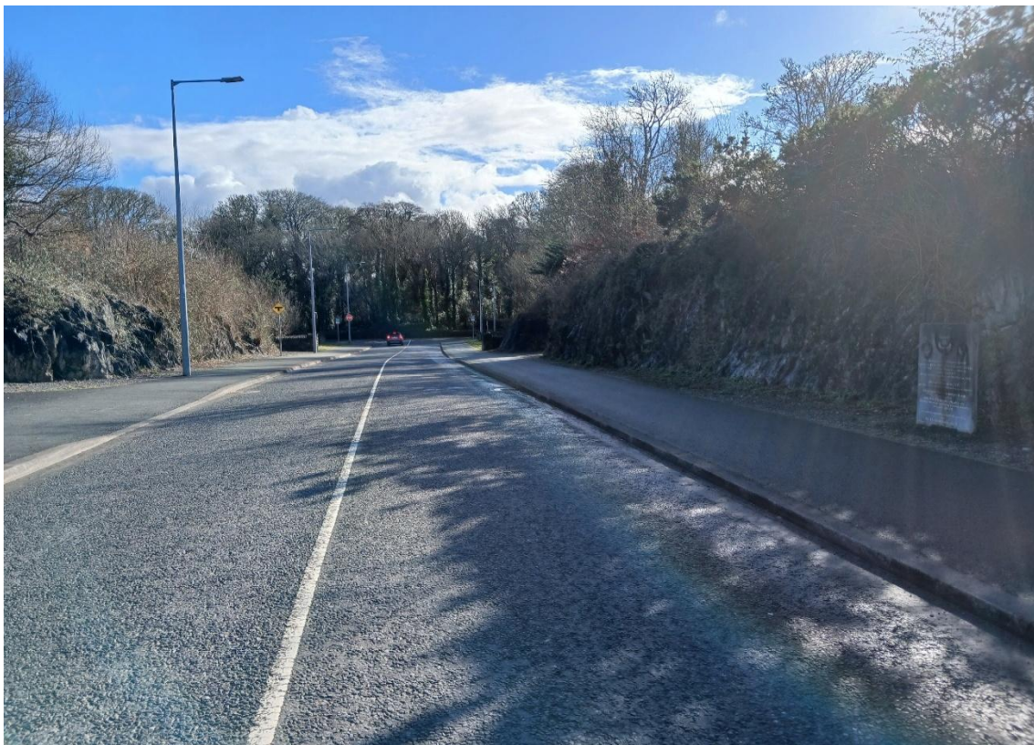
Photo C2 – Existing Shared Facility along Pat Scarteen Road
