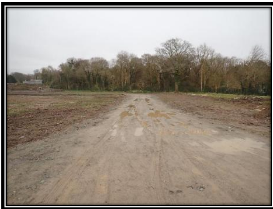
Plate 2: Spoil and Bare Ground (ED2)
