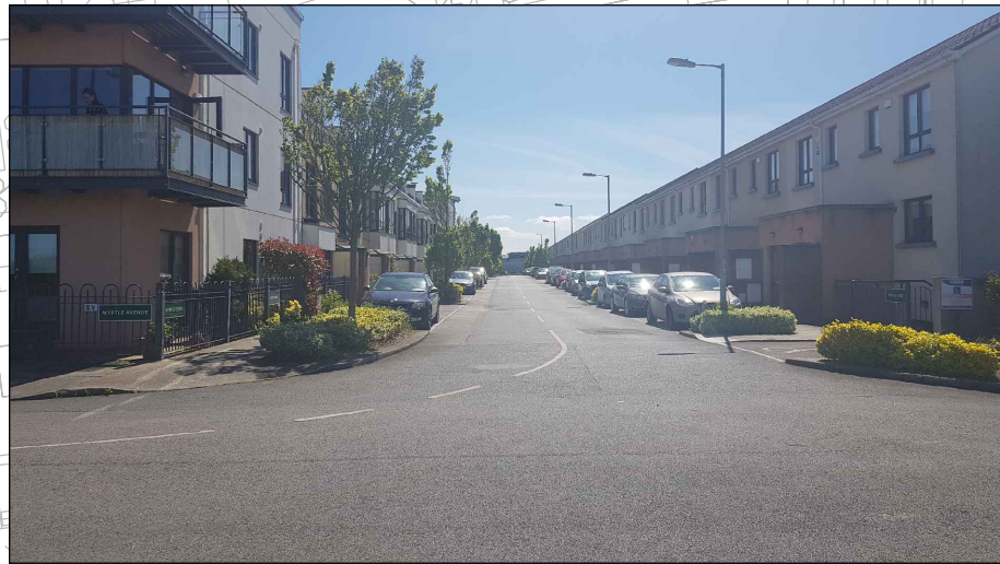
PHOTOGRAPH B. MYRTLE AVE. EASTBOUND.
