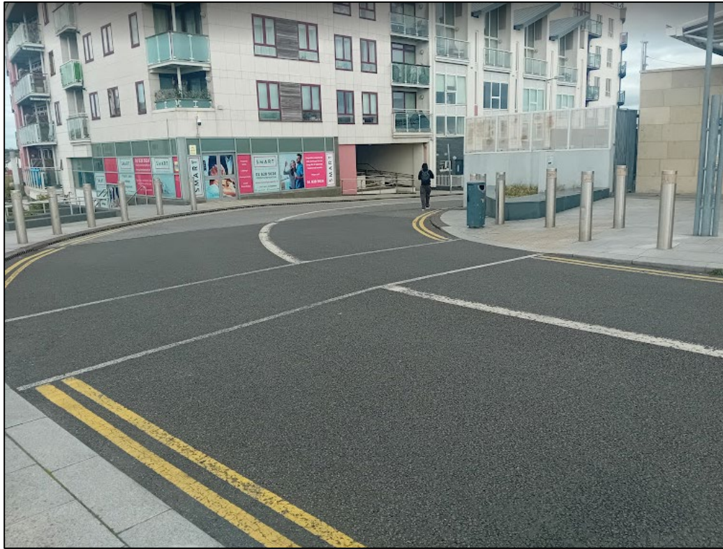
Figure 2.5 – Existing Tie-in at Railway overbridge as observed on site visit
