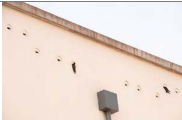
Example of installed Swift bricks in use.
