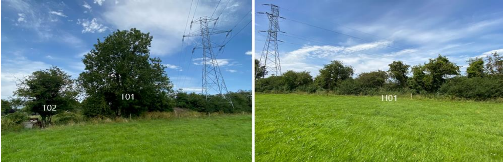
Fig 2 - Section of Hedgerow 01 to the east of Pylon – Trees T01 & T02 to west of Pylon
