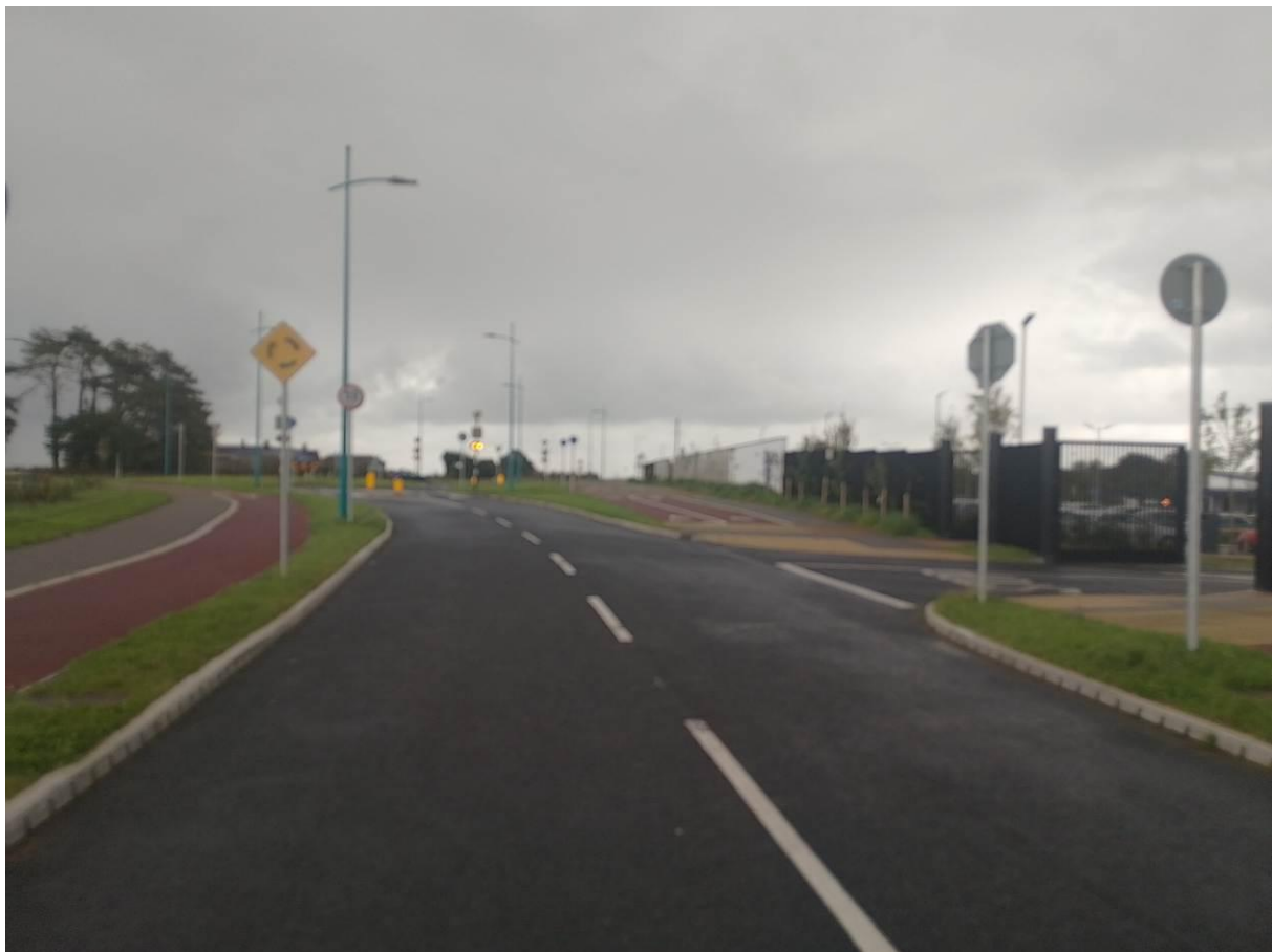
Photo A2 – Existing Public Lighting Columns along the existing scheme
