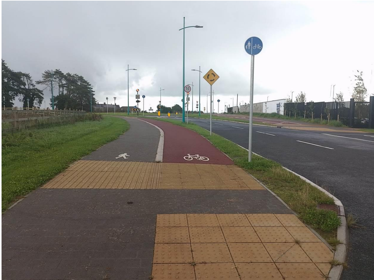
Photo A1 – Tie-in point to existing Active Travel Infrastructure
