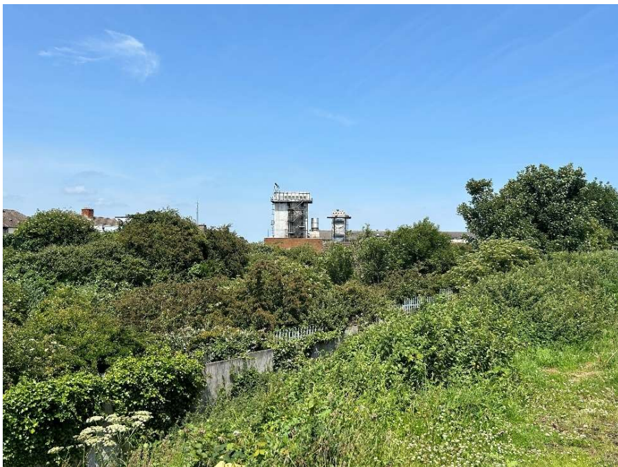
View looking northwest towards Batchelor's Industrial Facility
