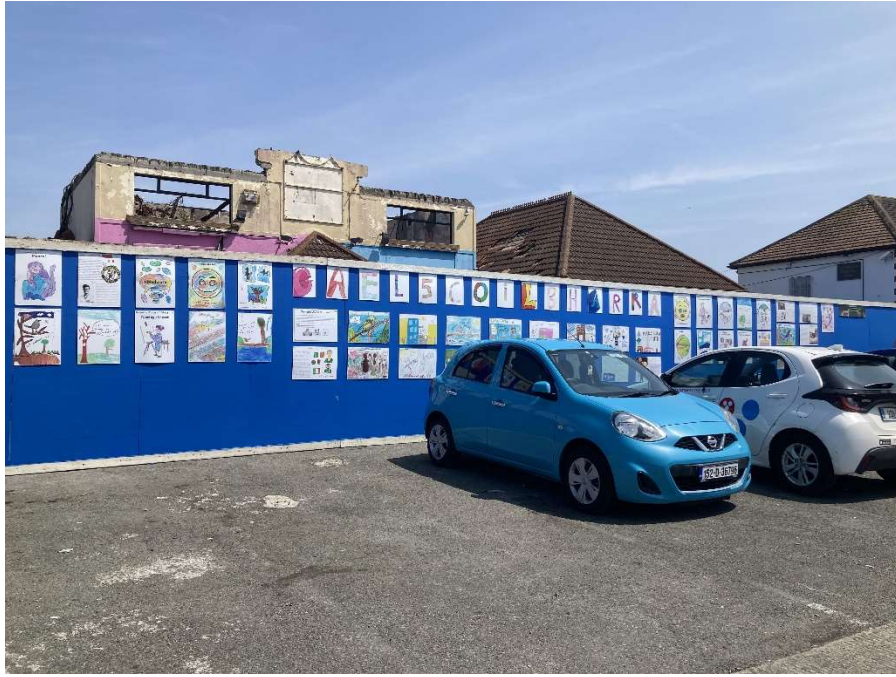
View from Fassagh Avenue looking north towards southern boundary of the site
