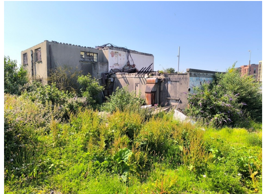
Plate 12: View of rear of public house, facing southeast
