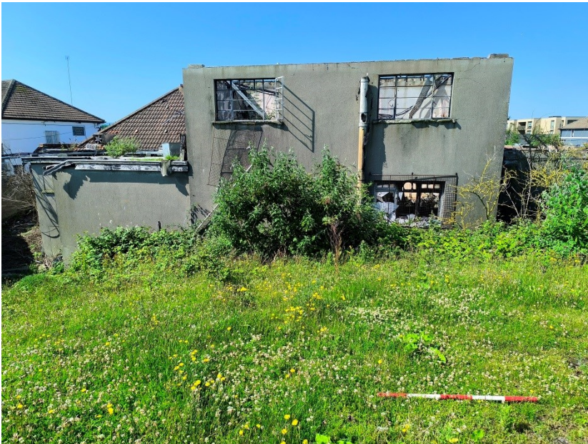
Plate 11: View of rear of public house, facing south
