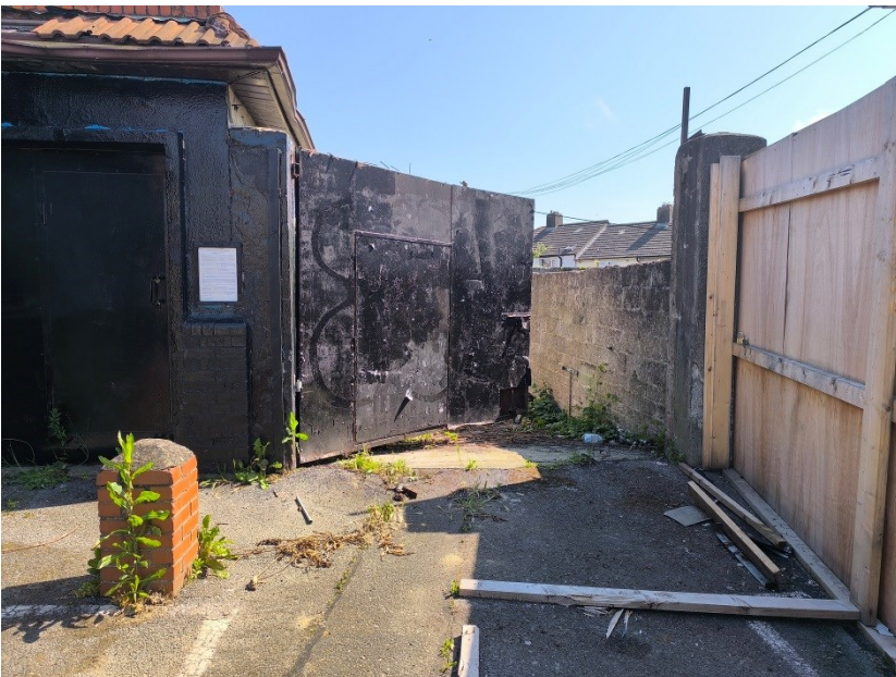
Plate 7: View of laneway access, facing northeast
