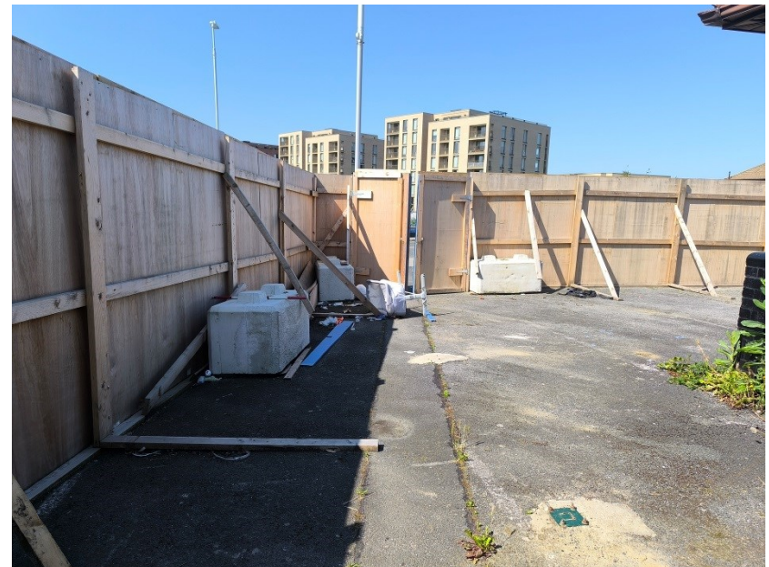
Plate 4: View of hoarding in front of site, facing southwest
