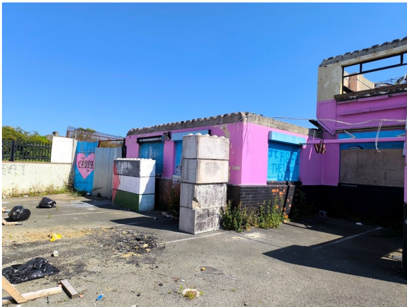
Plate 3: Front view of former Matt's of Cabra public house, facing northwest
