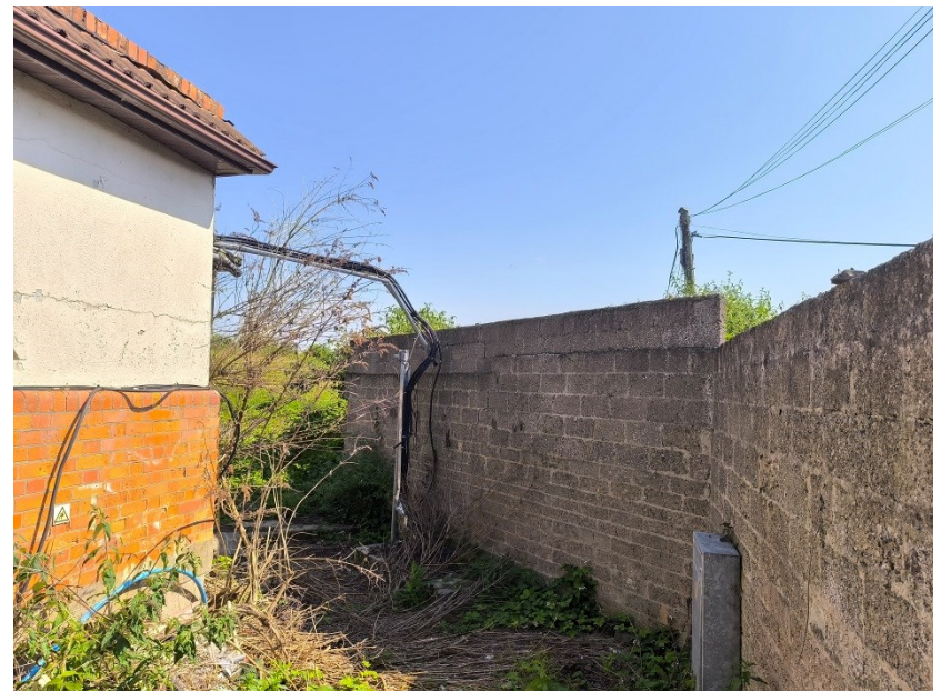
Plate 8: View of laneway providing access to rear of site, facing north-northeast
