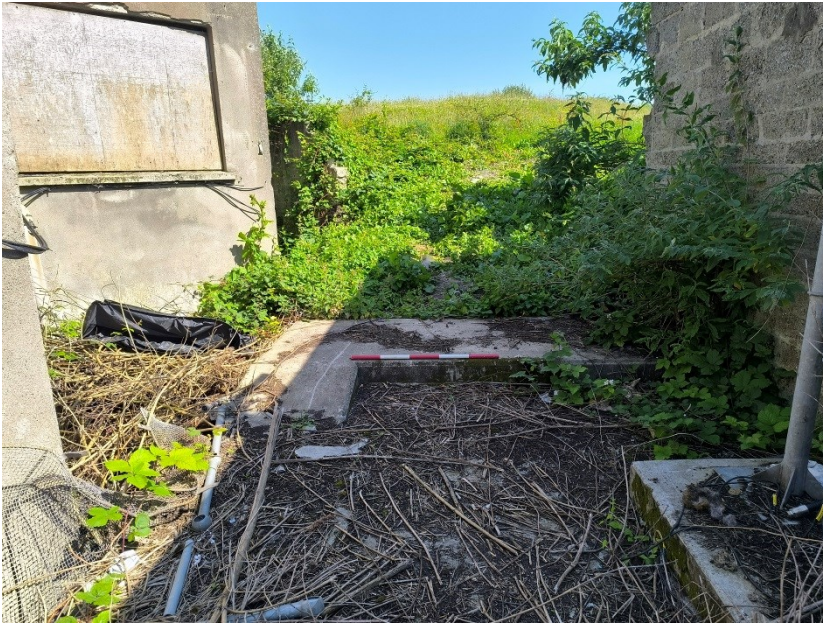
Plate 9: View from rear laneway looking to rear of site, facing northwest
