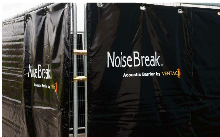
Figure 17: Temporary Construction Noise Barrier © Ventac
