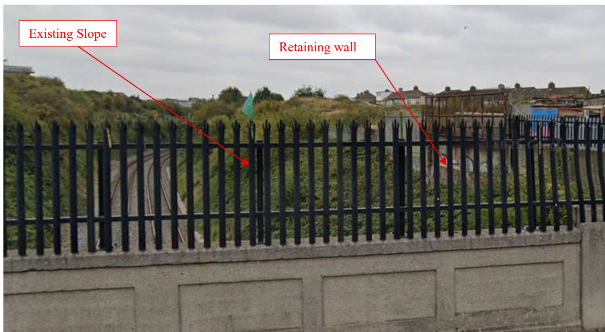
Figure 2-1: Photograph from Faussagh Avenue bridge facing north shown railway cutting slope (Google Maps, September 2024)
