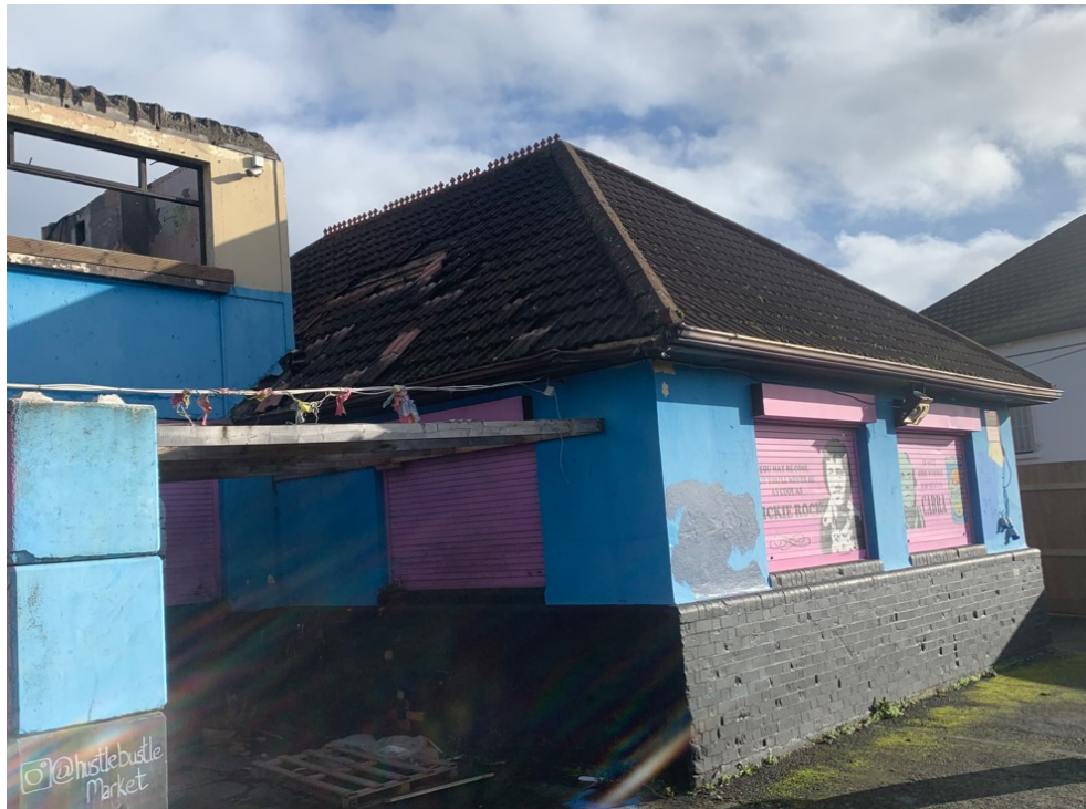
Figure A3: Front of Section 2
