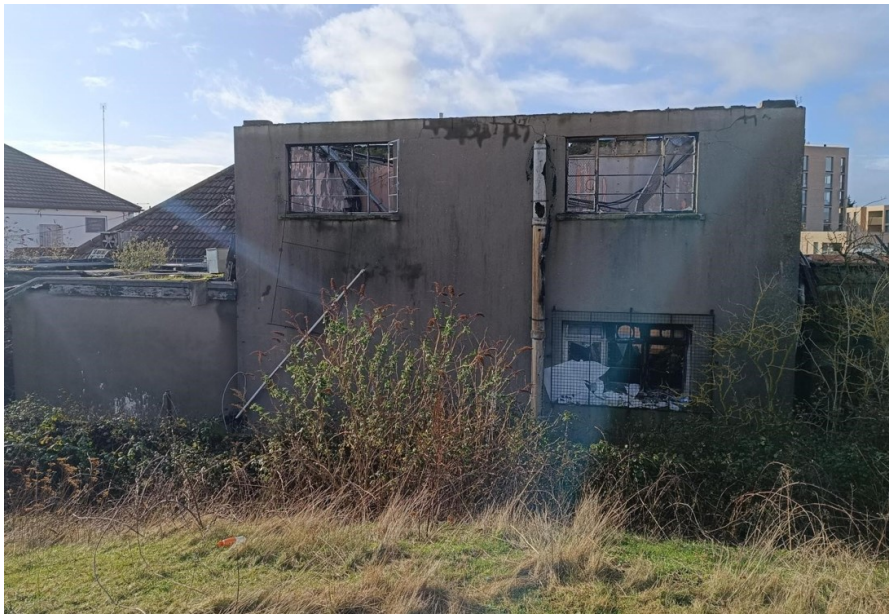
Figure A2: Rear of existing structure
