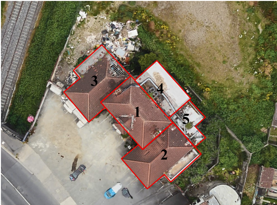
Figure 4.2: Aerial Photograph of Existing Buildings to be Demolished. (Source: Google Maps – Photo is outdated as it shows the now removed roofs of sections 1 & 3)
