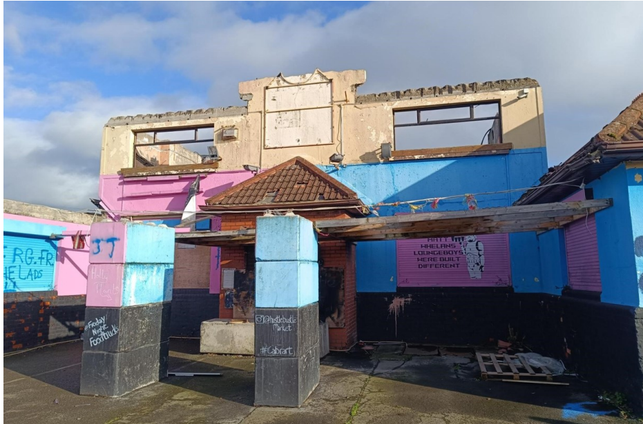
Figure A1: Front of Section 1 / Entrance to site
