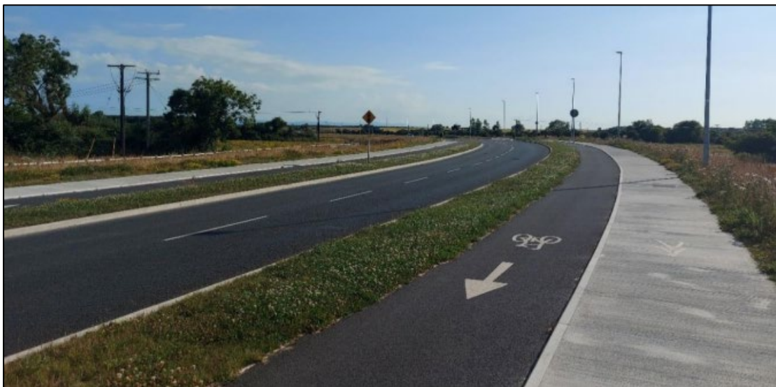
Figure 3-13: Existing Cycle and Pedestrian Facilities on the DDR (Source: TTA prepared by DBFL Consulting Engineers, 2024)
