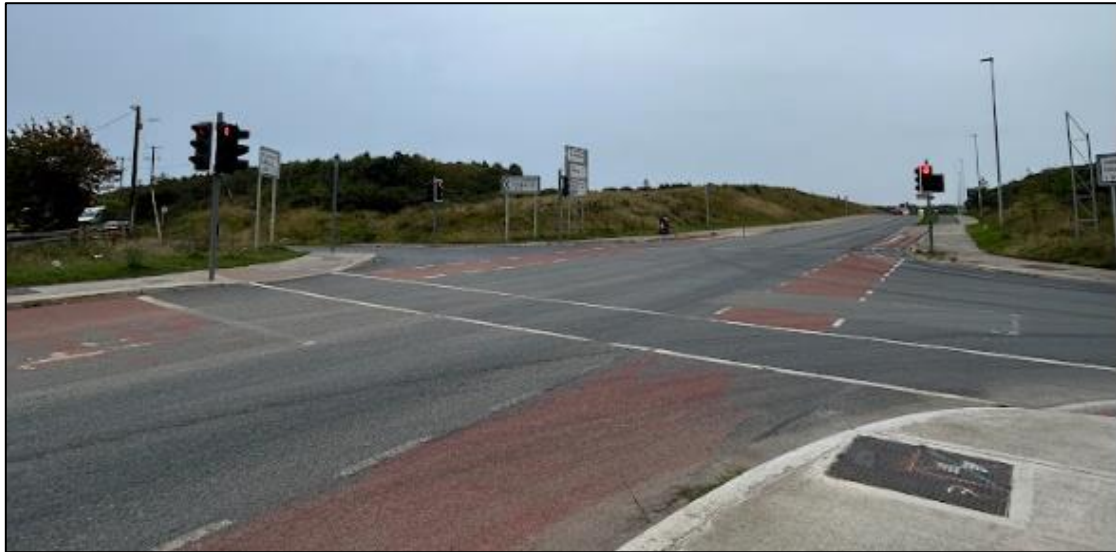
Figure 2-13: Pedestrian Crossing at the DDR/New Road Junction
