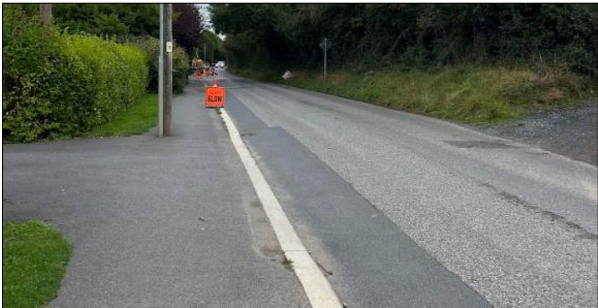
Figure 2-12: Existing Pedestrian Facilities on New Road
