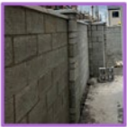
Concrete Block wall with Concrete Capping
