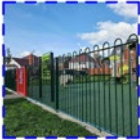
Playground Railing - Steel railings with gate
