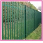
Palisade Fence - Security fence for pump station
