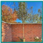
Brickwork wall - Facing public open space
