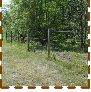
Timber Post and Wire Fence to Existing Hedgerow
