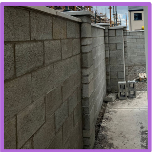
Concrete Block wall with Concrete Capping
