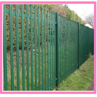
Palisade Fence - Security fence for pump station
