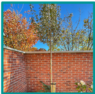
Brickwork wall - Facing public open space
