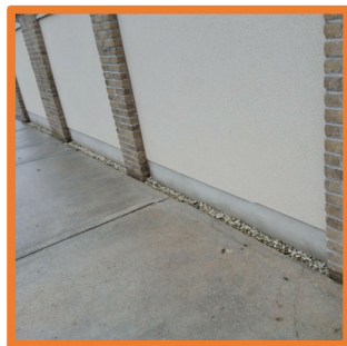
Blockwork wall with Brick Piers - Facing public realm
