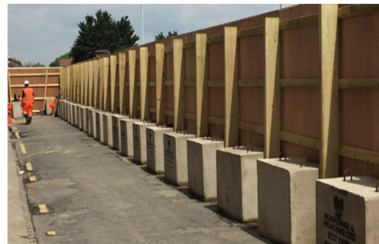
Figure 6.7: Example – Demountable 'Heras' fence and solid timber hoarding with ballast blocks
