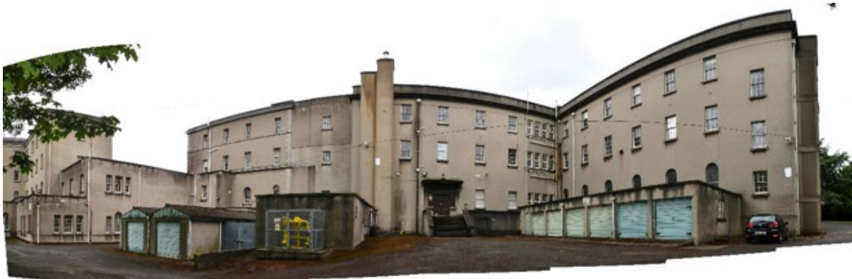
Figure 63: View of the rear facades of the new wing.
