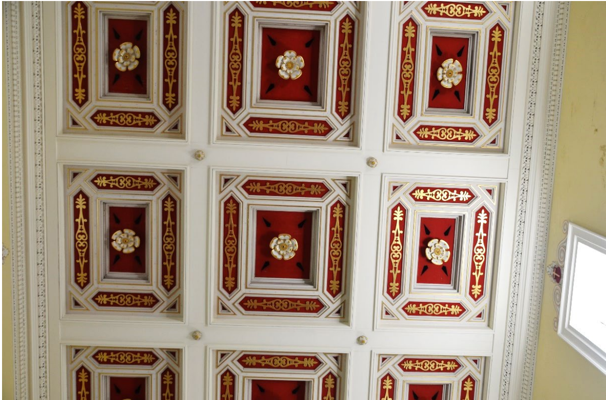
Figure 16: View of the panelled timber ceiling to the nave of the Church.
