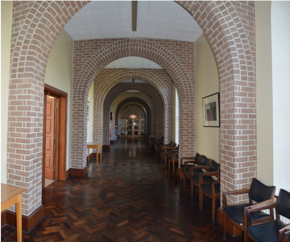
Figure 61: View of the late 20th century brick 'arches' at Ground Floor Level of the Main Seminary Block. The floors above and below are constructed in and supported by a steel and concrete frame. The brick visible here is a cladding which conceals the 1960s RSJs that intruded into Bourke's original corridor space. These represent 1960s cladding and support no loads above.
