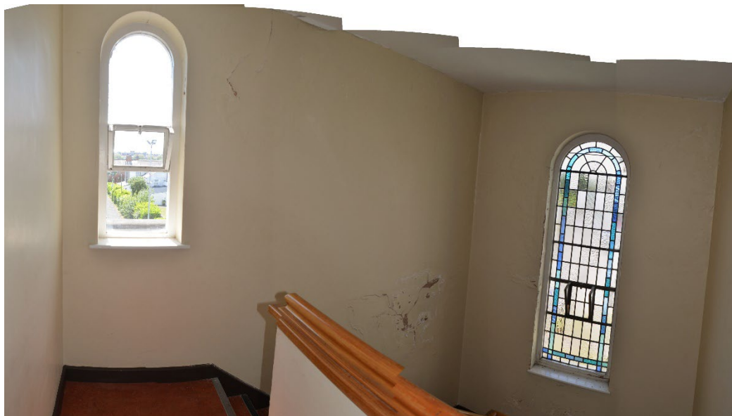
Figure 31: Front stair hall to the building.
