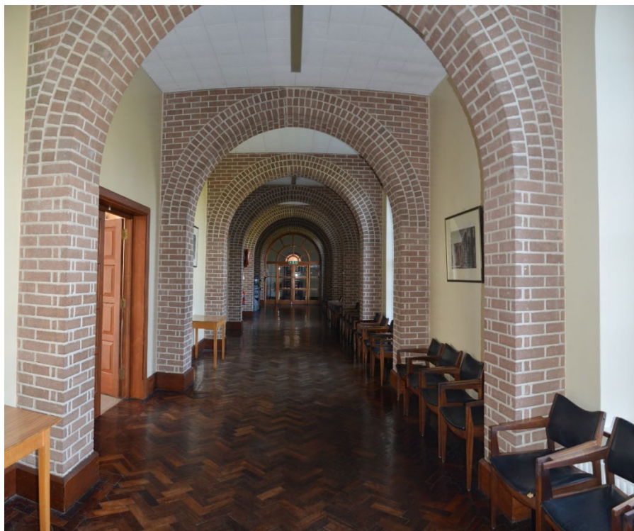
Figure 7: View of the late 20th century brick 'arches' at Ground Floor Level of the Main Seminary Block. The floors above and below are constructed in and supported by a steel and concrete frame. The brick visible here is a cladding which conceals the 1960s RSJs that intruded into Bourke's original corridor space. These represent 1960s cladding and support no loads above.
