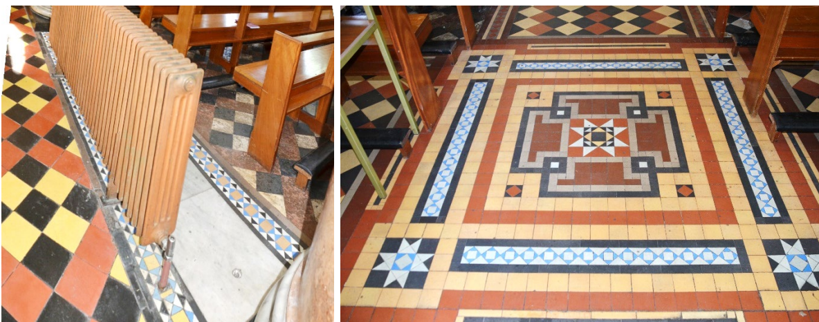
Figure 15: Photographs showing the encaustic tile flooring.
