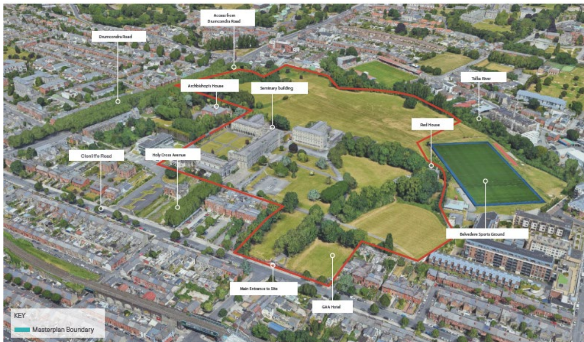
Figure 3: Aerial photo of overall site indicating relevant structures and red line of the subject site.
