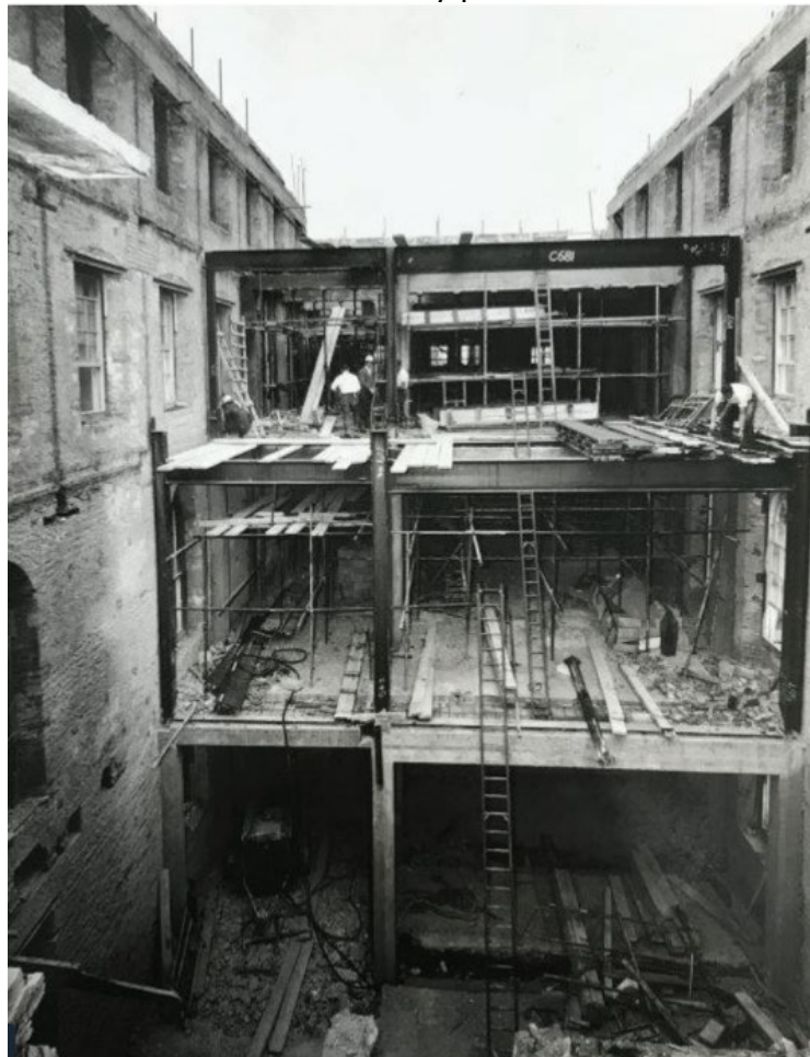
Figure 60: Photograph showing the complete internal reconstruction of the Main Seminary Block in 1966. Note the new concrete frame at the base and the RSJs which abut the walls and ultimately require cladding in brick slips.
