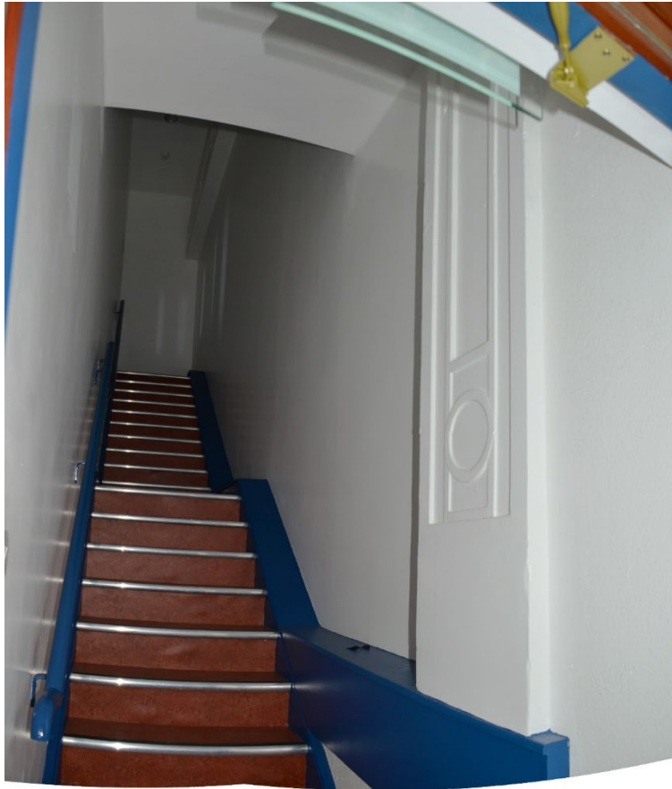
Figure 29: Internal photograph of the modern stairhall showing a surviving section of the original proscenium arch.
