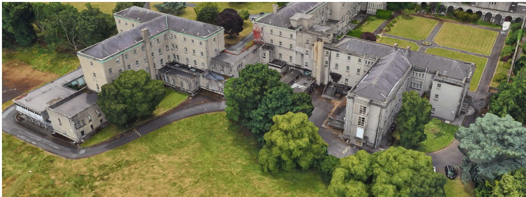
Fig. 66 Aerial view showing the much-later, mid-20 th Century, poorly executed 'pastiche' additions to the site known as the Library and New Wing.
