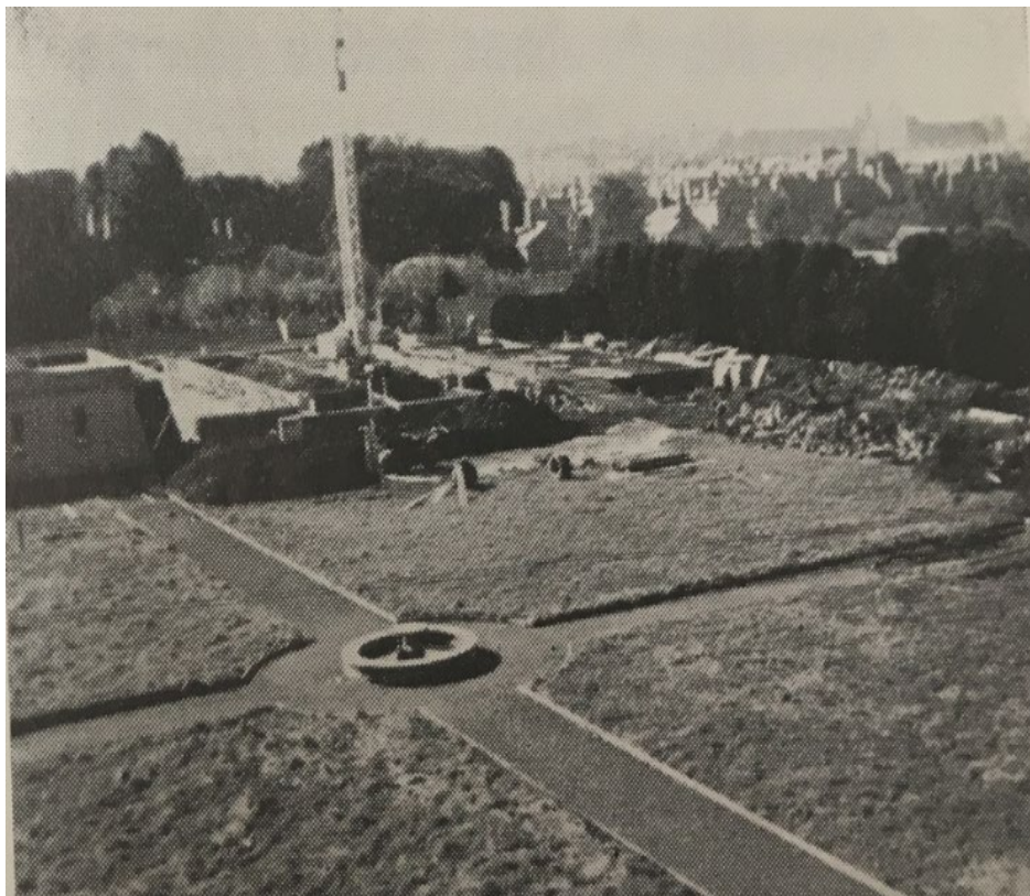
Figure 26: Photograph showing the construction of the new Assembly Hall to the south of the formal quadrangle to the rear of the Main College building and Holy Cross Church.
