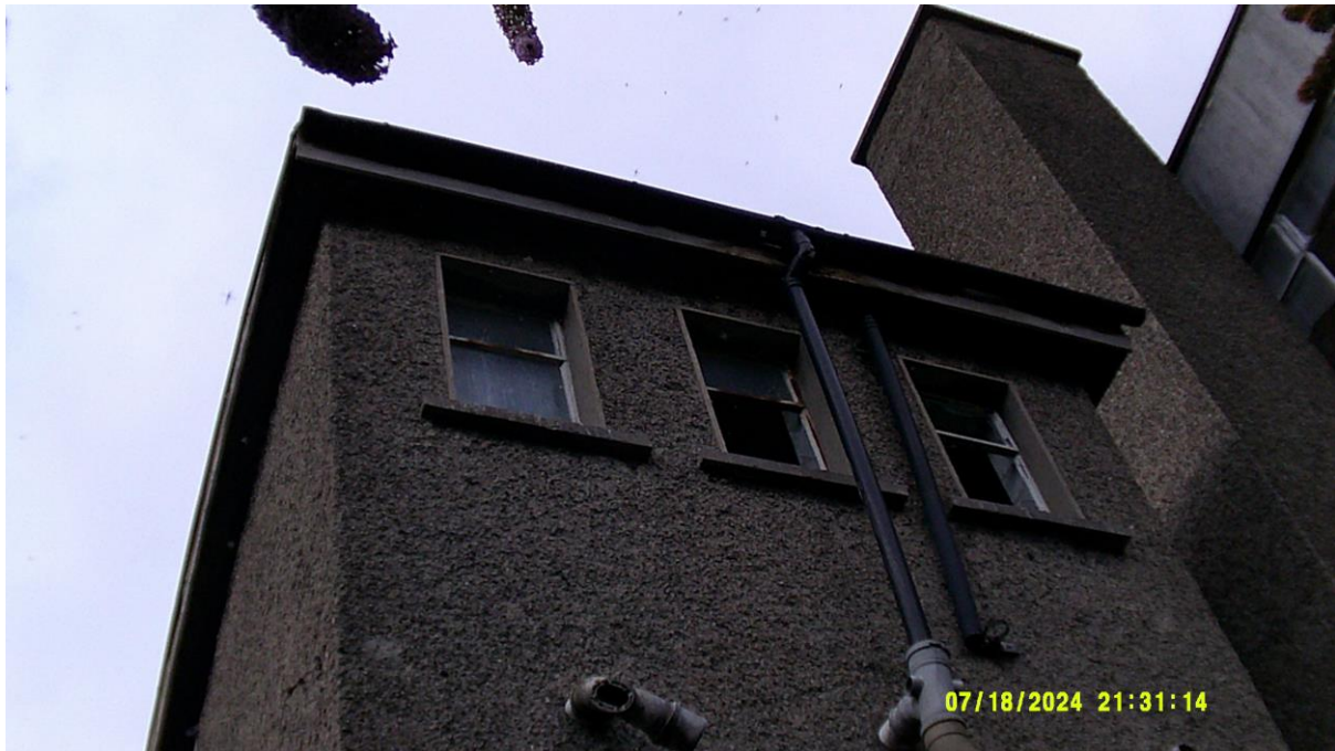
FIGURE 4. PRF 1 – TOWER STRUCTURE.
