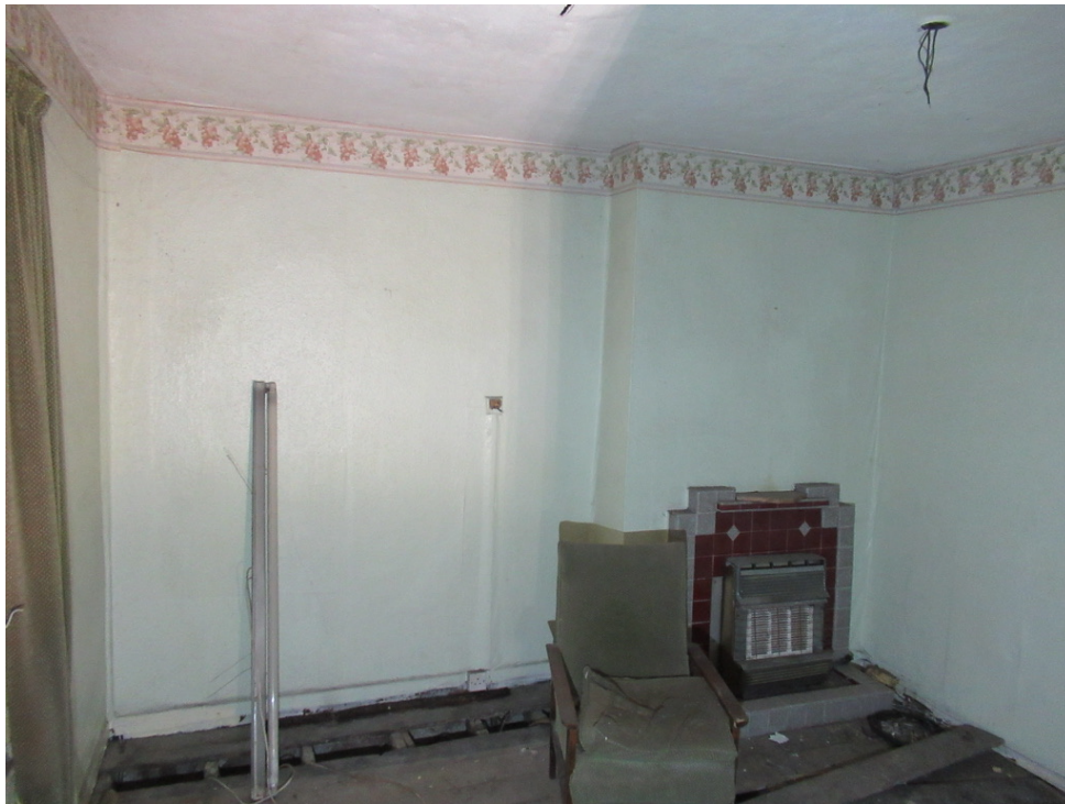
Plate No. 90. General internal view the first floor bedroom in No. 48 Dolphins Barn Street, as it appeared in 2017. The tiled fireplace dates from the middle of the 20 th century. (Photo by Stephen Farrell, 2017)
