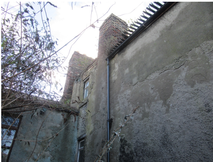
Plate No. 73. General view showing the north party wall elevation to No. 47 Dolphins Barn Street as it appeared in 2017. The space between the chimney stacks would have contained the stairwell inside the original house. Corner chimney breasts remain in all of the original principal rooms. (Photo by Stephen Farrell, 2017)
