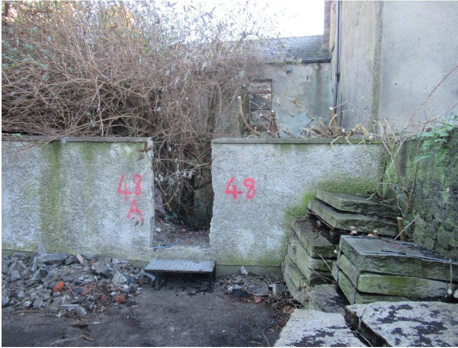
Plate No. 87. General view showing the rear elevation to No. 48 Dolphins Barn Street as it appeared in 2025. (Photo by the author, 2025)
