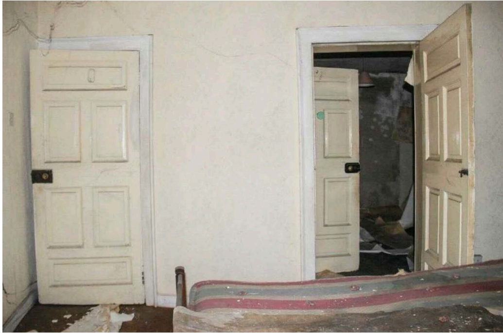
Plate No. 39. General view showing the 18th century paneled timber doors in the first floor in No. 44. These doors appear to date from around 1740-1760, and were left in place when the house was refurbished and updated around 1825. (Photo by Stephen Farrell, 2017)
