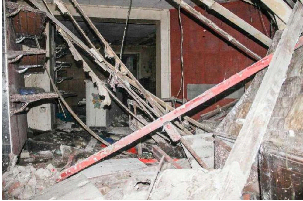
Plate No. 65. General view showing the ground floor shop in No. 46 Dolphins Barn Street as it appeared in 2017. This view shows that the large angled chimney breasts remain in place on the ground floor, and probably also in the floors above. Otherwise, nothing remains of the 18th century building fabric. This structure is now too dangerous to enter, other than the entry hall. (Photo by Stephen Farrell, 2017)
