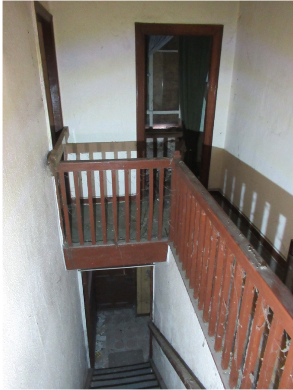
Plate No. 89. General internal view showing the plain mid-20 th century stairs and railing at the first floor landing in No. 48 Dolphins Barn Street, as it appeared in 2017. (Photo by Stephen Farrell, 2017)
