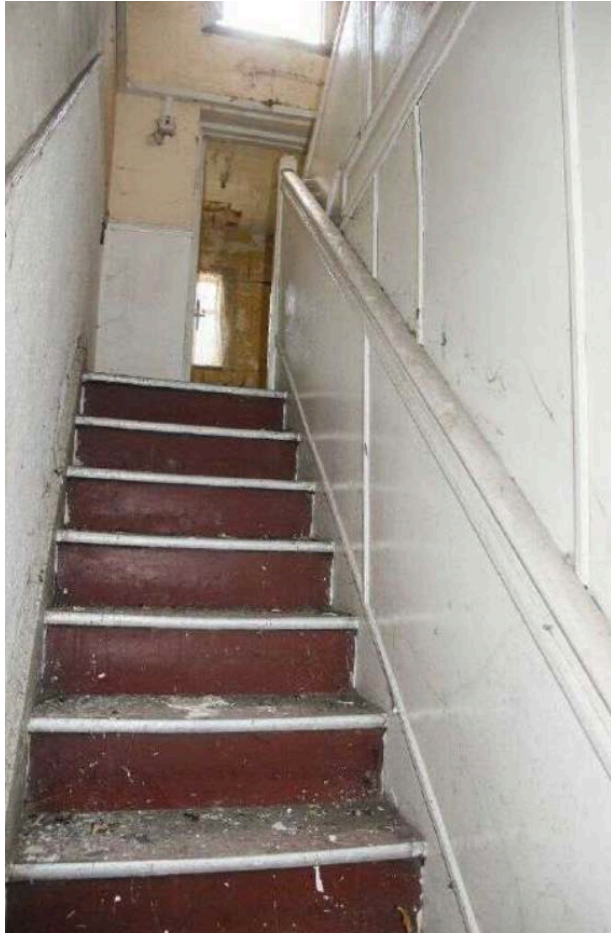
Plate No. 97. General view showing the rear stairs in No. 49 Dolphins Barn Street, as it appeared in 2017. (Photo by Stephen Farrell, 2017)
