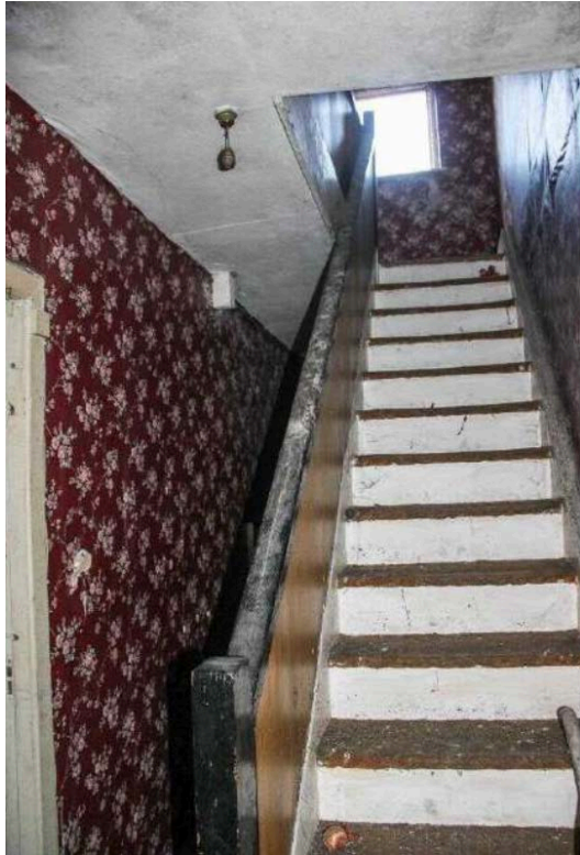
Plate No. 76. General view showing the timber stairs running from the first floor to the second floor, in the rear of No. 47 Dolphins Barn Street as it appeared in 2017. This stair dates from the second half of the 20 th century, and corresponds to the time when the entire interior of the house was stripped out and rebuilt. (Photo by Stephen Farrell, 2017)
