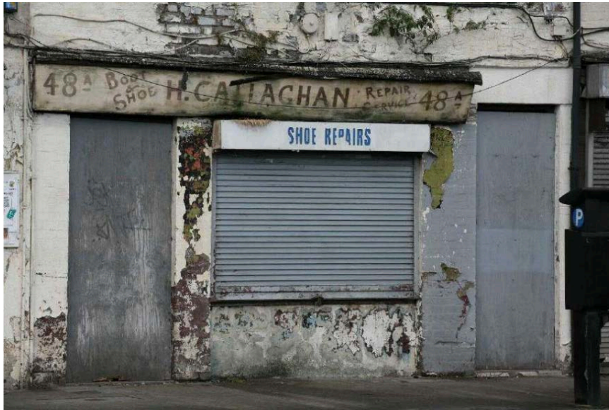
Plate No. 85. Detail view showing the ground floor shopfront to No. 48 Dolphins Barn Street as it appeared in 2017. The door to the left enters the shop and the door to the right enters the stairwell. (Photo by Stephen Farrell, 2017)
