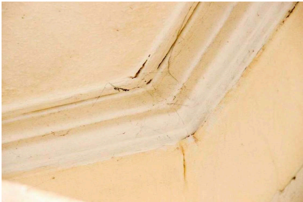
Plate No. 34. Detail view showing the early 19th century plaster coving in the ground floor rear room at No. 44 Dolphins Barn Street, as it appeared in 2017. (Photo by Stephen Farrell, 2017)
