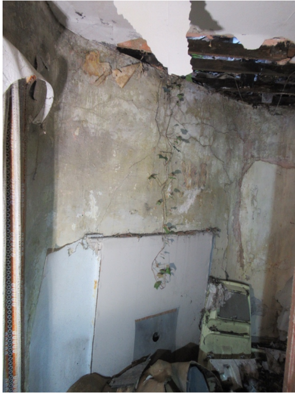
Plate No. 91. General view showing the angled chimney breast in the first floor room over the late 19 th century laneway in No. 48 Dolphins Barn Street, as it appeared in 2017. (Photo by Stephen Farrell, 2017)
