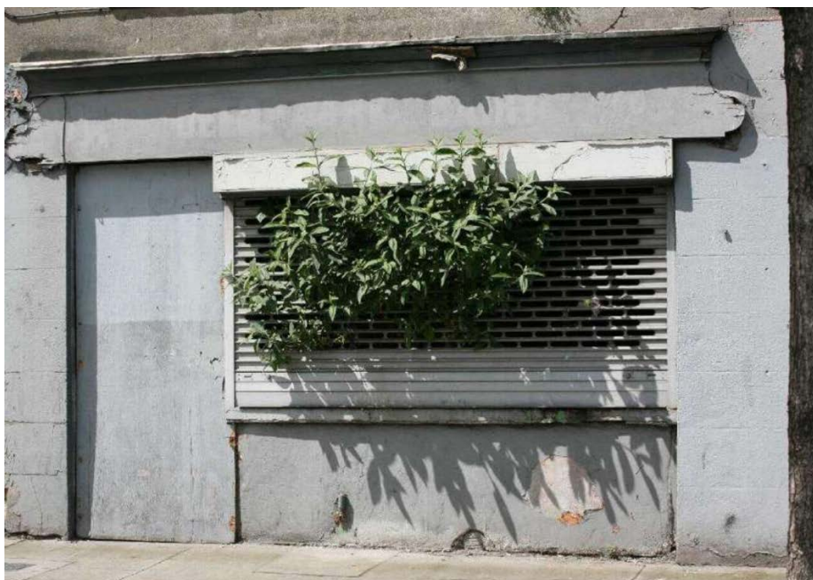
Plate No. 26. General view showing the front elevation to No. 44 Dolphins Barn Street. Note the early 20th century shopfront signboard, and the small shop window. (Photo by Stephen Farrell, 2017)
