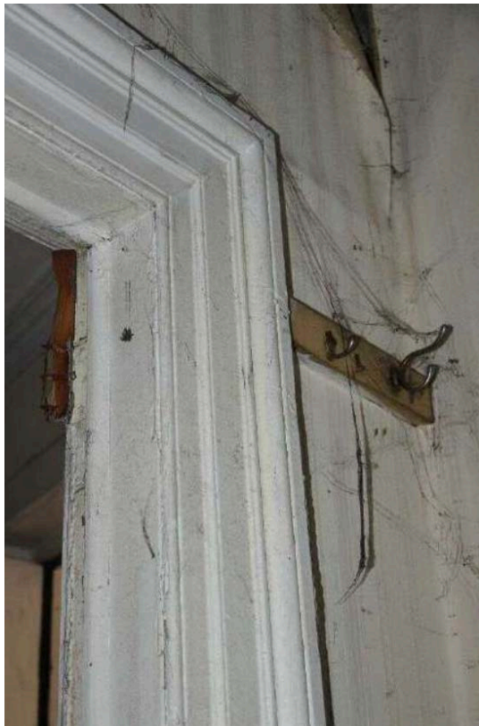
Plate No. 40. Detail view showing the early 19th century moulded timber door architrave seen in the ground and first floors in No. 44 Dolphins Barn Street as it appeared in 2017. These architraves likely date from the early 19th century. (Photo by Stephen Farrell, 2017)
