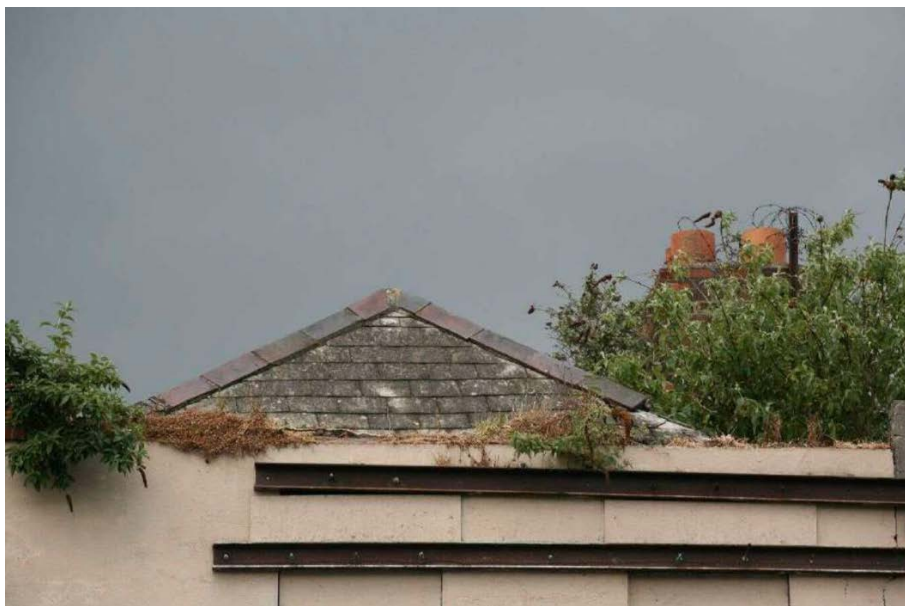
Plate No. 61. Detail view showing the hipped roof over No. 45 Dolphins Barn Street as it appeared in 2017. The shallow pitch of this roof strongly suggests that it is not the original 18th century roof, which would have been significantly steeper in pitch. (Photo by Stephen Farrell, 2017)
