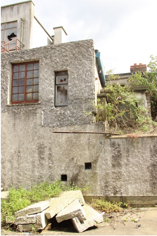
Plate No. 95. General view showing the rear elevation to No. 49 Dolphins Barn Street as it appeared in 2025. There are at least two periods of extensions to the rear of this property, likely dating from the middle of the 20 th century.
