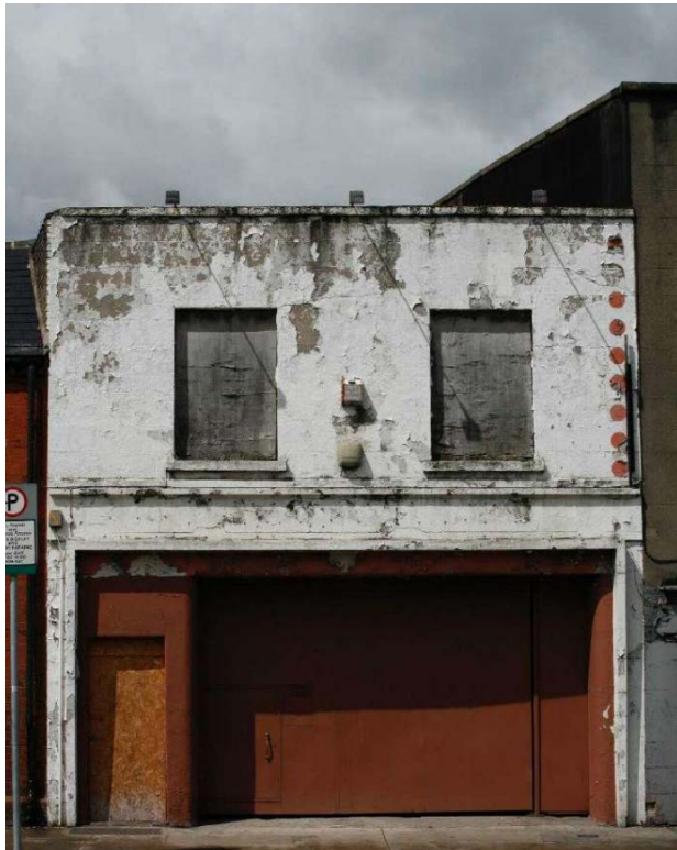
Plate No. 14. Front elevation to No. 43 Dolphins Barn Street, showing the entrance door at left, and the vehicular lane through to the rear site, taking up the rest of the front elevation. (Photo by Stephen Farrell, 2017)
