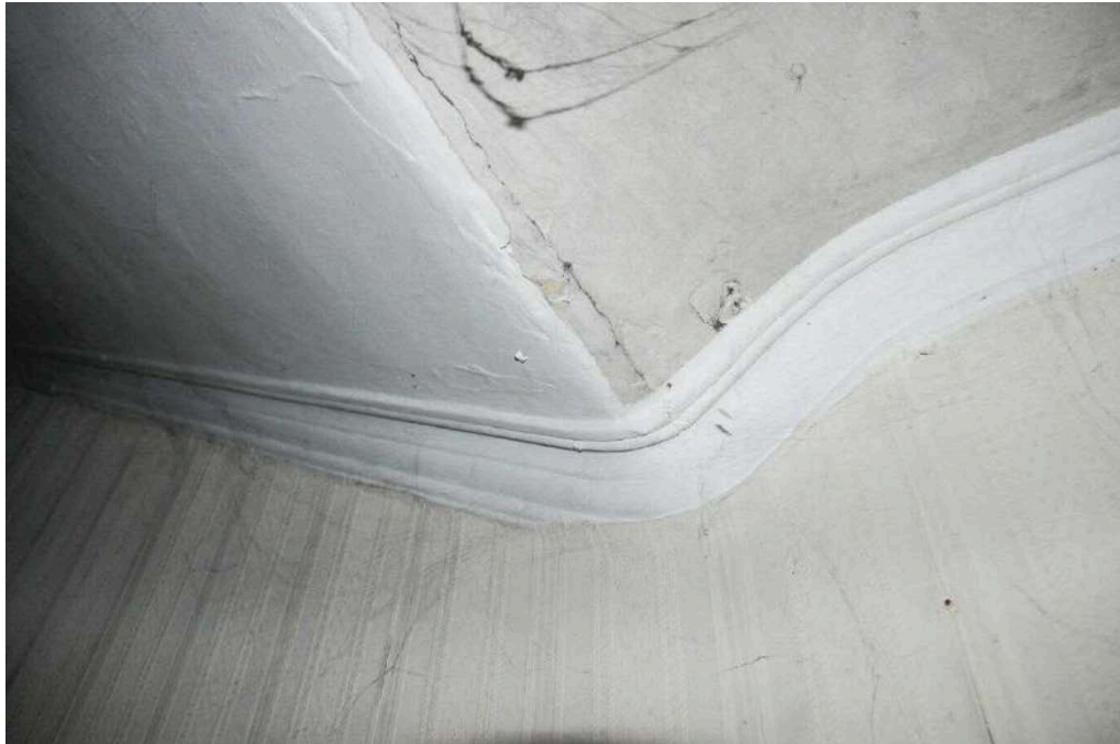
Plate No. 35. Detail view showing the early 19th century plaster coving to the stairwell in No. 44 Dolphins Barn Street as it appeared in 2017. That area has since been heavily damaged by damp rot and dry rot fungus. (Photo by Stephen Farrell, 2017)
