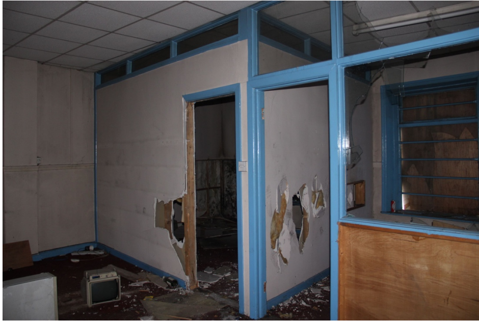
Plate No. 21. General view showing the appearance of the first floor in No. 43, as it appeared in 2017. There are no early chimney breasts on the party wall, and no trace of any internal building fabric earlier than the mid to late 20 th century. (Photo by Stephen Farrell, 2017)
