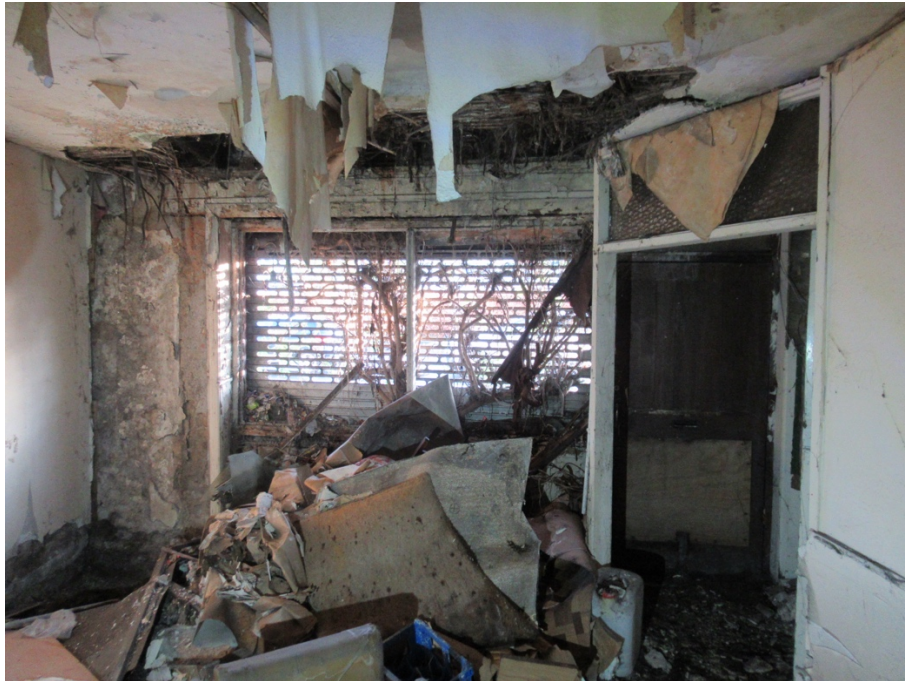
Plate No. 29. General view showing the front elevation to No. 44 Dolphins Barn Street. Note the flat roof, early 20th century shopfront signboard, and sand and cement render. (Photo by the author, 2025)
