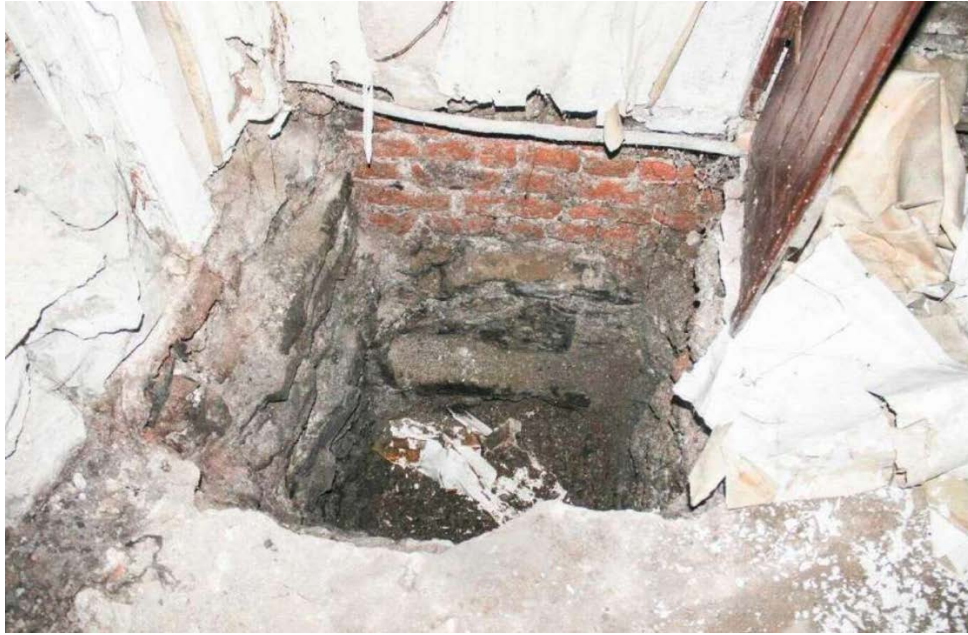
Plate No. 33. Detail view showing the test hole in the ground floor slab to No. 44 Dolphins Barn Street. This excavate reveals that foundation consists of handmade red brick on a rubble stone foundation. (Photo by Stephen Farrell, 2017)
