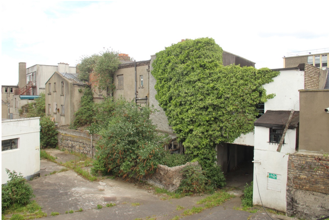
Plate No. 18. View showing the rear elevations and rear site to the group of former houses. The vehicular lane through No. 43 is at the right. (Photo by Stephen Farrell, 2017)
