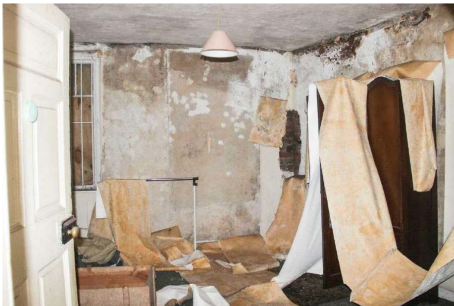
Plate No. 42. General view showing the rear first floor room in No. 44 Dolphins Barn Street as it appeared in 2017. That area has since been more heavily damaged by damp rot and dry rot fungus. There is an angled corner chimney breast at the right, out of the view. (Photo by Stephen Farrell, 2017)
