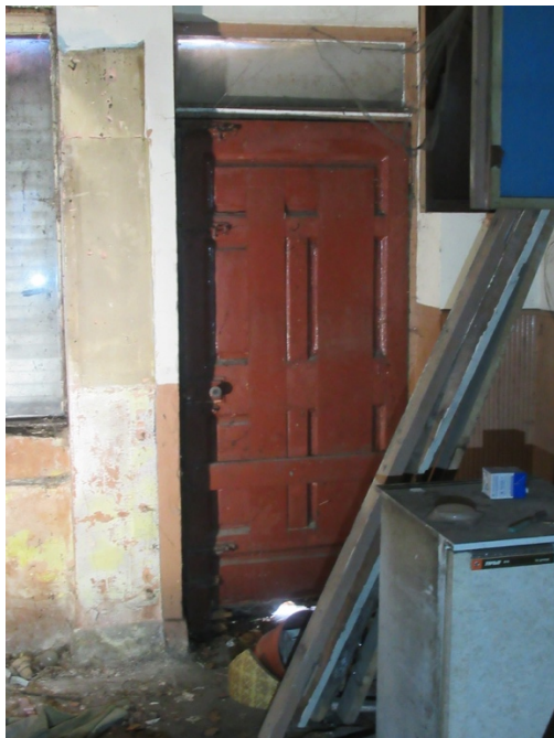
Plate No. 86. General view showing the rear elevation to No. 48 Dolphins Barn Street as it appeared in 2017. This door is older than the structure that is currently in place. It could have been re-used when the earlier house was rebuilt, or it could have been salvaged from another site when the shopfront was installed or renovated during the 20 th century. (Photo by Stephen Farrell, 2017)
