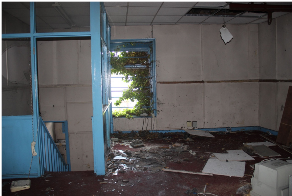
Plate No. 22. General view showing the rear half of the first floor in No. 43, as it appeared in 2017. (Photo by Stephen Farrell, 2017)
