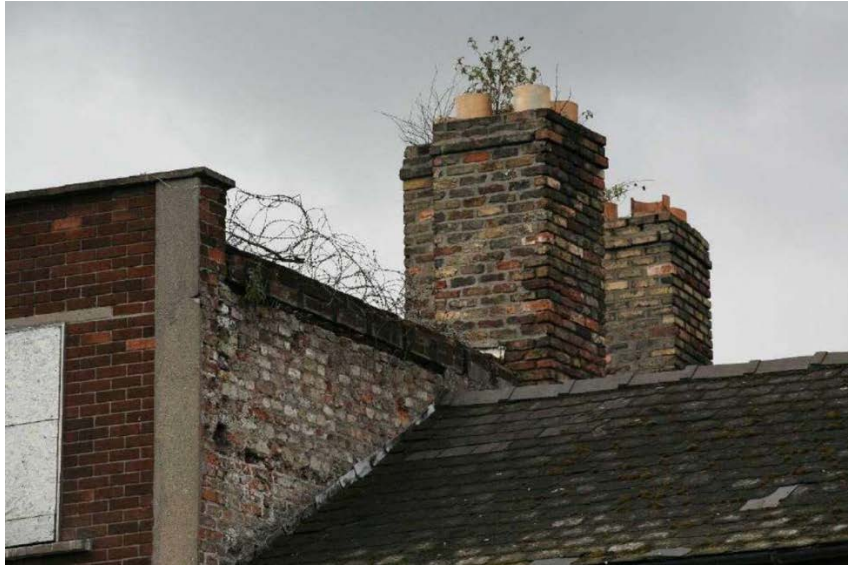
Plate No. 72. General view showing the north party wall and the two massive chimney stacks that served the corner fireplaces in No. 47 Dolphins Barn Street. (Photo by Stephen Farrell, 2017)
