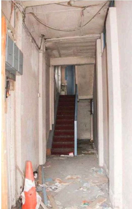
Plate No. 19. View showing the ground floor entry hall, looking towards the stairwell. (Photo by Stephen Farrell, 2017)
