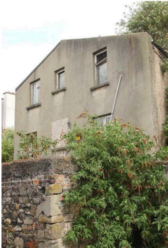
Plate No. 74. General view showing the rear elevation to No. 47 Dolphins Barn Street as it appeared in 2017. The shallow pitch of the rear half of the roof shows that the original gabled roof was replaced, probably around 1960. It is unclear how much of the rear elevation was also replaced. (Photo by Stephen Farrell, 2017)
