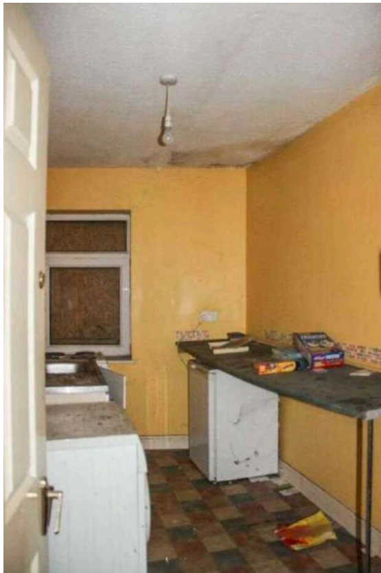
Plate No. 59. General view showing the second floor front kitchen room in No. 45 Dolphins Barn Street as it appeared in 2017. There is no trace of the 18th century wall or ceiling plaster, or any historic joinery in this structure. (Photo by Stephen Farrell, 2017)
