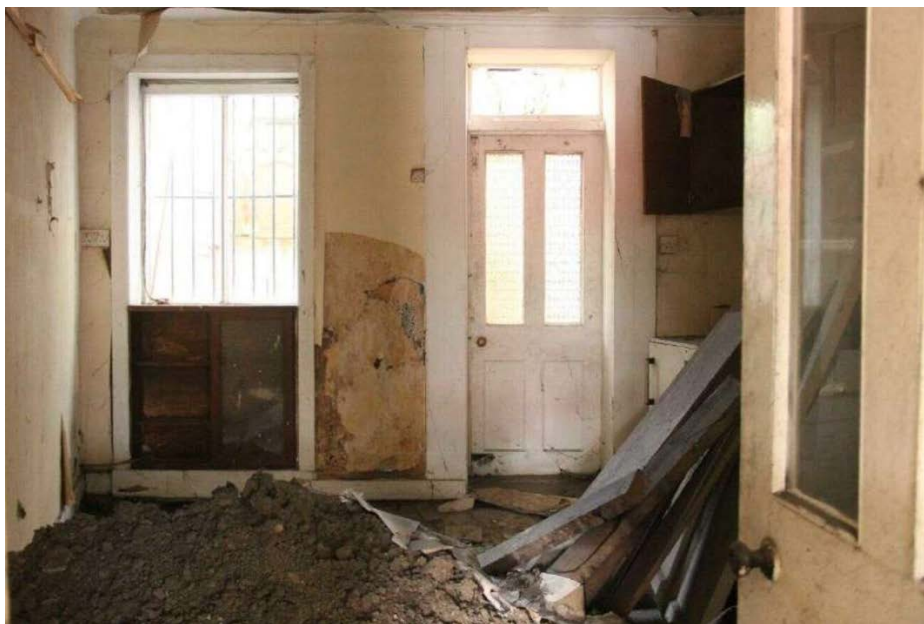
Plate No. 30. General view looking to the rear, showing the rear room in the ground floor to No. 44 Dolphins Barn Street. The pile of clay was from an archaeological test pit. (Photo by Stephen Farrell, 2017)
