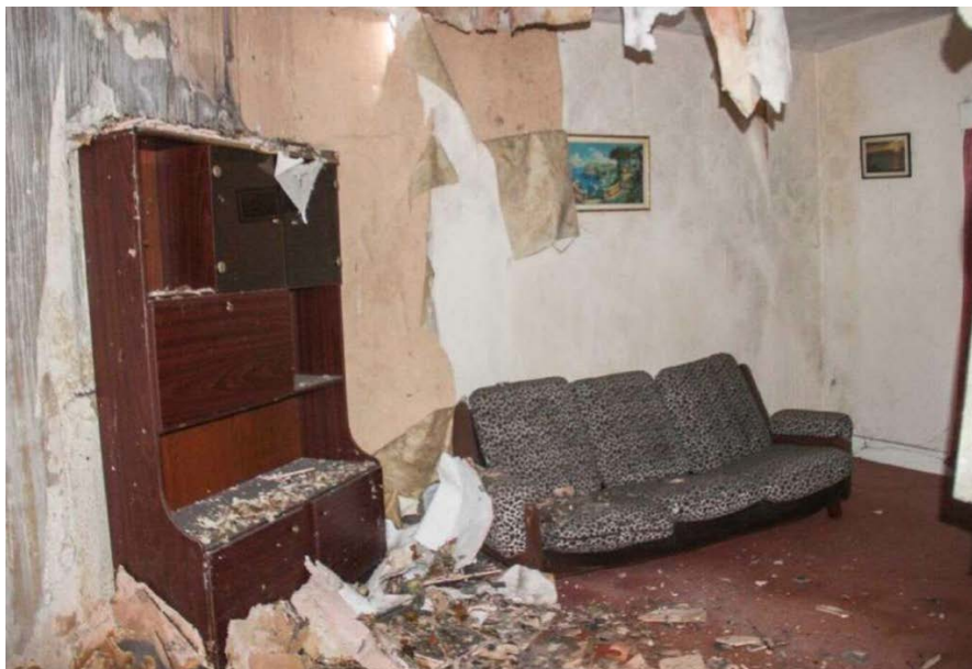
Plate No. 98. General view showing the angled chimney breast in the first floor front room in No. 49 Dolphins Barn Street, as it appeared in 2017. It is possible that some of the basic structure to No. 49 has survived from the original 18 th century structure, including this chimney breast. (Photo by Stephen Farrell, 2017)
