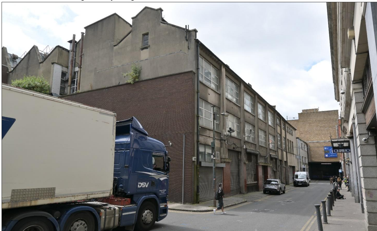
Photo 3: A view west along the site frontage to Prince's Street North
