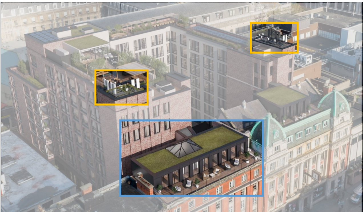
Figure 1a: Aerial view of the Stage 2 proposal showing the rooftop telecommunications infrastructure and a vertical extension to Emerald Chambers
