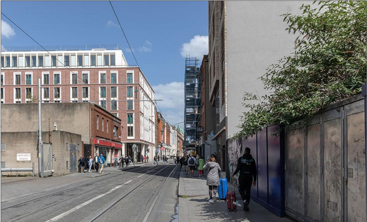
Photo 20: The Motel One hotel at the corner of Abbey Street and Liffey Street Upper
