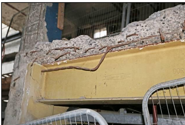
RFC and steel deck detailing on mezzanine floor.
