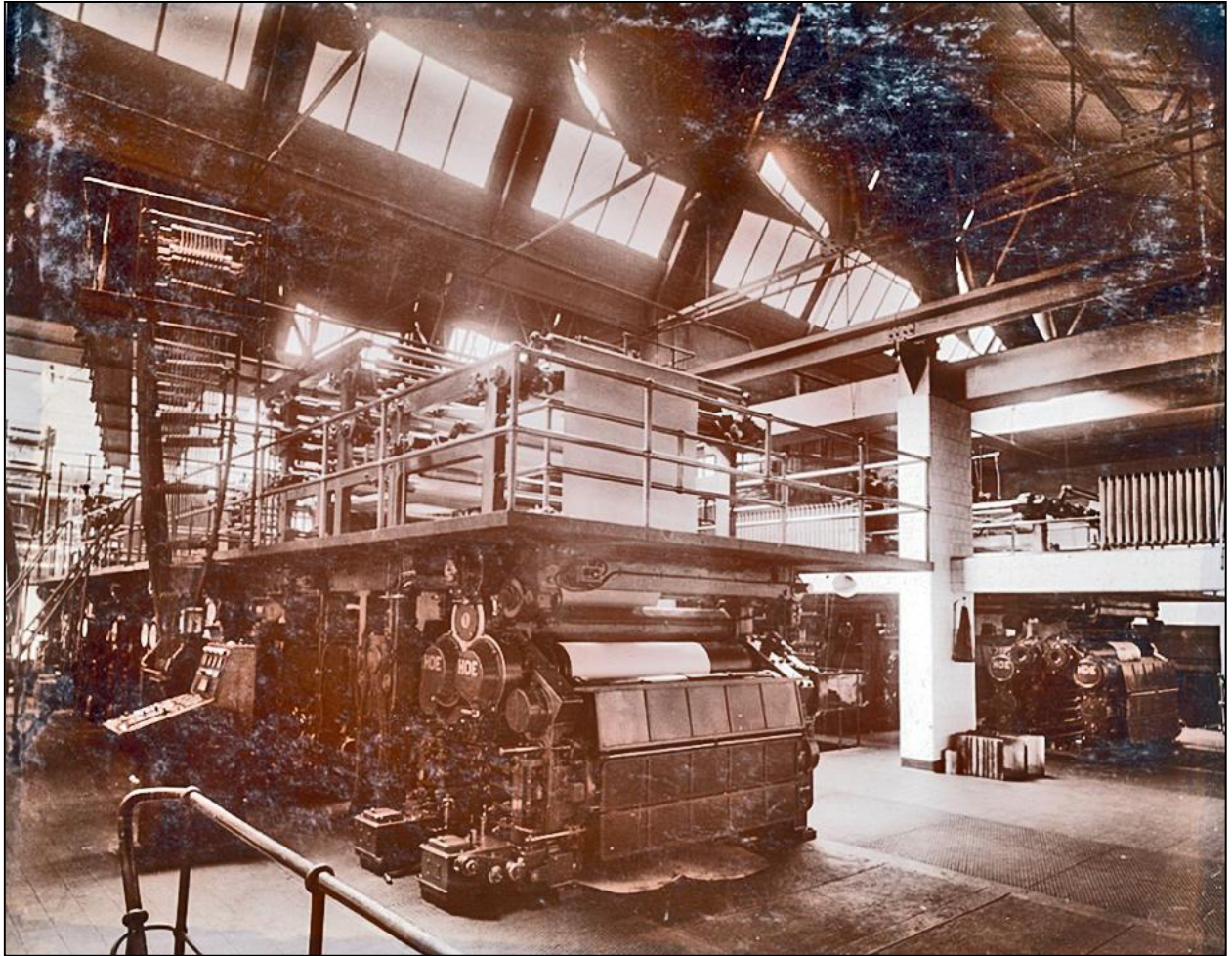
Fig 1.17 Circa 1938 view of the enlarged Machine Hall, as viewed from the SW corner of the ground floor of its west bay. The handrail around the stairs to the basement is visible at bottom left. The massive presses run the length of the hall and rise up to the saw-tooth roof, the windows of which face north to reduce glare. The press on the right is in the 1924 bay and the one at left is in the new extension. 'Hoe', their manufacturer, is evident on the gear covers along the sides of both machines. Note also the skeletal reinforced-concrete column-and-beam frame between the two bays and the central heading radiators on the beam between the ground and first floor levels. Overhead travelling cranes served the presses, the rails of which are visible just below the roof valleys ( University College Dublin: Photographic Archive, item 243 ).
