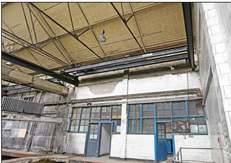
Above: Cranes in east bay (arrowed in red), from NE corner of the basement. The back one could lift 1½ tons (1524kg).
