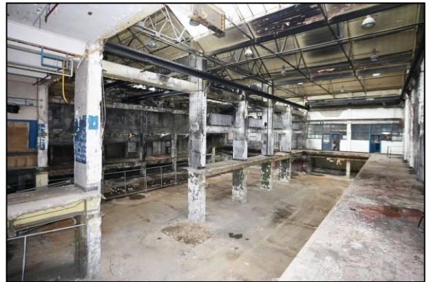
Looking SE from NW corner of mezzanine floor.
