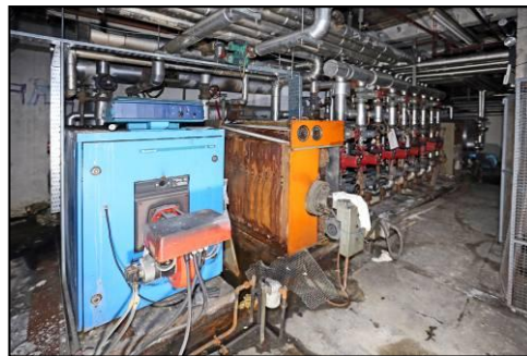
Left: Firedoor at entrance to boiler room.
