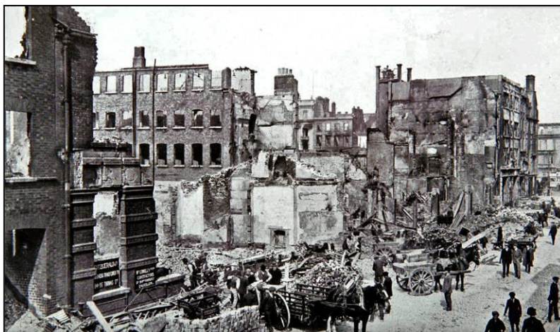
Looking east along Middle Abbey St. The entry to William's Lane and the burnt-out shell of Messrs Fitzgerald are at extreme left ( The Sinn Féin Rebellion, Belfast 1916 ).
