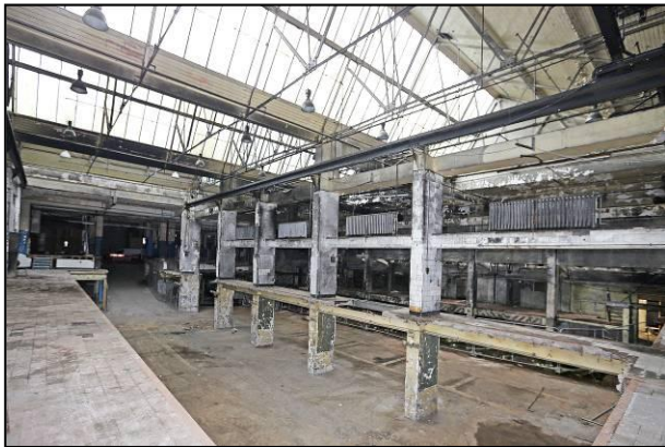
Looking NE from SW corner of mezzanine floor.
