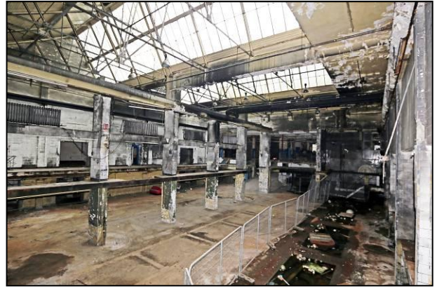
Looking NW from SE corner of mezzanine floor.
