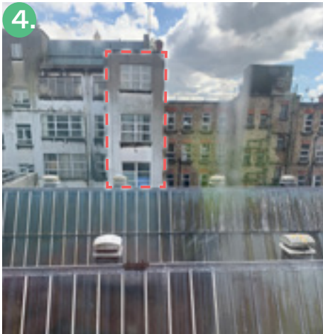
Non-original upper levels / vertical extension of rear return of Independent House removed
