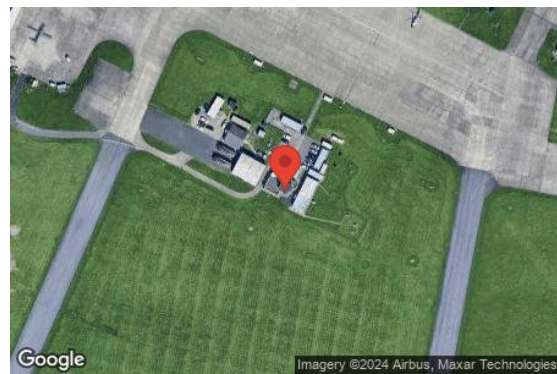
Figure 27. 8-ATCT Baldonnel ATCT
