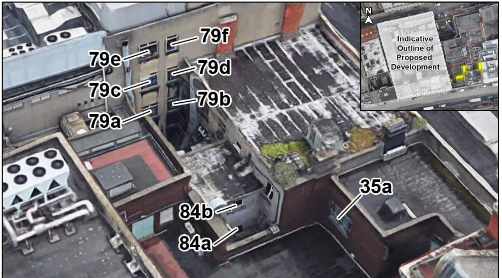
Fig. 5.7: Indication of the position of assessed windows (T), Aerial view of assessed location (B)
