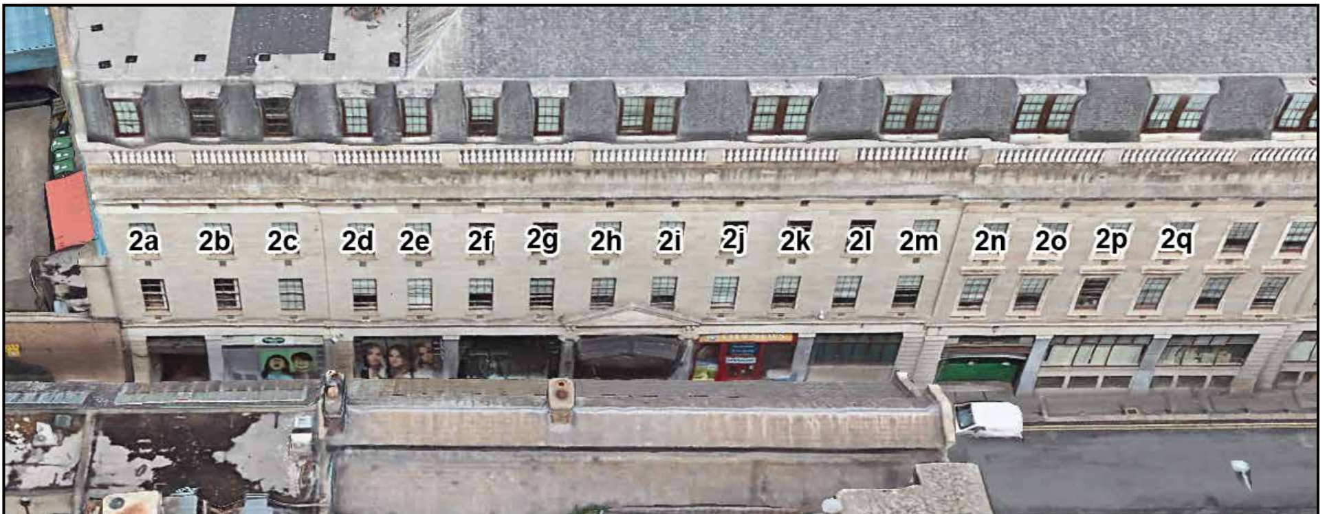
Fig. A.17: Indication of the position of assessed windows (T), Aerial view of assessed location (B)
