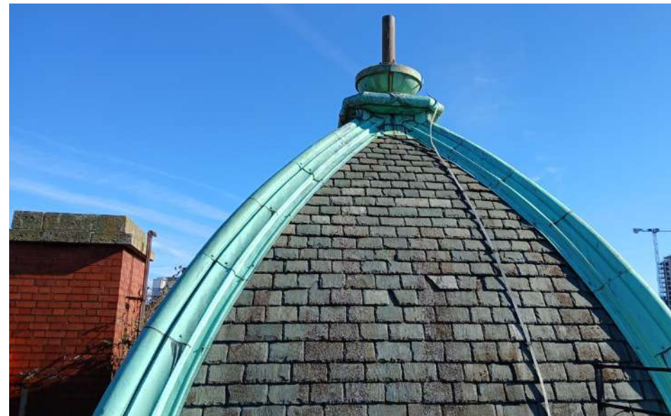
Plate 26: Natural slates laid in diminishing courses, with copper panel cladding the ribs. Integrated base for flagpole.
