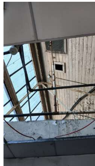
Plate 86: Underside of pitched roof above Independent House, Lightweight steel truss, timber boarding with slate lining externally, patent glazing system to north pitch.
