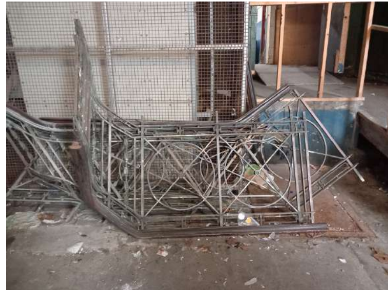
Plate 238: Salvaged stair / ramp balustrade with timber handrail stored within Zone 4. Original position was possibly within this service zone of the main stairs in Independent House.
