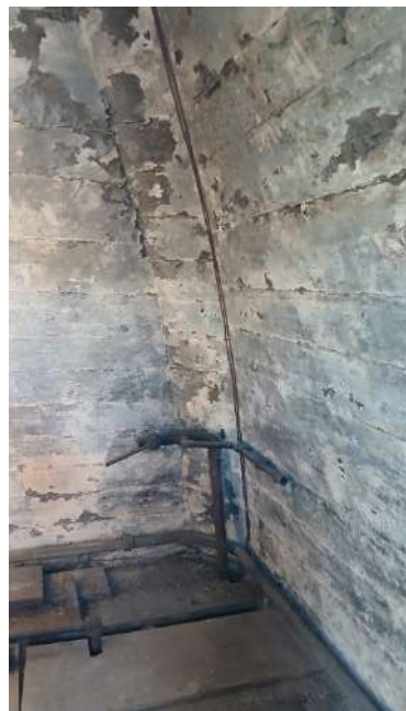
Plate 31: The structure of the domes is revealed internally as comprising board-marked concrete shell with cross vault ribs.
