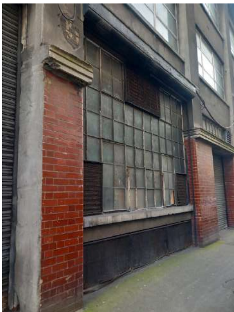
Plate 220: Multi-pane metal window frames with inset louvred vents and grilles at street level.
