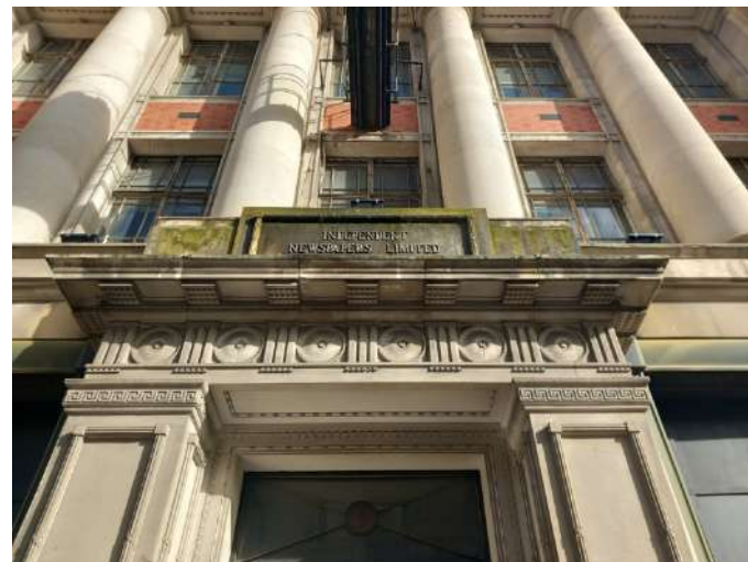
Plate 8: Framed panel and brass lettering stating 'Independent Newspapers Limited' above entablature.
