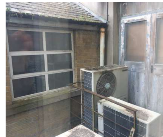
Plate 172: View of Williams Lane facing south towards Middle Abbey Street. West elevation of Zone 5 (left), forming the eastern boundary of Williams Lane. Stock brick wall finish, laid in English garden wall bond. The northern end of Williams Lane is covered with a smooth cement render.
