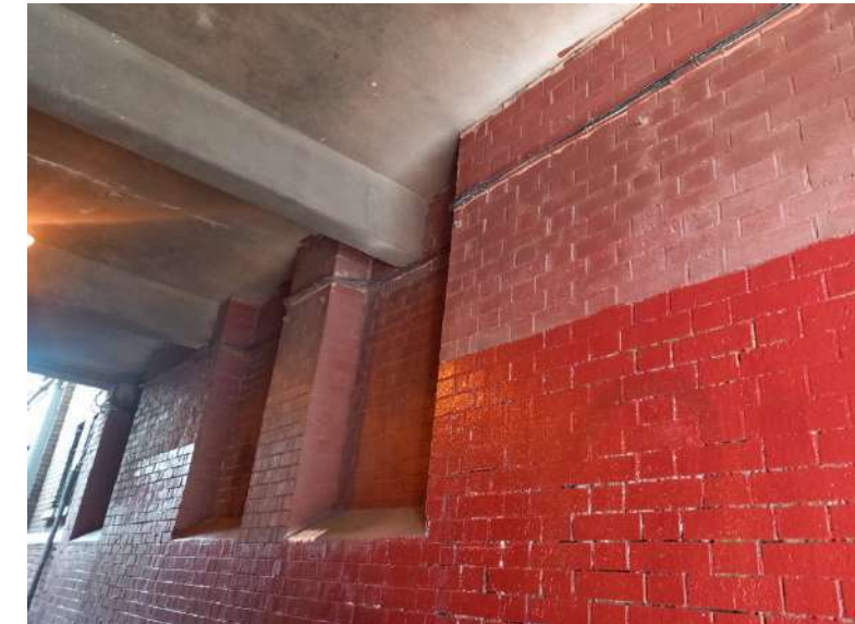
Plate 105: Blind windows on the western boundary wall of 87-90 Middle Abbey Street. The concrete soffit of Abbey Chambers 94-96 Middle Abbey Street is integrated into the brick boundary wall.
