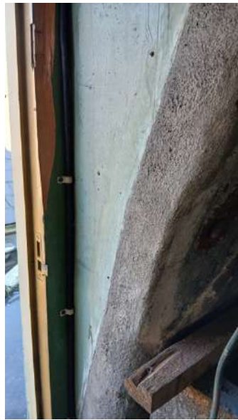
Plate 28: The dome structure is comprised of a thin concrete shell.
