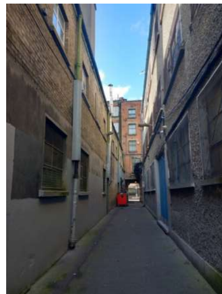
Plate 107: William's Lane facing south towards Middle Abbey Street. Abbey Chambers 94-96 Middle Abbey Street extends over the lane. Building F of the rear building range is aligned with William's Lane. The external wall is comprised of brick, with cement render applied to localised areas.
