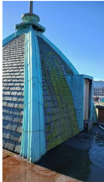
Plate 22: West dome on main roof contains original and later water tank. Access via a door on the northern face.
