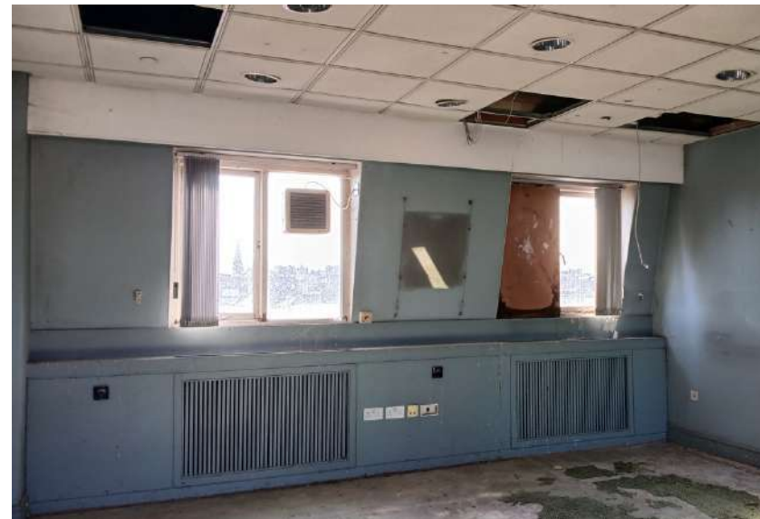
Plate 94: Replacement timber windows at fourth floor level. Contemporary wall linings.
