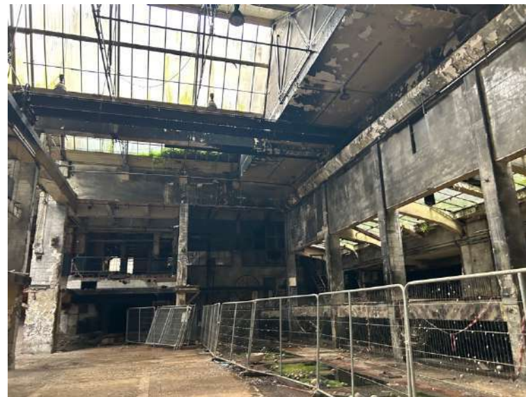
Plate 188: View facing north. Masonry columns clad in white (discoloured) glazed tile. Area to the east of the hall was inaccessible due to safety concerns. Historic maps suggest that this eastern side of the hall was constructed c1924, and subsequently extended post the acquisition of the adjoining site in 1936.
