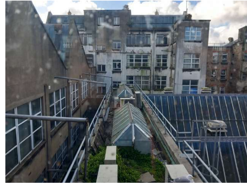
Plate 20: Rear façade of Independent House. The projecting bay to the west (right) is a later extension to what was originally a single storey return.
