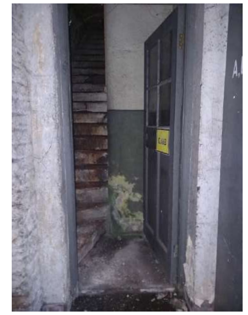
Plate 198: Granite stairs within bottom winder step in southwest corner at upper ground level, attached to the rear of 87-90 Middle Abbey Street. Door with two lower solid panels and glazed upper panels.
