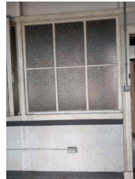
Plate 65: Typical glazed screen on upper level of internal partitions.
