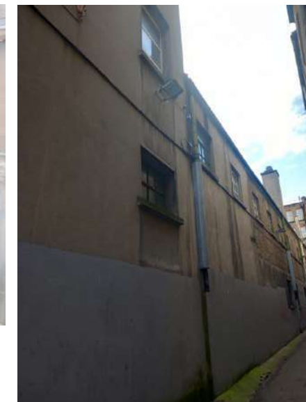
Plate 177: West elevation of Zone 5, forming the eastern boundary of Williams Lane. Stock brick wall finish, with areas of cement render.
