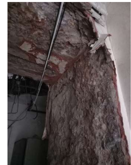
Plate 144: Opening through the party wall between 91-92 and 87-90 Middle Abbey Street (Independent House) is crudely formed through concrete structure.
