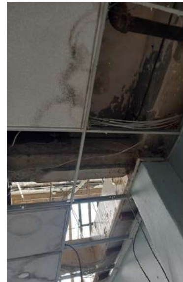
Plate 90: Contemporary ceiling on top floor, concealing original sawtooth rooflights over.
