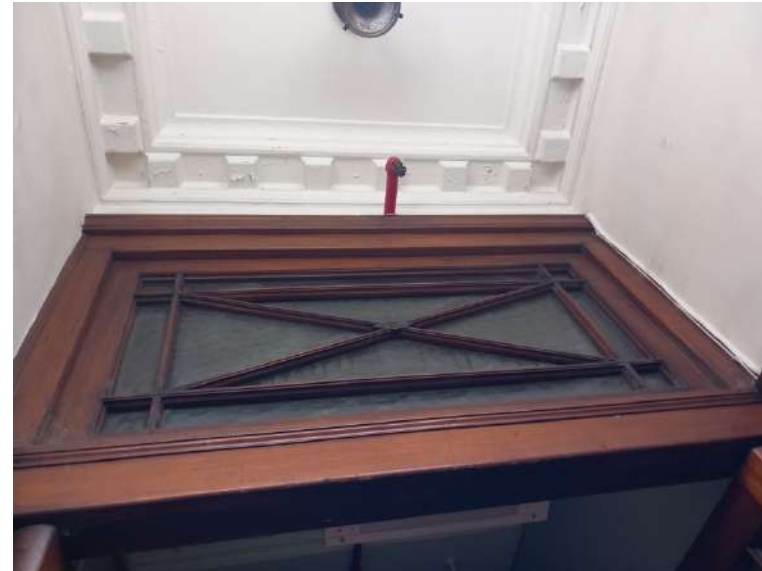
Plate 130: Timber frame transom light above internal lobby door with margin lights and cross bracing.
