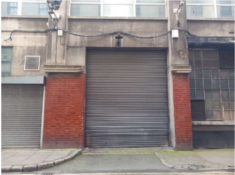
Plate 215: Granite kerbs (dropped on western side) leading to former vehicular entrance. This stepped cornice originally spanned across the full width of the opening, with a multipaned window over, but the
