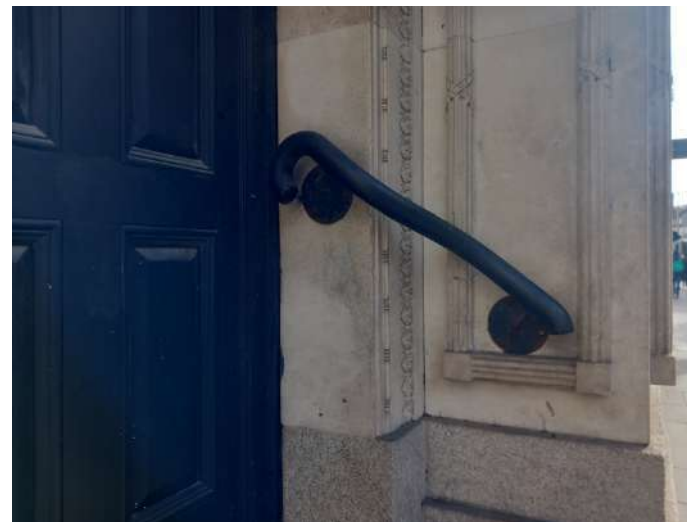
Plate 9: Handrail at entrance door fixed to Portland stone reveals.
