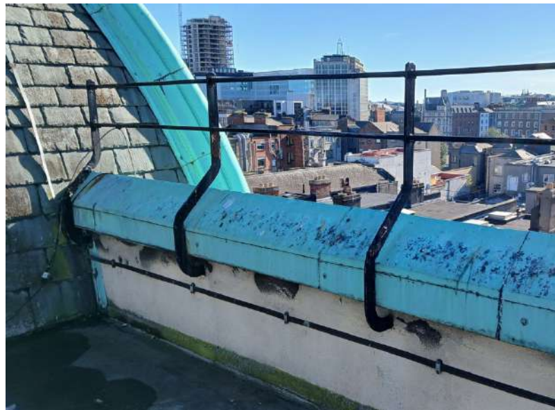
Plate 25: Copper panelling to front parapet with industrial style railings fixed to the masonry upstand.
