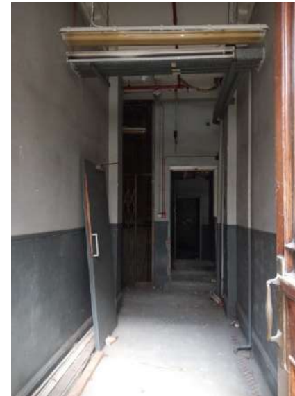
Plate 131: Entrance Hall, original mosaic floor with contrast colour boarder, original moulded timber skirting, rendered walls with inset dado, modillion cornice. Surface mounted contemporary services throughout.
