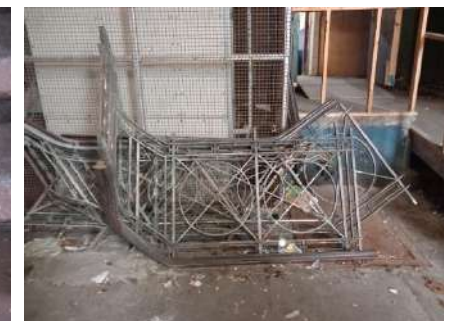
Plate 5 Original balustrade, previously installed on ground to first floor levels. Presently located in Zone 4b.
