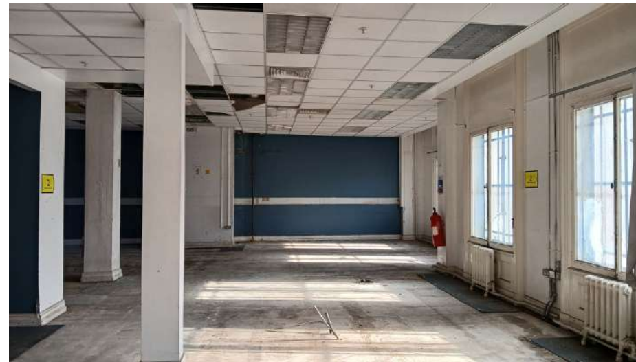
Plate 54: Level 2 has been extensively modernised to create an open plan office space. Contemporary wall linings and suspended ceiling. Original window fabric.
