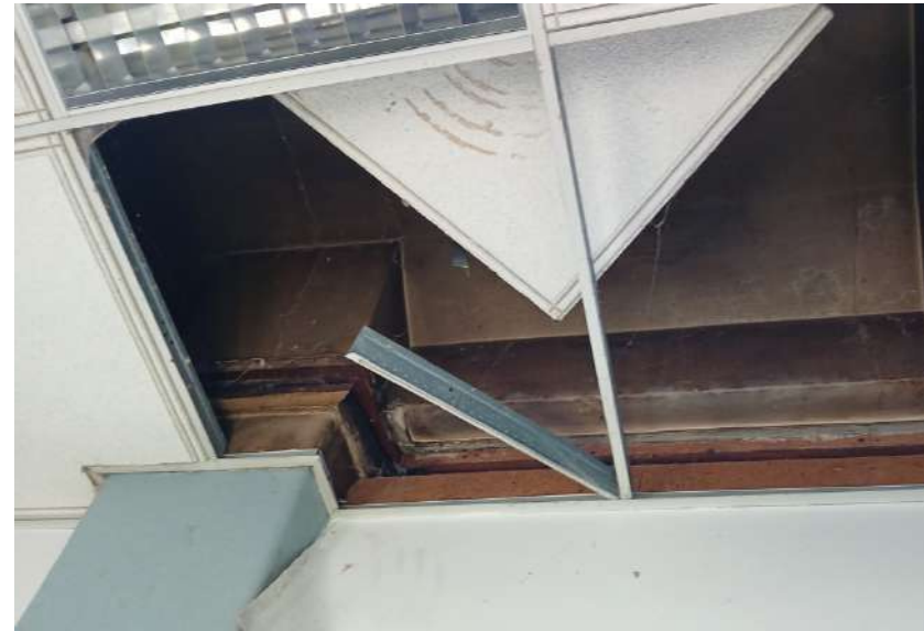
Plate 91: Original concrete roof structure above contemporary suspended ceiling.
