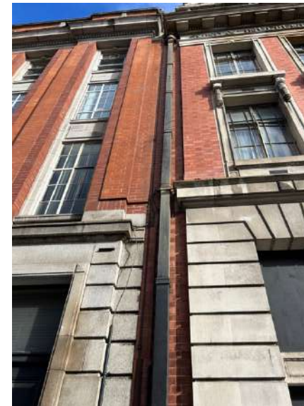
Plate 115: Rectangular profile cast iron downpipe between No 91-93 and Independent House.
