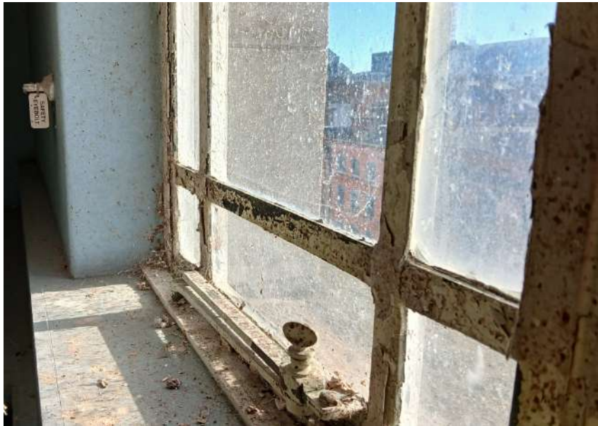
Plate 96: Detail of original metal casement window with margin lights.
