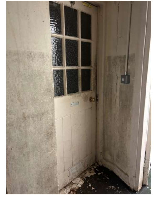
Plate 255: Example of original door within Zone 4. 2 panel door with vertical boarding to lower panel and multipaned glazing to upper panel.
