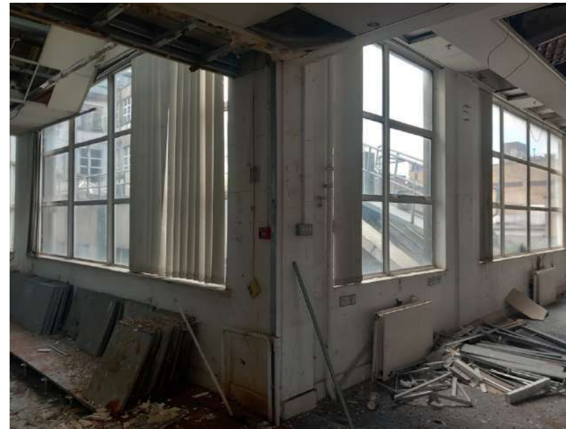
Plate 273: View facing south-west. uPVC windows, raised access floor, contemporary lay-in ceiling tiles. Former open plan office space.
