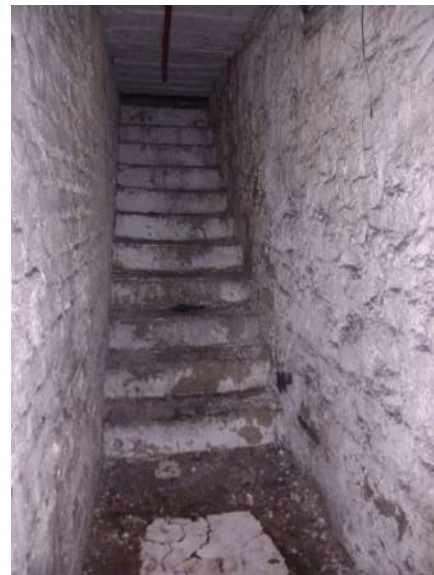
Plate 123: Granite stair from basement level, behind main central stair is aligned with rear Calp limestone basement wall. Access is obstructed at ground level.
