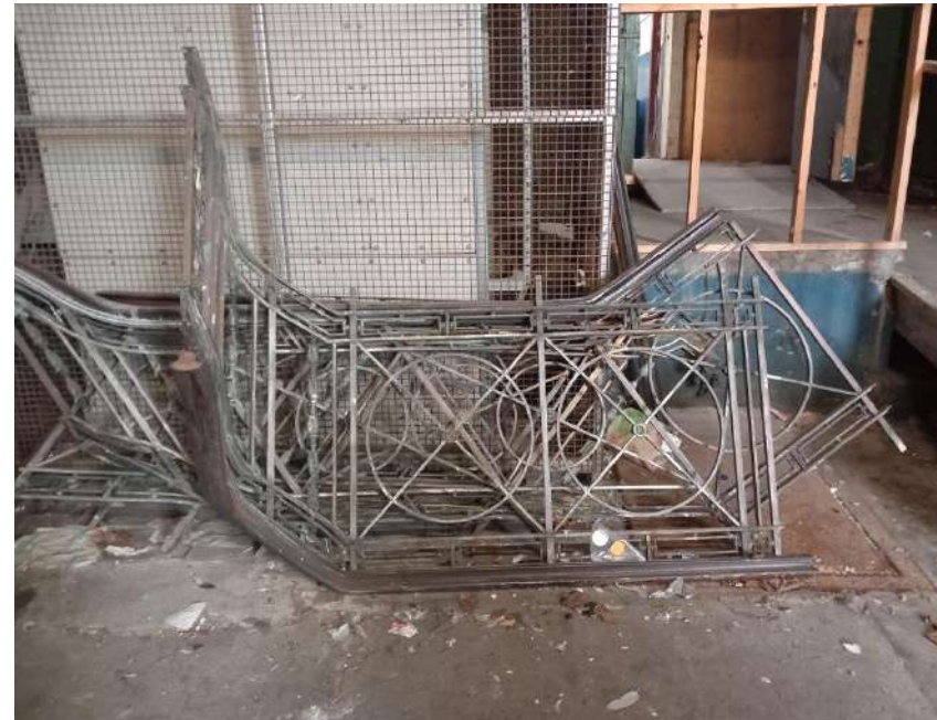
Plate 52 The original balustrade pertaining to the stairs in Independent House have been cut and dismantled. The high-quality sections and are in a salvageable condition and will be reinstated in their original location.
