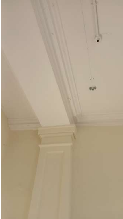
Plate 160: Cornices and panelling details to columns and pilasters and bressummer beams.
