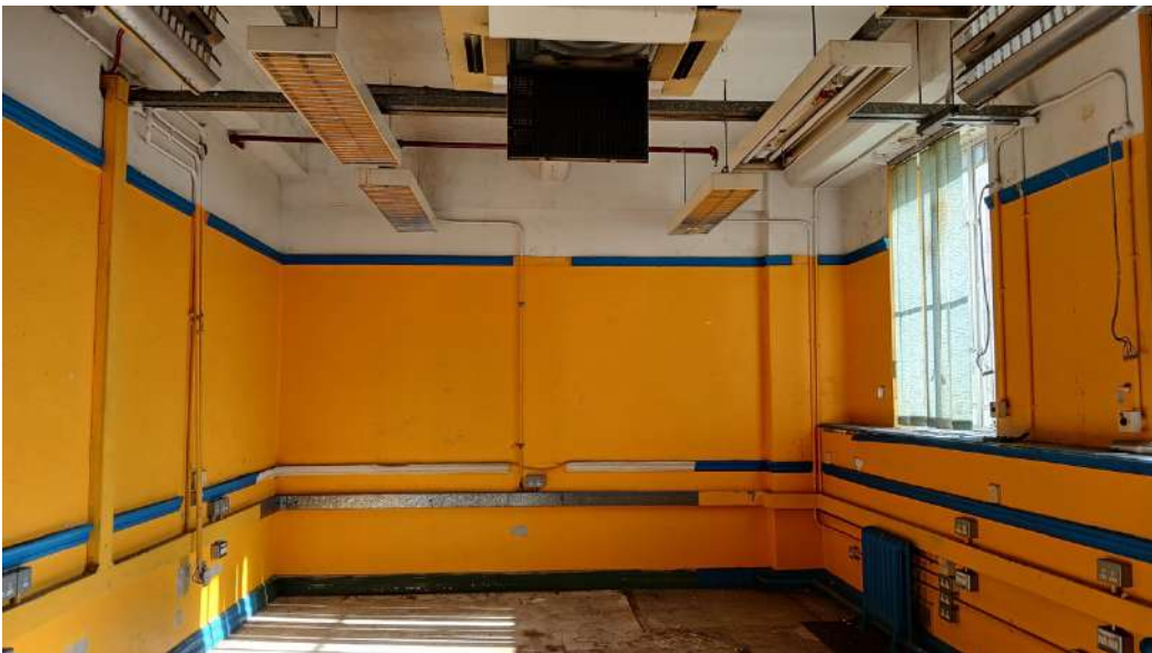
Plate 67: Typical cellular office, with concrete bressummers. Exposed contemporary services throughout. Note the continuous sill detail to the windows.
