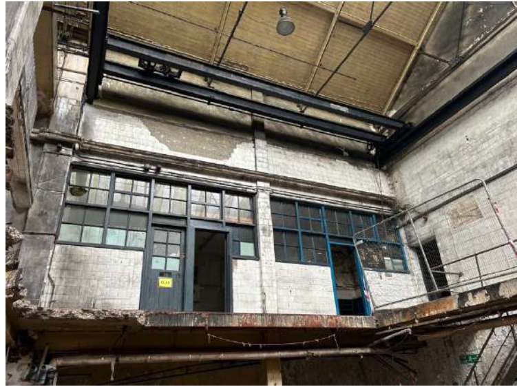
Plate 202: Offices at southern end of Printing Hall. The upper level ground floor slab has been partially demolished. Original timber screen walls and door-set with vertical boarded to lower panel and glazed upper panel, subdivided into six panes.
