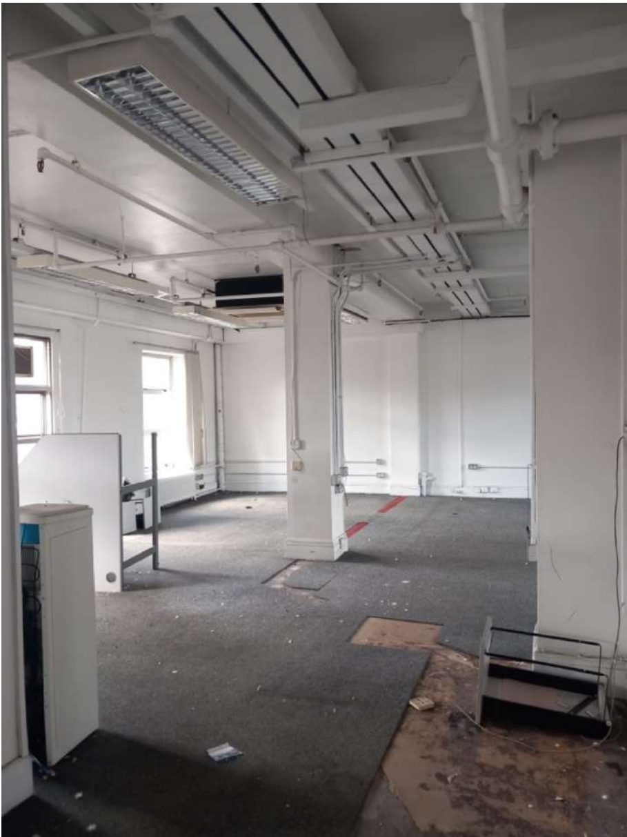
Plate 167: Open plan office. Plain run cornice, original metal windows, surface mounted services. Cornices and panelling details to columns and pilasters.
