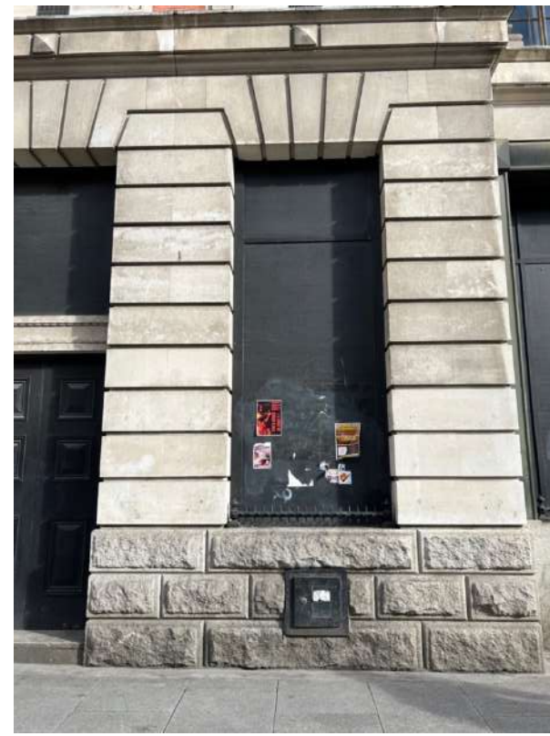
Plate 16: Typical ground floor window with cill guard.
