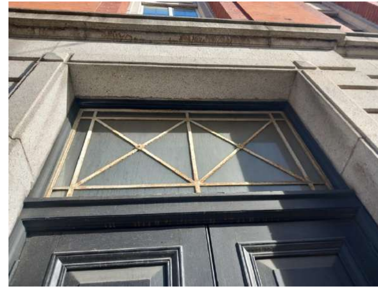
Plate 111: Detail of original metal-framed transom light.
