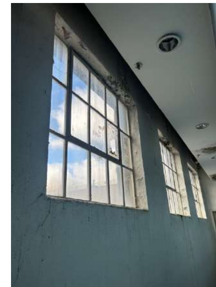
Plate 257: Original metal framed windows, 5 x 3 pane with 6 panel central pivot opening section.
