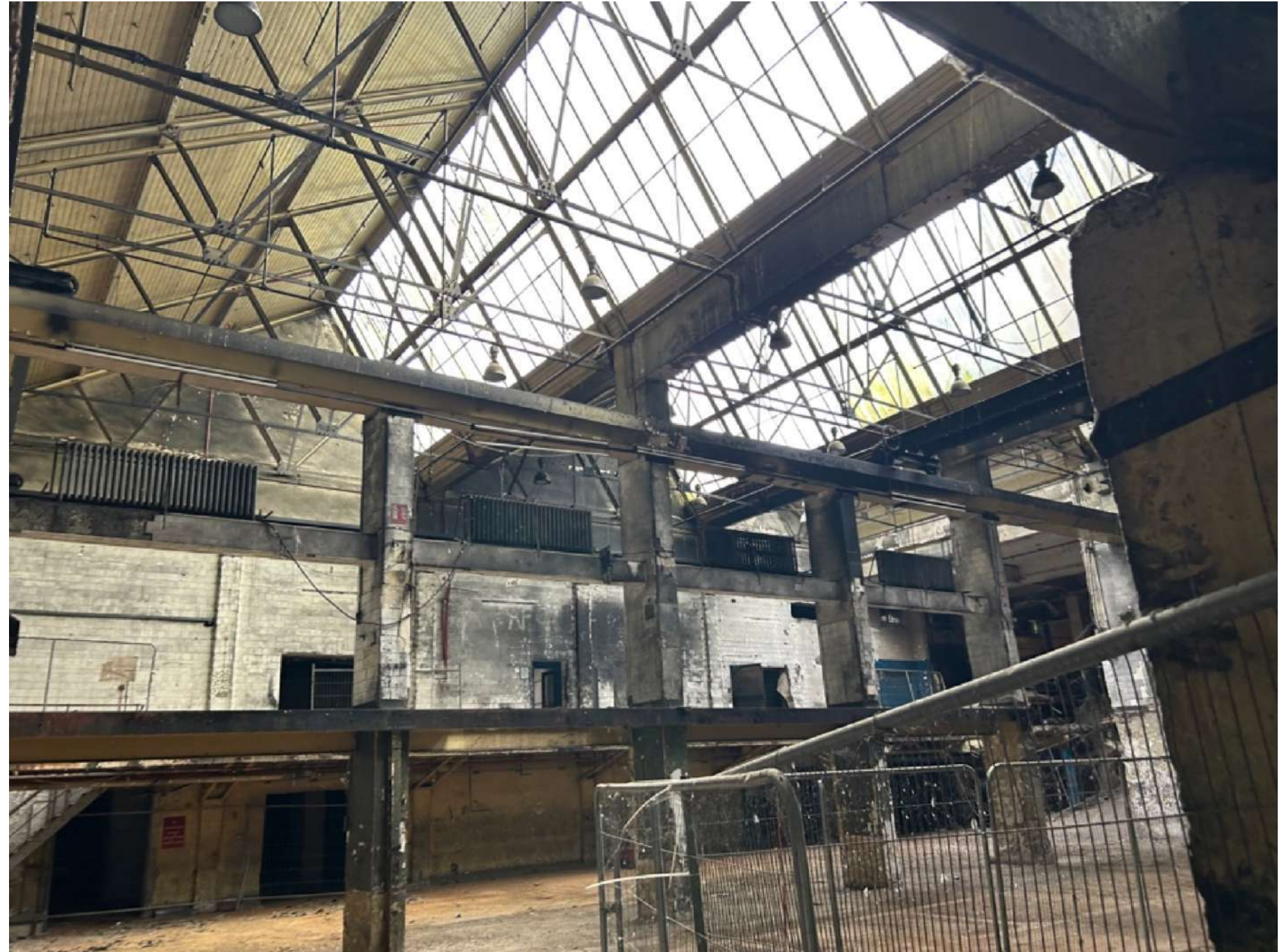
Plate 199: View from western side of Printing Hall towards south east. The central row of masonry column subdivide the hall; cartographic research suggests that the western side of the hall was a later addition. The columns supported a gallery at upper ground level, now demolished.
