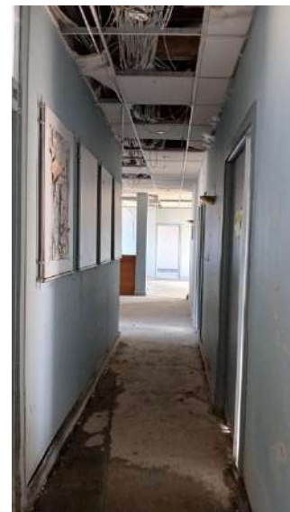
Plate 87: Contemporary partitions and doors on fourth floor level.
