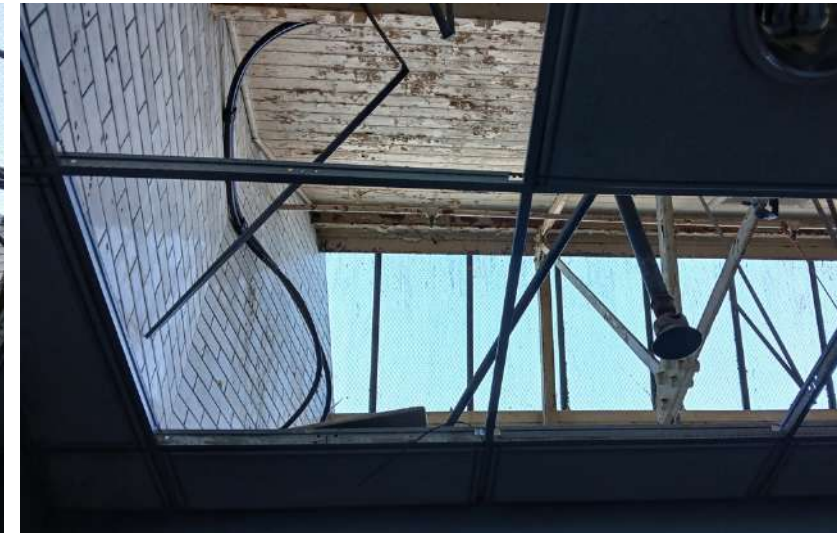
Plate 84: Concealed above contemporary suspended ceiling: the pitched roof at the rear of the main roof. Patent glazing system with replacement wired glass panels. Lightweight metal truss roof structure.
