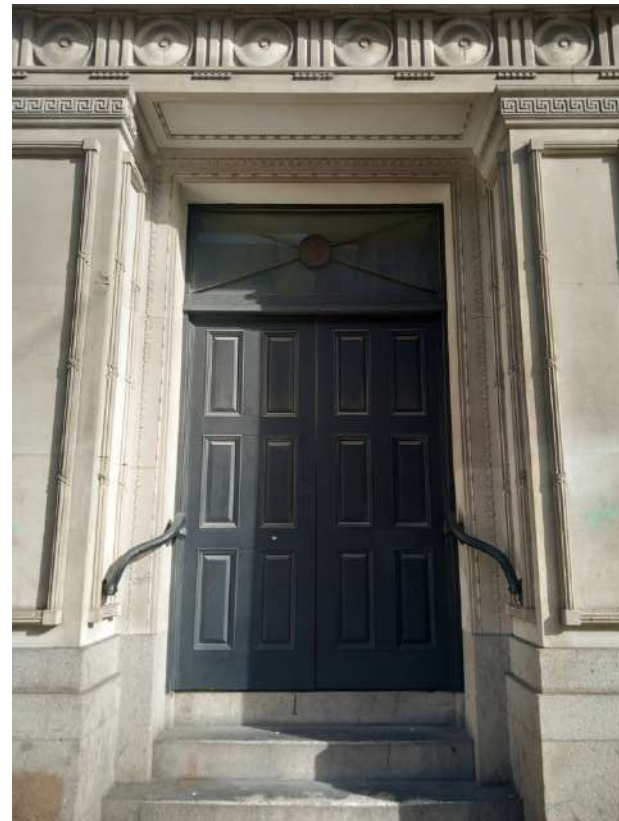
Plate 4: Replacement double doors, with pair of heavy handrails fixed to stone reveals.
