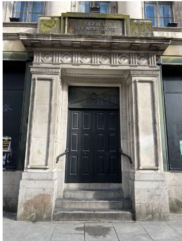
Plate 3: Replacement double-leaf timber panelled central front doors with projecting Portland stone doorcase surround. Original rectangular overlight with diagonal bracing, and four granite steps. Architrave surround flanked by large, panelled piers with Greek key capitals rising from granite plinths supporting full Doric entablature with metope-triglyph frieze.
