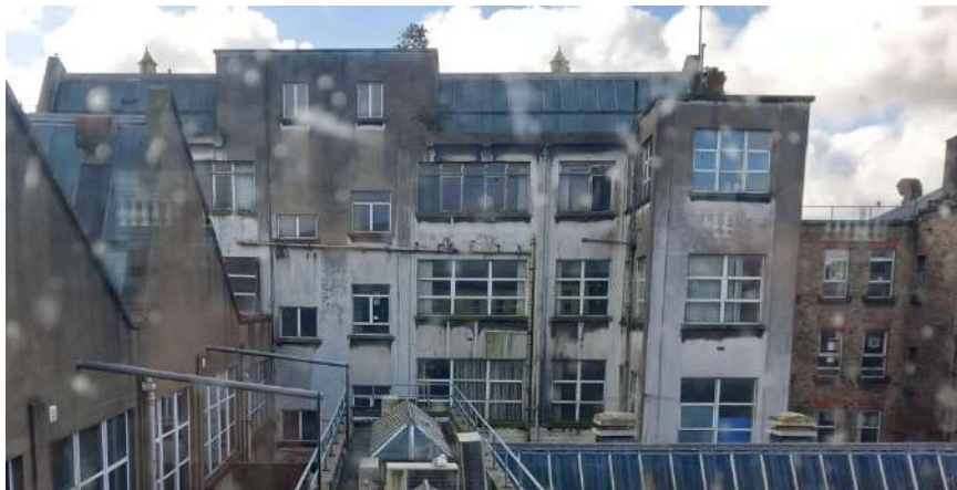
Plate 2 The rear elevation of 87-90 Middle Abbey Street, Independent House [Zone 1].
