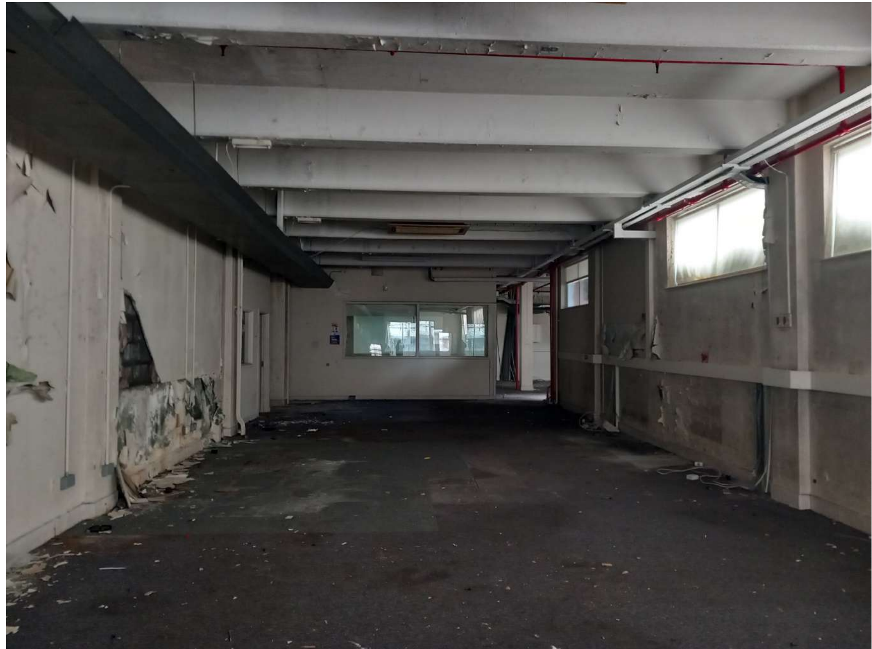
Plate 259: Facing east. Beams spanning in a north-south orientation. Contemporary partitions and internal glazing at the eastern end of the space.
