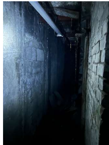
Plate 124: Narrow corridor orientated on an east-west axis at the rear boundary basement wall of 87-90 Middle Abbey Street.
