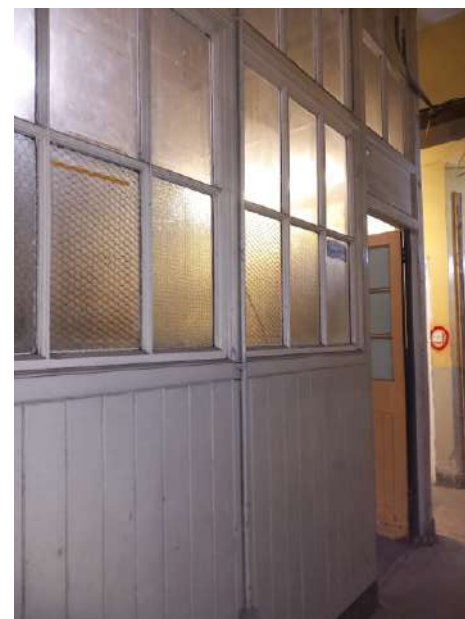
Plate 244: Original partitions screen wall with vertical timber boarding at lower level and multipaned glazed screen over.
