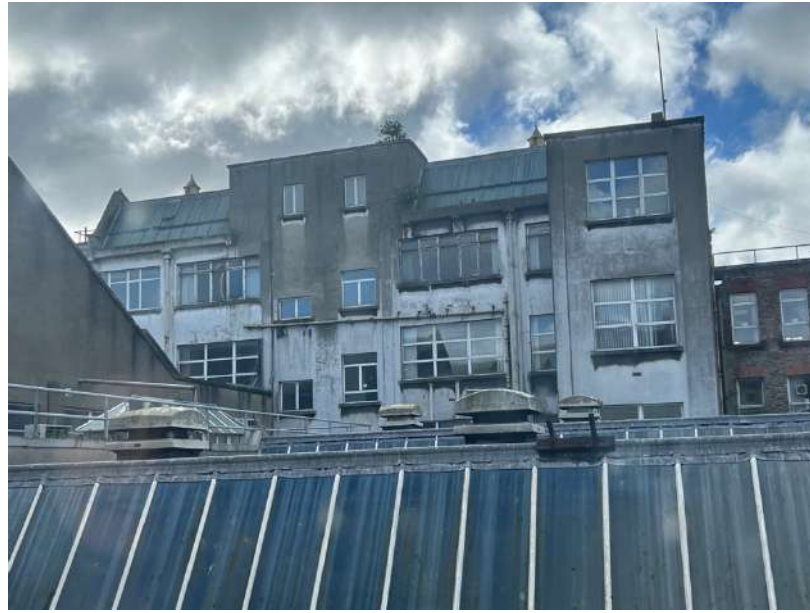
Plate 18: Rear façade of Independent House, render finish, cast iron rainwater goods, mixture of original and later uPVC windows. North-facing rooflights to upper floor.
