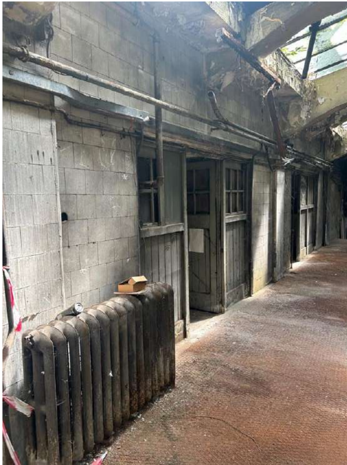
Plate 53 Original timber screen, with glazed doors, tiled finishes and exposed concrete frame structure will be retained, refurbished and integrated into the new development
