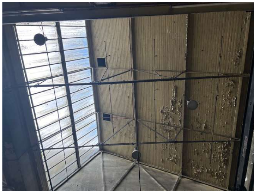
Plate 200: Typical roof bay; four lightweight steel trusses, with glazed panels to northern pitch (subdivided into 5 x 2 panels between trusses. Painted timber cladding to underside of south-facing pitch. Square opening section to roof vents. Original industrial light fittings.
