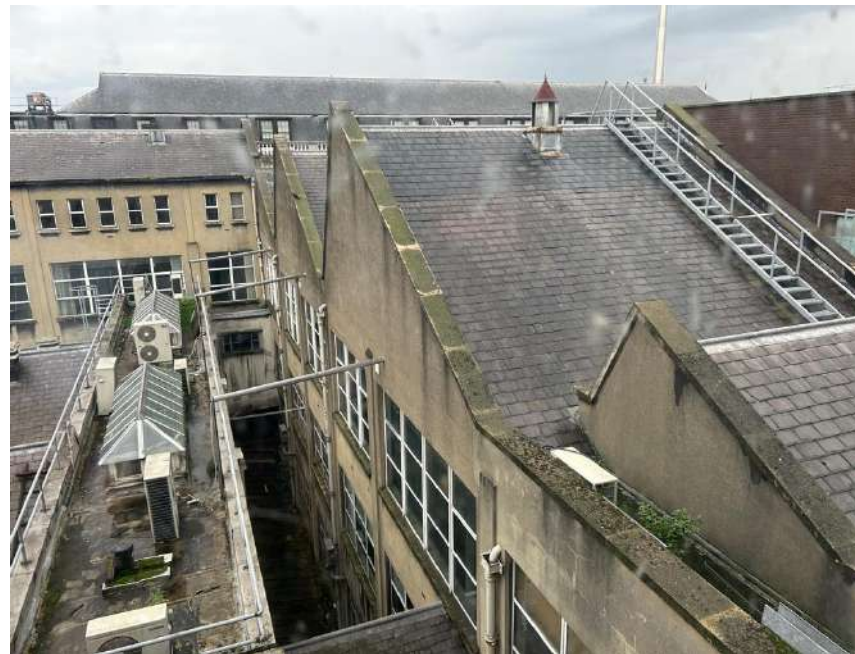
Plate 21: Sawtooth roof profile of Area 4. To the east of the narrow lightwell.
