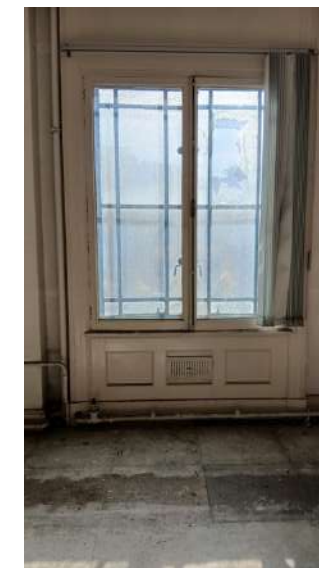
Plate 58: Original metal frames windows with margin lights externally, and timber-framed secondary glazing system with original ironmongery.
