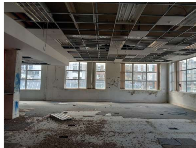
Plate 272: View facing south, overlooking roof of former Printing Hall. uPVC windows, raised access floor, contemporary lay-in ceiling tiles. Former open plan office space.
