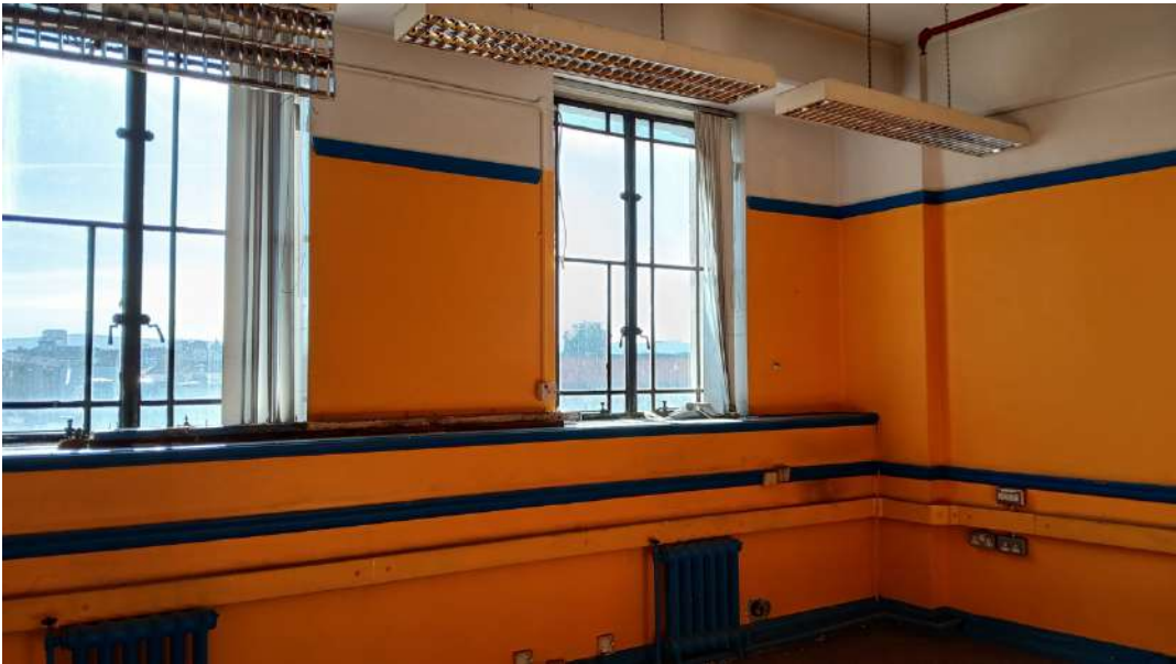
Plate 69: Cast iron casement windows with margin lights, original ironmongery. Continuous window sill along length of room.
