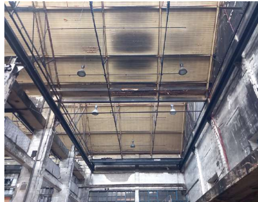
Plate 192: West side of Printing Hall roof, facing south. Heavy steel beams spanning east to west supporting a series of lightweight trusses of sawtooth roof. Original sarking boards and tiled finishes at upper level.
