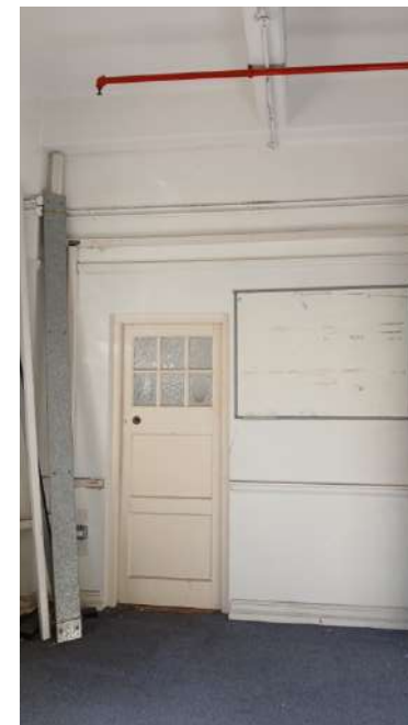
Plate 52: Original joinery on level 1, with three panelled door with multipaned glazing on upper panel, moulded architrave, skirting, dado and picture rail.
