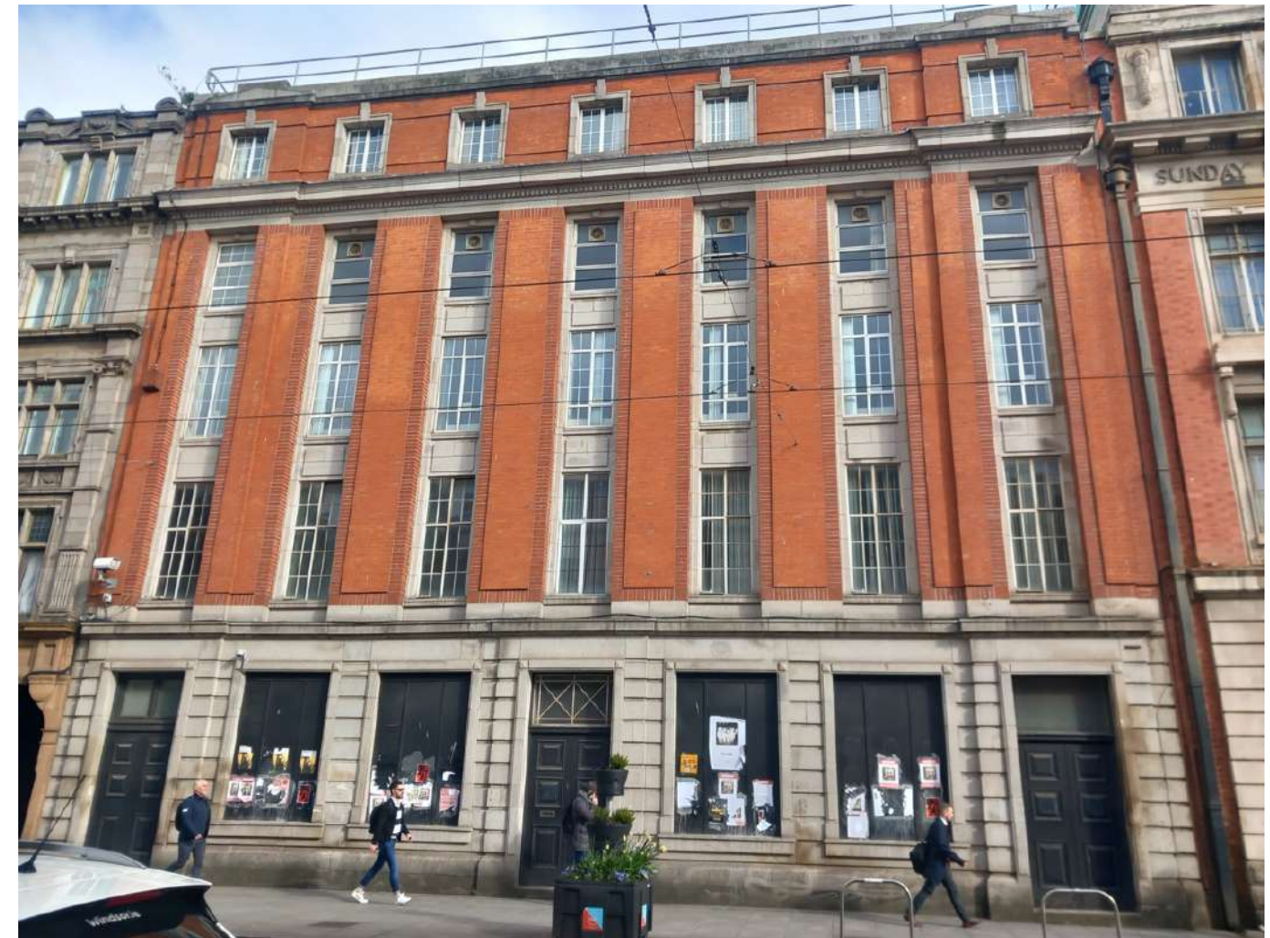
Plate 101: Front façade of 91-93 Middle Abbey Street.
