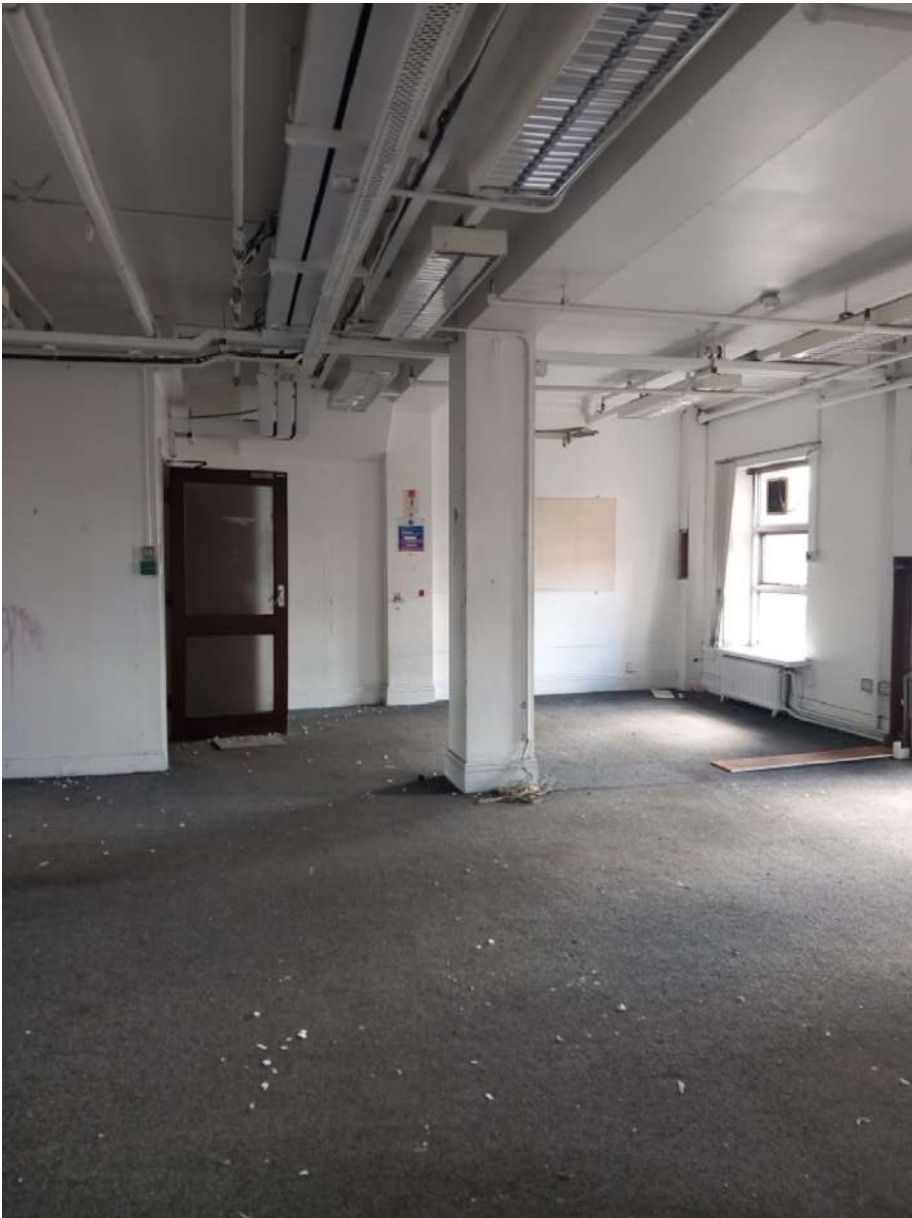
Plate 168: Open plan office. Plain run cornice, original metal windows, surface mounted services. Concrete floor slab.
