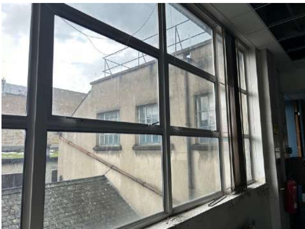
Plate 223: View of rear of Zone 4, as viewed from Zone 4, Original metal window frames.
