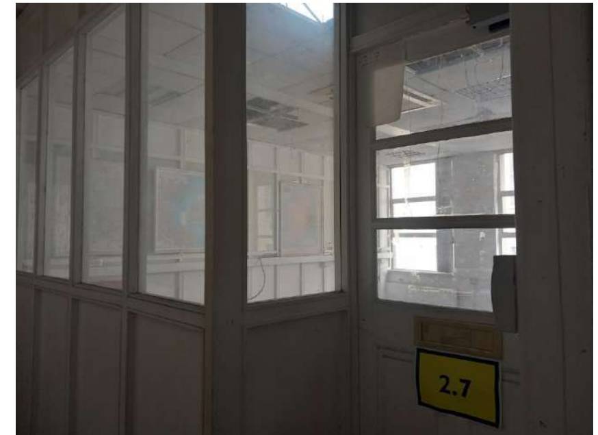
Plate 264: Contemporary partitions and wall linings on Level 2.
