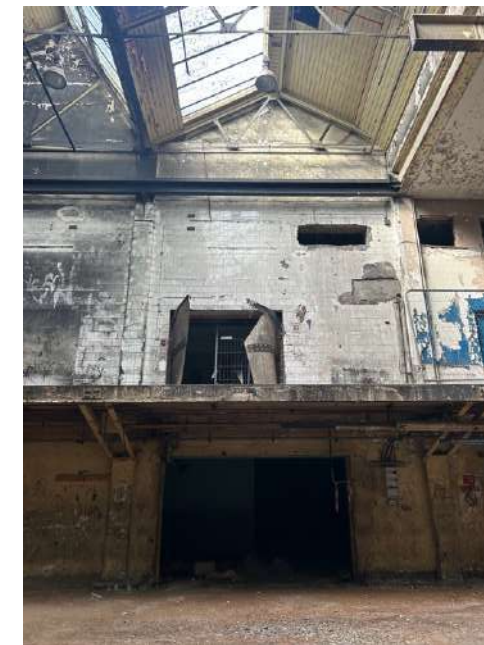
Plate 197: View facing west. Undercroft, beneath Zone 5 is accessed via the square headed opening under the upper ground floor gallery. Upper level walls are clad in glazed white tiles, in square format, laid in running brick bond.
