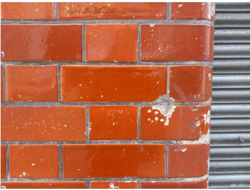
Plate 221: Detail of glazed ceramic brick with bullnosed detail to reveal at former vehicular entrance. Contemporary security shutter.
