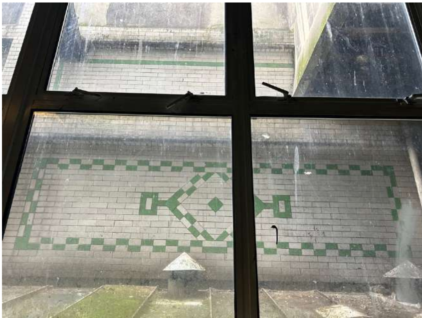
Plate 228: Detail of decorative pattern on glazed brick in lightwell in Zone 4..
