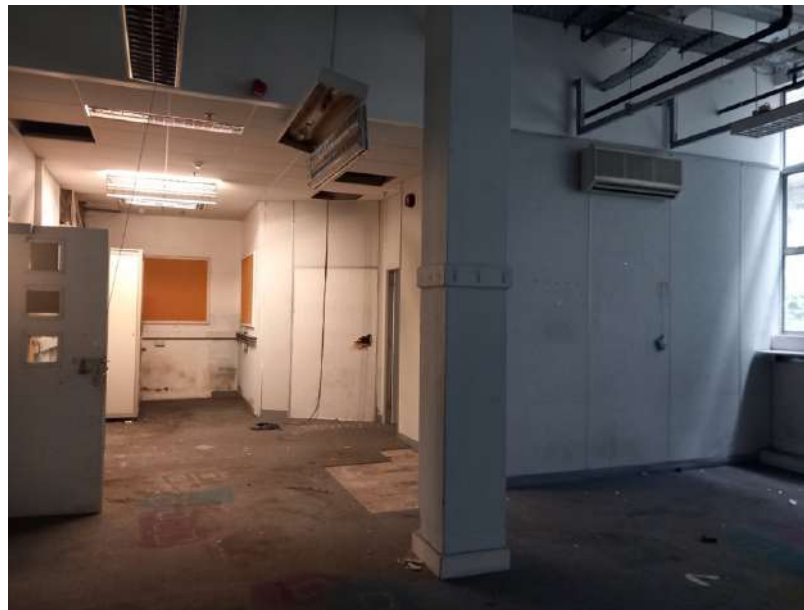
Plate 246: Contemporary partition walls forming office in south-west corner of room. Contemporary suspended ceiling, uPVC windows. No features of architectural heritage.
