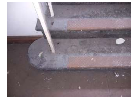
Plate 4 Detail of bullnose bottom step and inset incised metal nosings on the treads.
