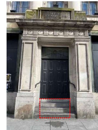
Plate 38: Existing stepped entrance to Independent House, which is proposed to be amended to create level access.
