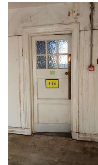
Plate 56: Limited remains of original joinery on level 2: panelled door with multipaned glazing un upper panel
