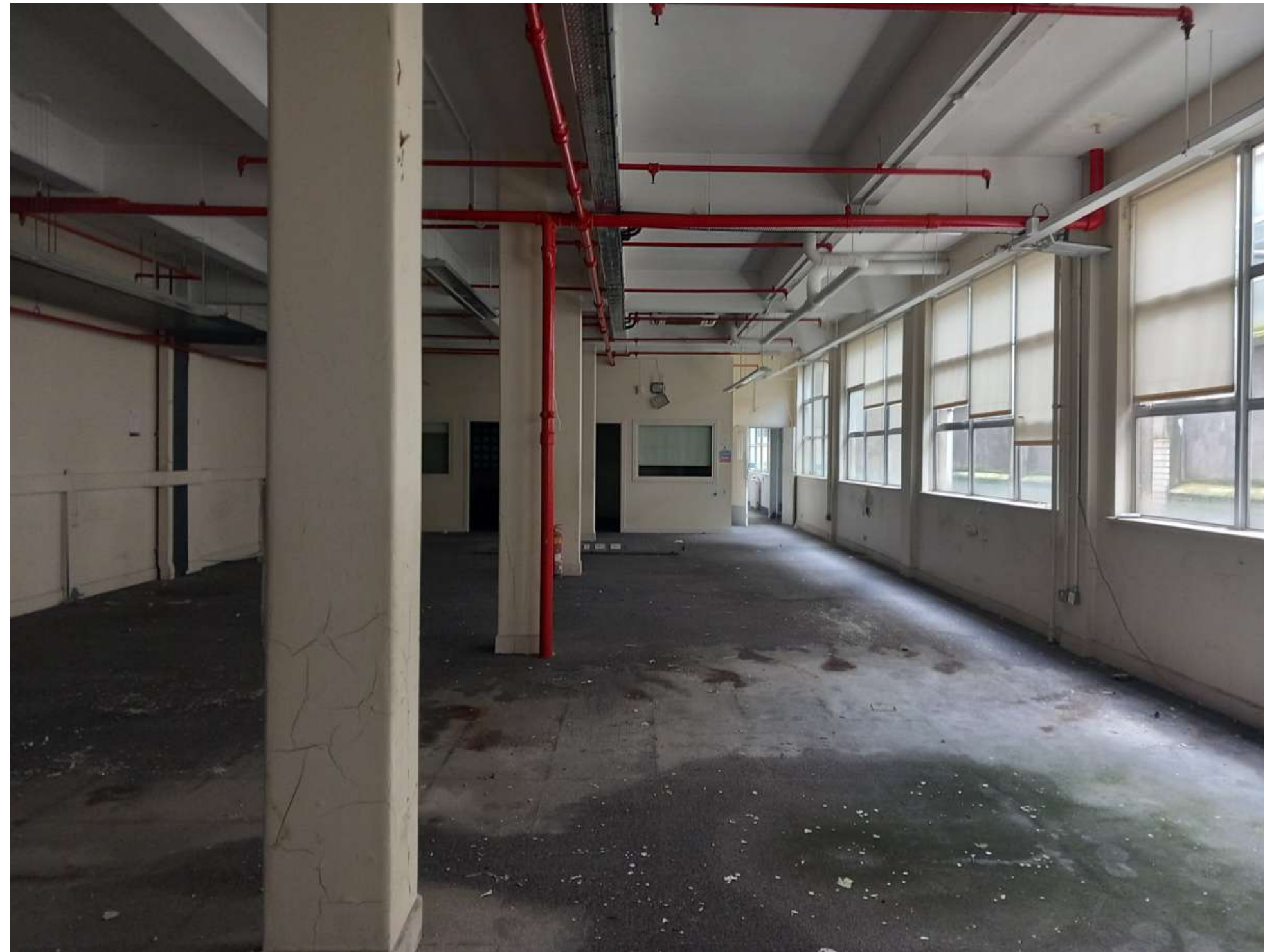
Plate 247: Zone 4, facing south, with linear lightwell to the right. Steel and concrete frame structure, replacement glazing. No finishes of architectural heritage interest.
