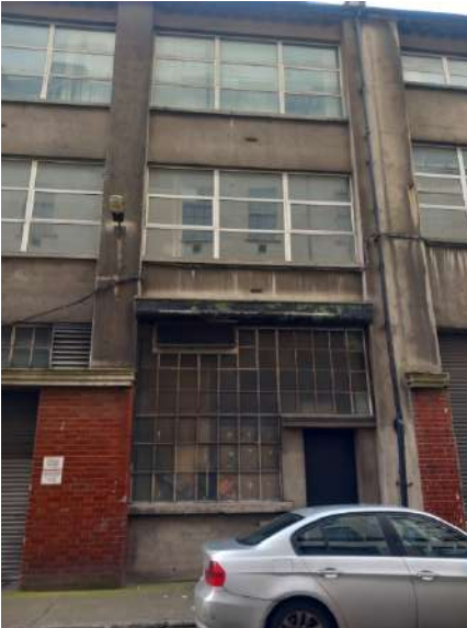
Plate 217: Multipaned metal framed window at ground floor level. Single leaf door surmounted by stepped cornice.
