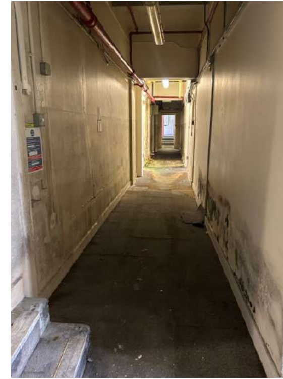
Plate 254: View facing west down central corridor. Layout appears to be original, but limited features of architectural interest observed.
