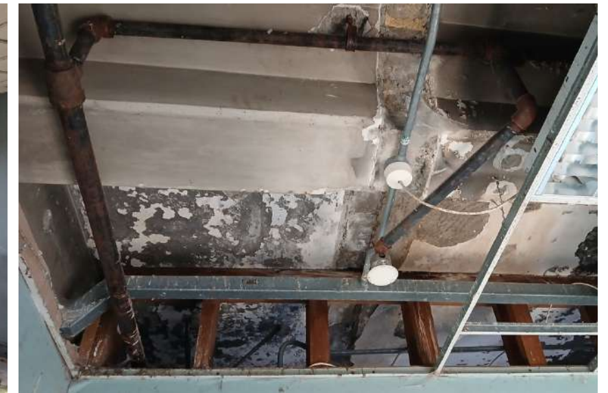
Plate 95: Scarring in concrete roof structure indicates position of original dividing walls internally.
