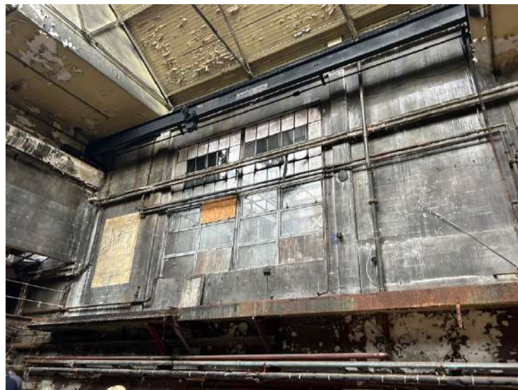
Plate 206: Glazed screen on southern wall, comprised of multipaned metal framed windows at west side of Printing Hall opening onto lightwell at the rear of Independent House.
