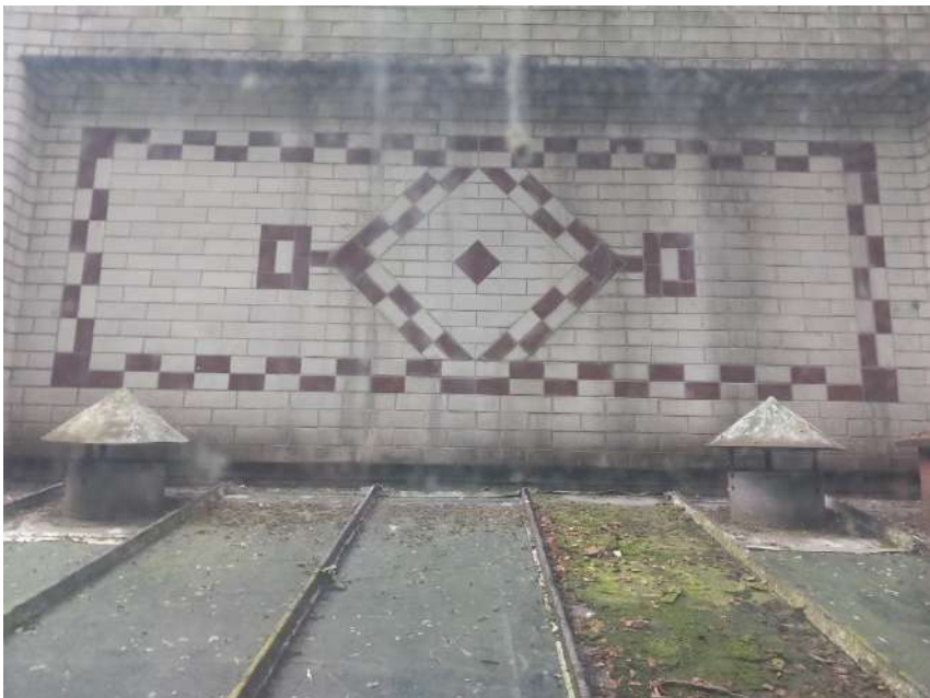
Plate 227: Detail of decorative pattern on glazed brick in lightwell in Zone 4.
