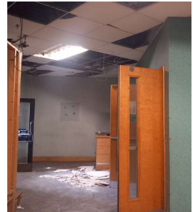
Plate 44: Entrance lobby, with contemporary doors, partition walls and fittings, suspended lay-in ceiling tiles. Original decorative ceiling noted above later ceiling.
