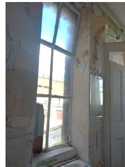
Plate 157: Multipaned steel framed windows.
