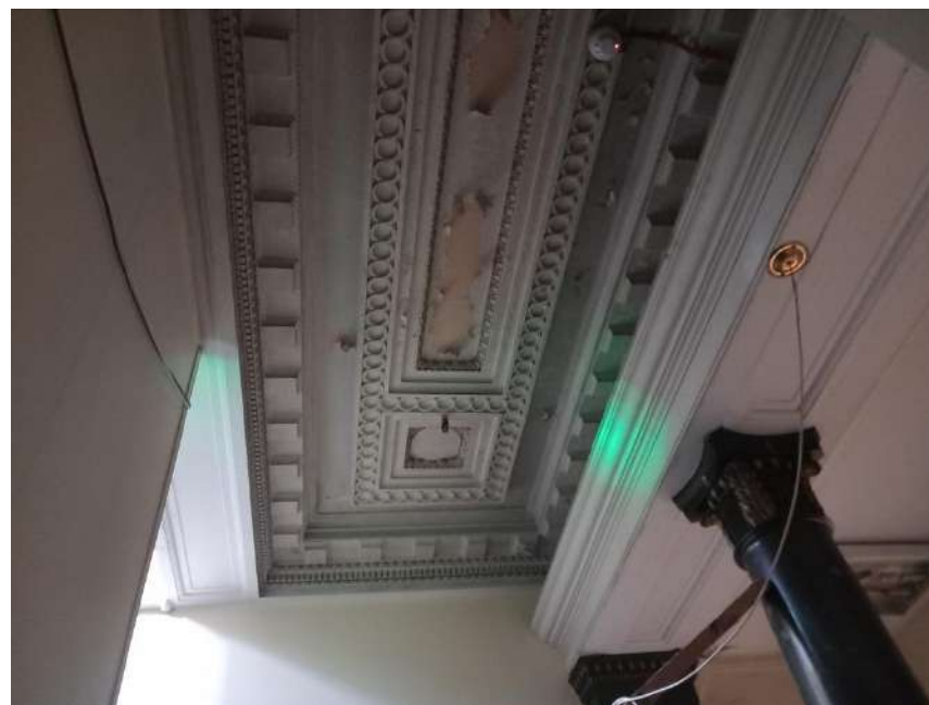
Plate 8 The ceiling in stair hall features a neoclassical geometric design.
