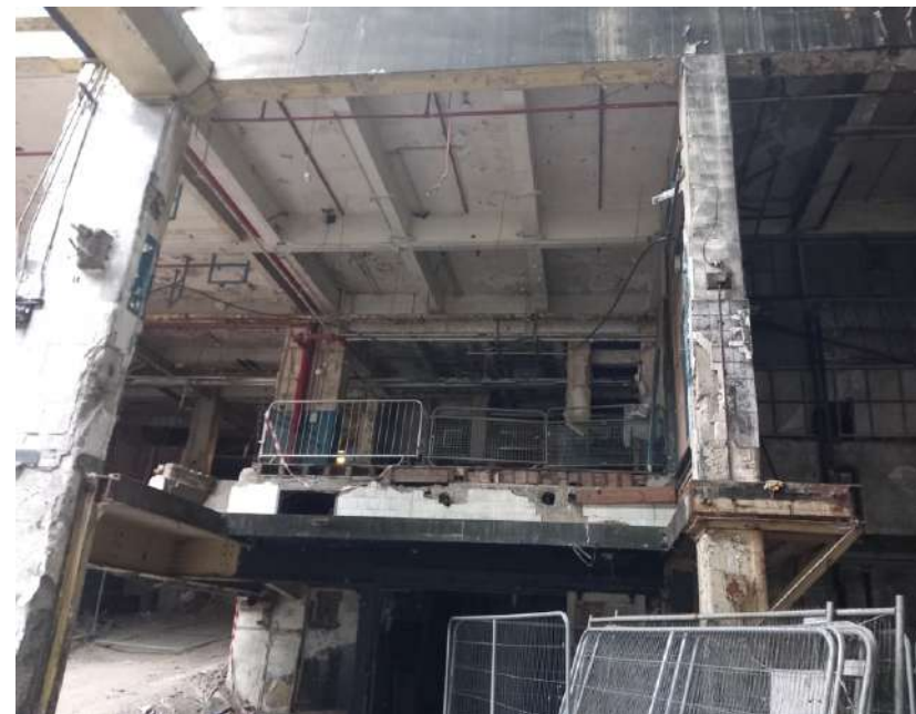
Plate 196: View from within former Printing Hall facing north and upwards towards ramp to entrance (Zone 4) on Prince's Street North. The gallery floor has been demolished in this area. The steel and concrete frame structure supporting upper floors of Zone 4 is visible to underside of floor above.
