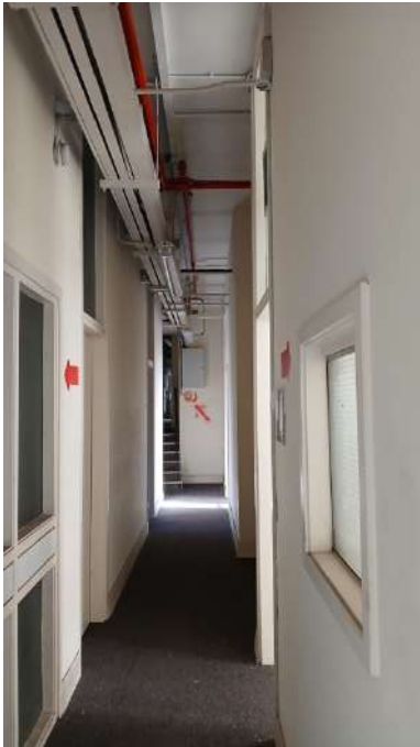
Plate 163: Contemporary partition walls along central corridor.
