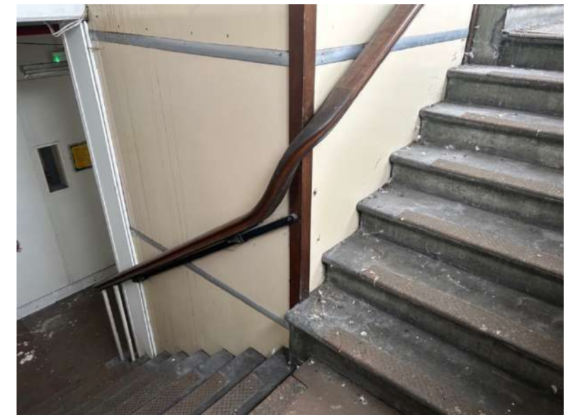
Plate 42: Hardwood handrail fixed to lift shaft in stairwell. Contemporary doors to lobby.
