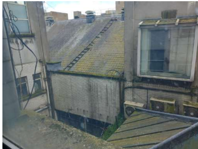
Plate 185: Lightwell to south of Former Printing Hall, attached to rear return of Independent House and Zone 4. Slate finish to south-facing pitch of sawtooth roof. Glazed white brick finish to lightwell. The lower levels of the deep lightwells were lined with glazed brick due to their light-reflecting attributes.
