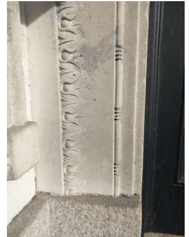
Plate 6: Detail of egg-and-dart and bead-and-barrel moulding on stone dressings.
