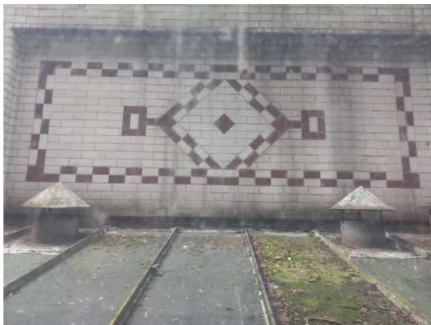
Plate 54 Original wall tiling on the external face of the printing hall will be retained
