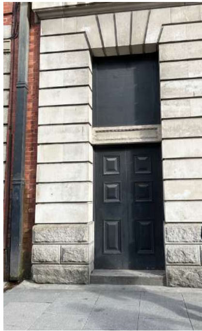
Plate 11: Secondary door with panelled lintel and square-headed over-light. Horizontally channelled ground floor, with rusticated plinth with plain margins. Single granite step to threshold.
