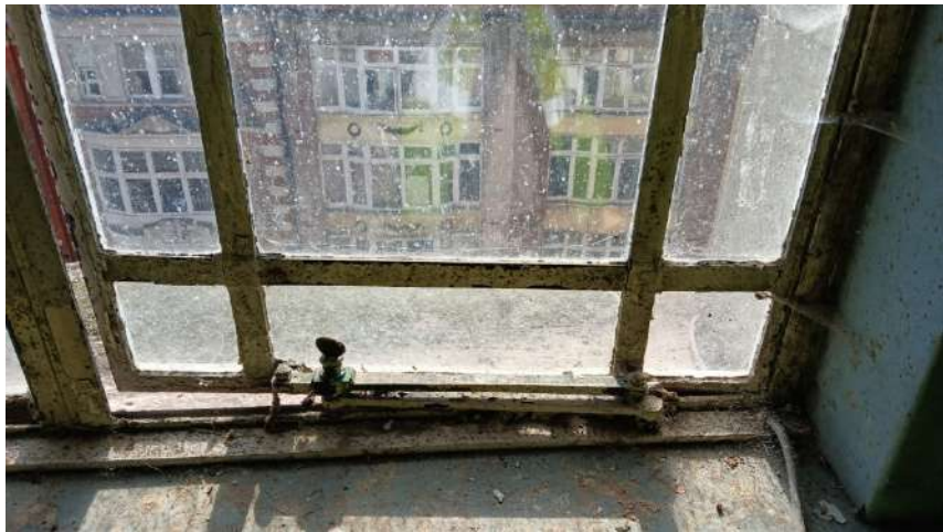
Plate 100: Original brass casement stay.
