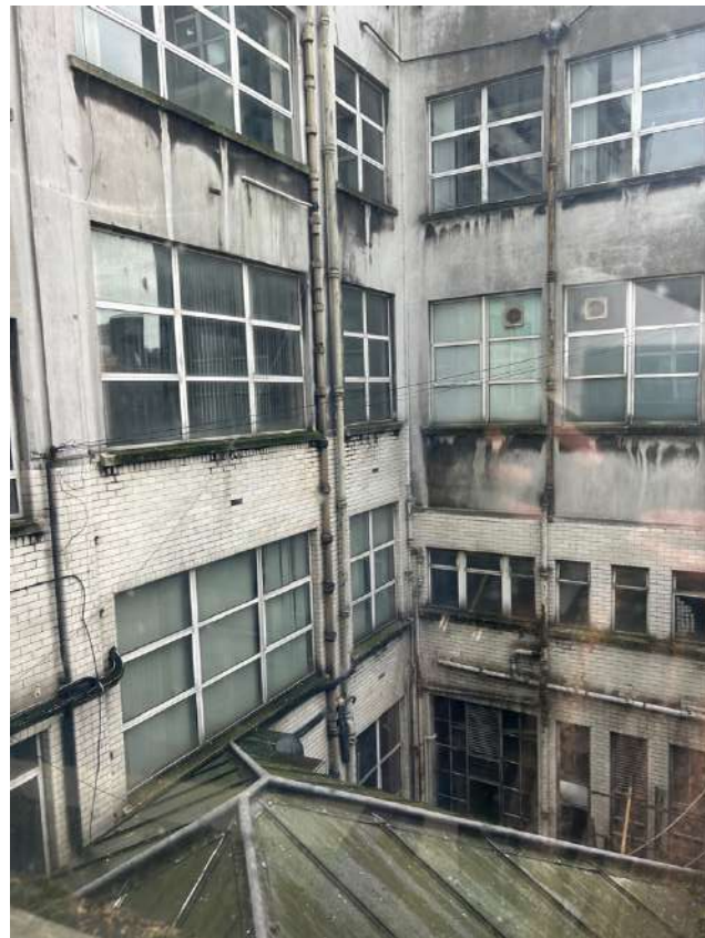
Plate 21: Rear façade of Independent House, with rear return shown to right. It appears that the rear return was vertically extended from original two storeys to 5 storeys.
