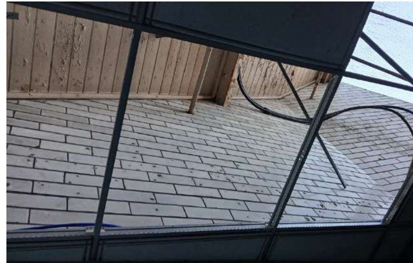
Plate 83: Glazed white tile finish to flanking walls of pitched roof. (Rear section of main roof). Painted timber boarding to underside of roof structure.
