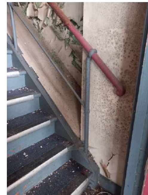
Plate 277: Industrial steel balustrade to stairs with ball joints.
