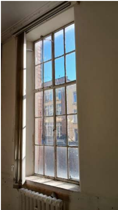
Plate 162: Metal frame windows with original ironmongery, rendered reveals with gently rounded rendered reveals.
