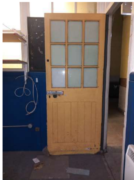
Plate 243: Original door joinery with vertical boarding to lower panel and multipaned glazed panel to upper. Original ironmongery. Door forming part of internal partition screen.
