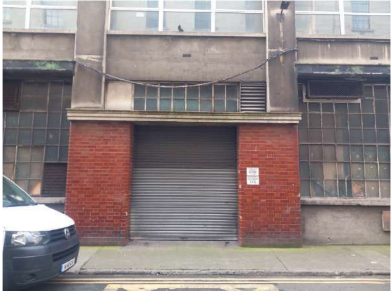
Plate 216: Former entrance on Prince's Street North; flanked by glazed brick piers with bullnose brick detail at corners and surmounted by Art Deco style stepped cornice. Original metal transom window above
