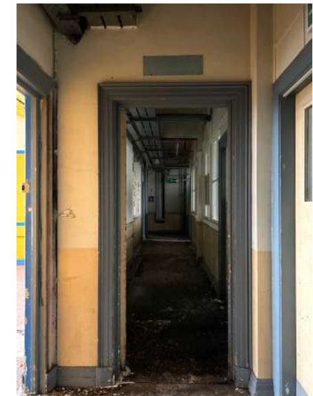
Plate 66: Original moulded timber architrave on blocks with stepped skirting. View down central spine corridor beyond, with original partition walls within interior multipaned screens. Exposed contemporary services throughout.
