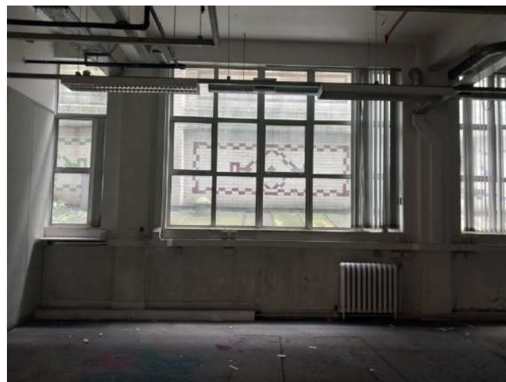
Plate 260: Zone 4 facing west towards linear lightwell. uPVC windows. Concrete bressummers to ceiling.
