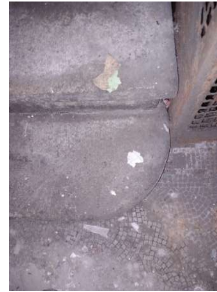
Plate 147: Granite stairs from ground to fourth floor level, with bullnose bottom step. Original mosaic floor in entrance laid in fan scallop pattern, with contrast boarder.
