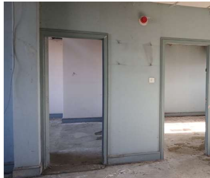
Plate 93: Contemporary joinery, contemporary wall linings and suspended ceiling at level 4.
