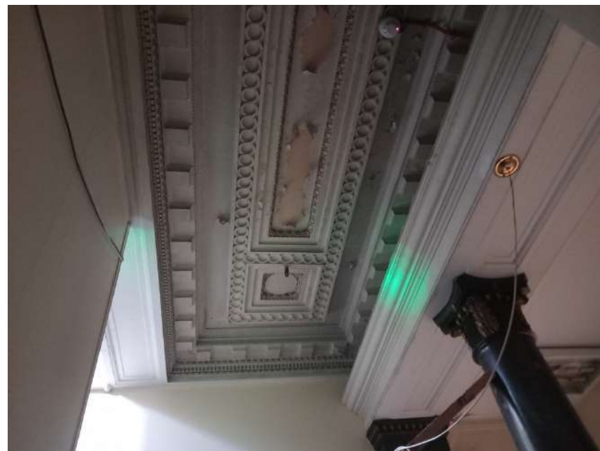
Plate 45: Neo-classical elements in entrance lobby of Independent House; Corinthian capital to columns, decorative plaster ceiling panels with egg and dart and modillion cornice, with inset panels framed with interlaced circle motif.
