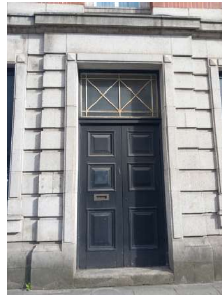
Plate 110: Central bay with double door with raised and fielded panels and transom light over, cut granite architrave and granite step to threshold.
