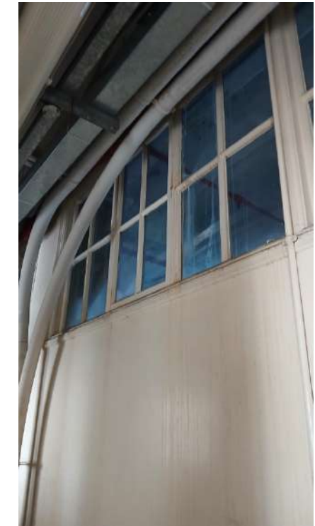
Plate 50: Detail of clerestory glazing with pivot opening sections.
