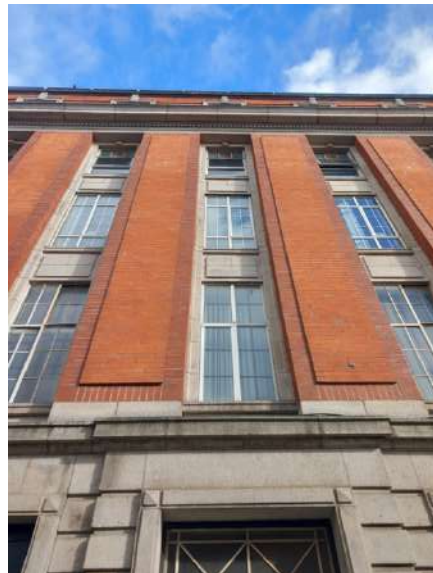
Plate 113: Detail of central bay. Raised brick panel laid in Flemish bond framed by soldier course. Mixture of uPVC replacement windows and original multipaned steel windows.
