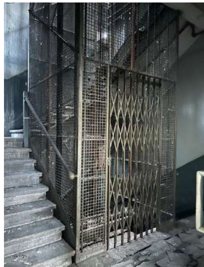
Plate 14: Handrail mounted on caged lift enclosure Plate 15: Underside of the granite stair lift enclosure
