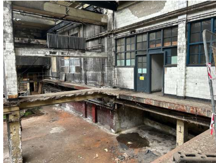
Plate 203: View from upper ground level facing south-west. The floor of the central gallery has been demolished.
