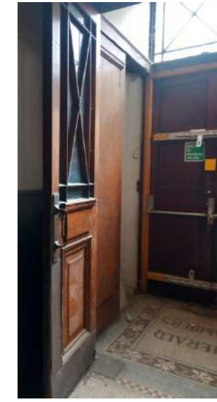
Plate 132: Internal lobby doors comprised of glazed upper panel with margin lights and diagonal cross bracing, raised and fielded panel at lower level, original ironmongery; pull handles and kickplate with floor springs.
