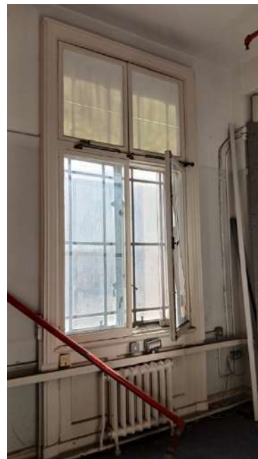
Plate 51: Level 1 windows: Original metal frames windows with margin lights externally, and timber-framed secondary glazing system with original ironmongery. Moulded architraves with panelled window apron.
