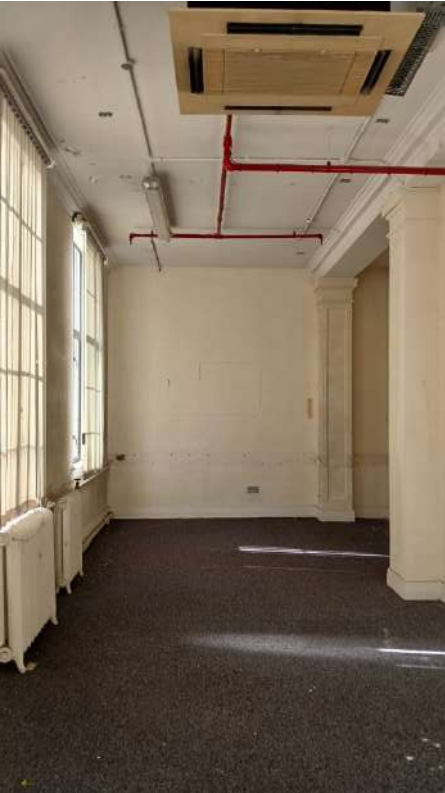
Plate 161: Open plan office. Plain run cornice, original metal windows, surface mounted services. Concrete floor slab.
