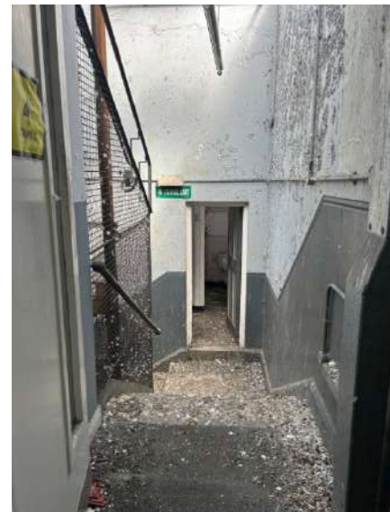
Plate 150: View from top of stairs towards quarter landing. Moulded timber skirting, dado integrated into wall render. Handrail fixed to lift enclosure.
