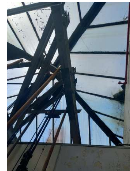
Plate 152: Pyramidal roof lantern above stair enclosure.
