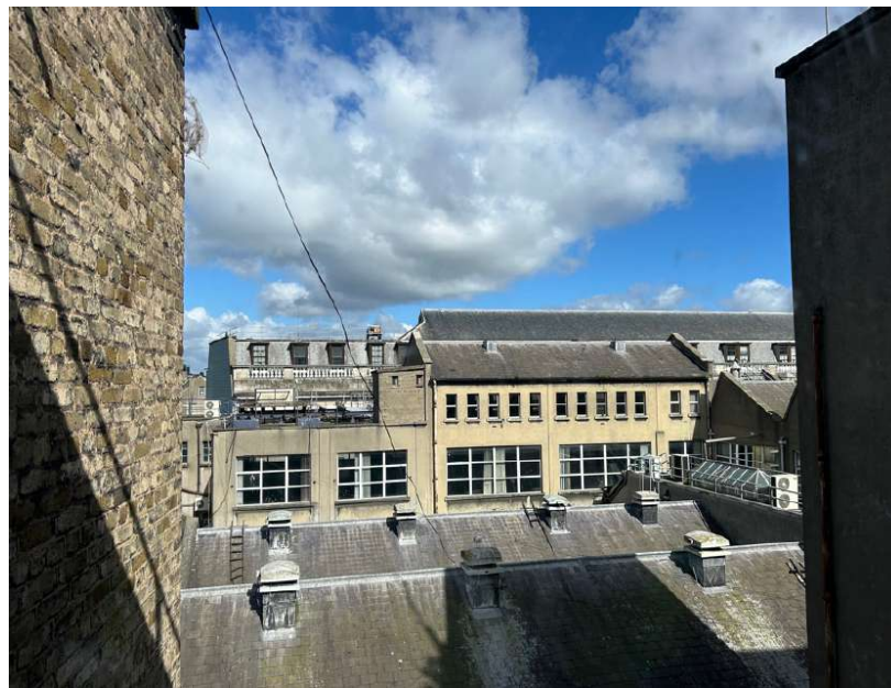
Plate 210: Rear (south facing) façade of rear building range Zone 4, with mansard roof of GPO visible in background.
