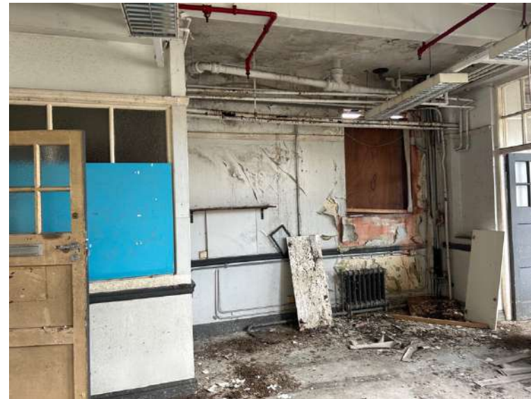
Plate 64: Rear room, facing west. Panelled door with glazed upper panel.
