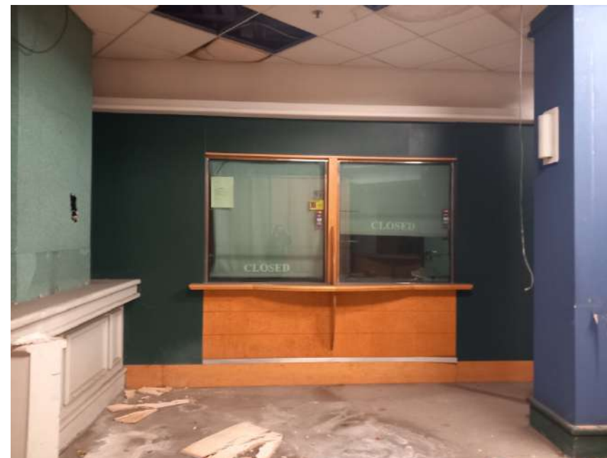
Plate 46: Contemporary fittings in entrance lobby. Original decorative ceiling noted above later ceiling.
