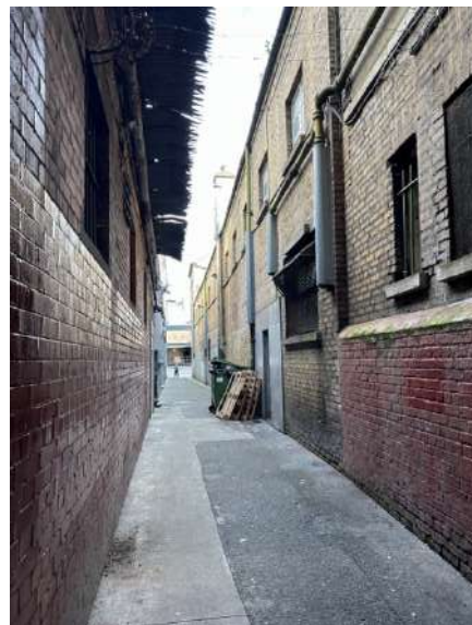
Plate 106: William's Lane facing north towards Princes Street. The western boundary wall of the subject site is faced in buff coloured brick.
