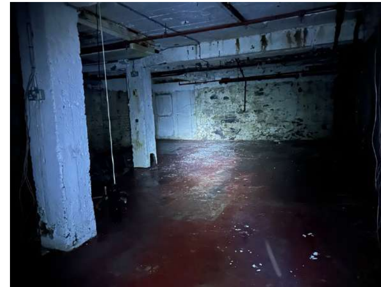
Plate 125: Concrete frame structure, with calp limestone wall enclosing basement wall.
