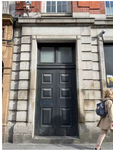
Plate 109: Double door with raised and fielded panels and transom light over, cut granite architrave and granite step to threshold.
