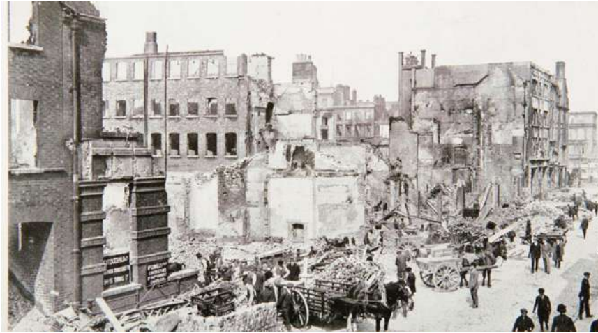
Plate 32: 'Post 1916 Rebellion – removing the debris from Middle Abbey Street. The former entrance to William's Lane to the extreme left of image. The site from William's Lane eastwards (left- to-right) was occupied by Fitzgerald's & Co. Wine and Spirit Store 91-93 Middle Abbey Street, The Nation Newspaper and Alexander Thoms.
