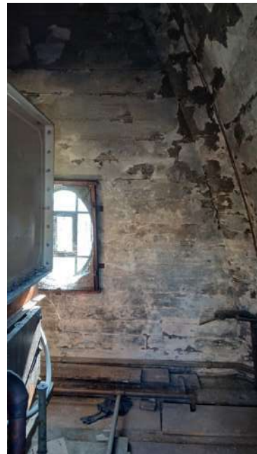
Plate 29: Interior of the west dome, with original oval window intact. Original and later water-tanks stored within west dome.
