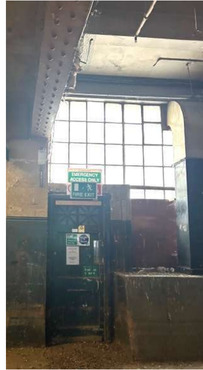
Plate 237: Former service entrance on Prince's Street North: Panelled door with decorative frame to transom light, multipaned metal framed window.
