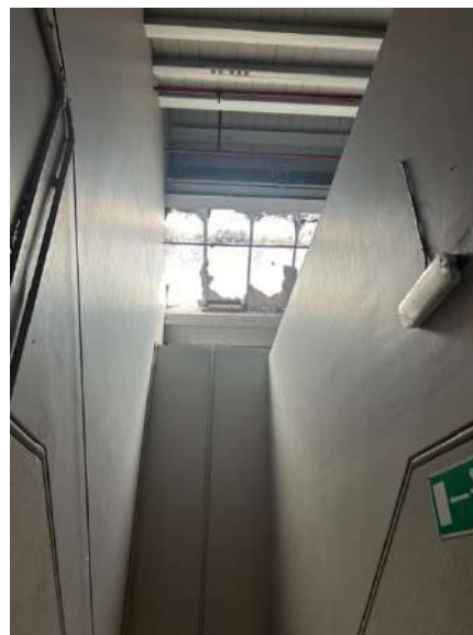
Plate 232: Dado rail integrated in render, with exposed sarking boards and rooflight to north facing aspect.
