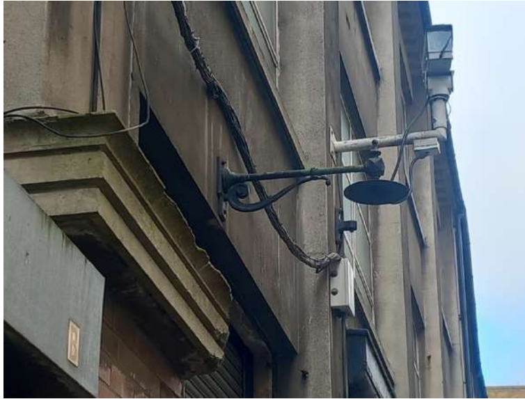
Plate 218: Detail of cornice and original wall mounted bronze light fitting over secondary entrance. Contemporary services fixed to cement rendered façade.
