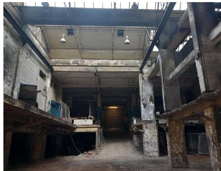
Plate 19: The western side of the Printing Hall, was added c1939.
