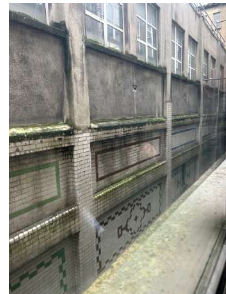
Plate 226: The lower levels of the lightwells between the rear buildings are faced in glazed white brick. This long liner lightwell between within Zone 4 has decorative geomatic designs using coloured glazed bricks.
