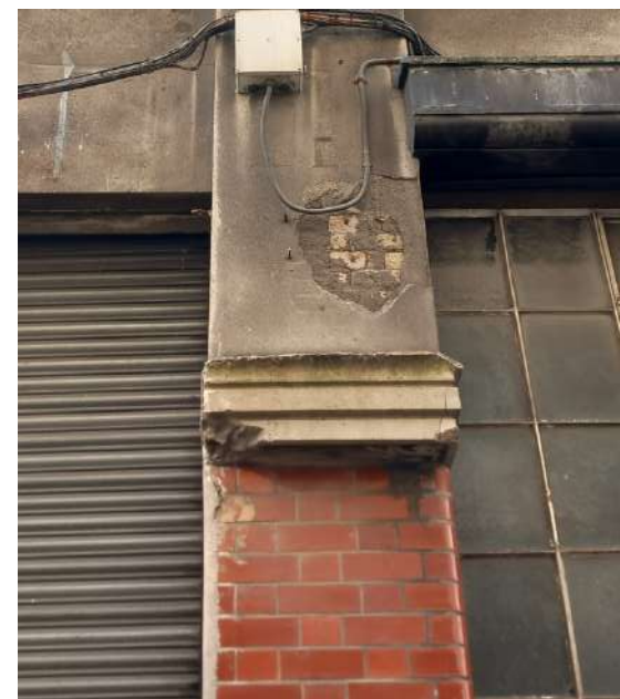
Plate 219: The external piers are comprised of brick; glazed ceramic at ground floor level, and localised failure in the render finish reveals the substrate at higher level to be buff brick. Impact damage to rendered cornice observed at openings and it is noted that the reveal to the secondary entrance has been faced in cement, adhered to the original ceramic brick face.
