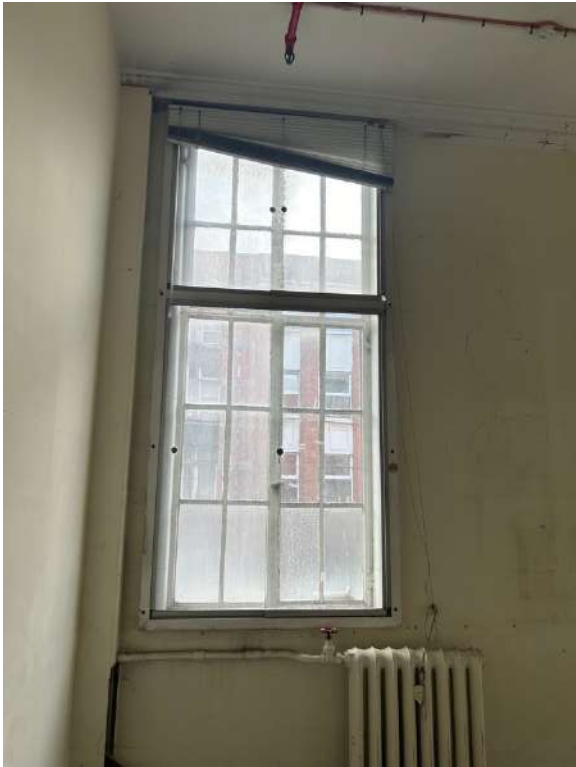
Plate 159: Cellular office. Plain run cornice, original metal windows with contemporary secondary glazing, surface mounted services. Later partition walls subdividing spaces.
