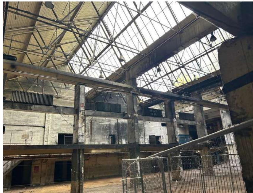
Plate 16: The interior of the Printing Hall (Zone 3)
