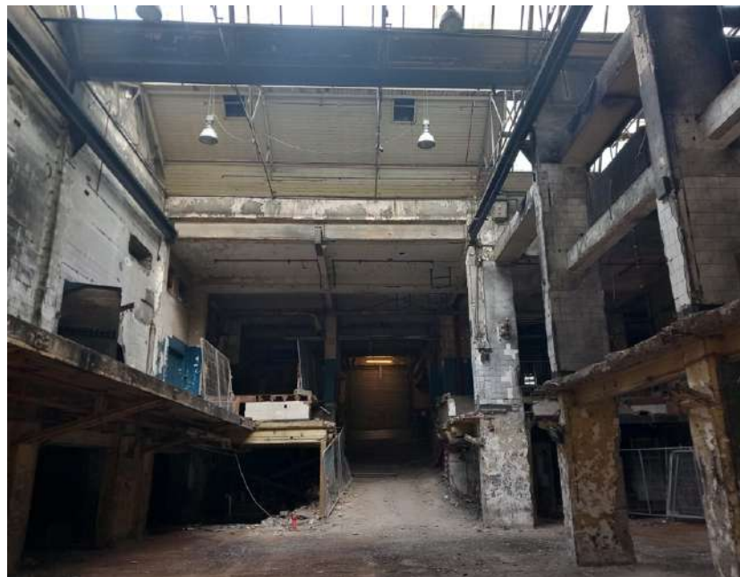
Plate 195: View from within former Printing Hall facing north towards recently formed ramp connecting to the entrance (Zone 4) on Prince's Street North. The structure has been partially demolished in this area, revealing the composition of the floors to be reinforced mass concrete.
