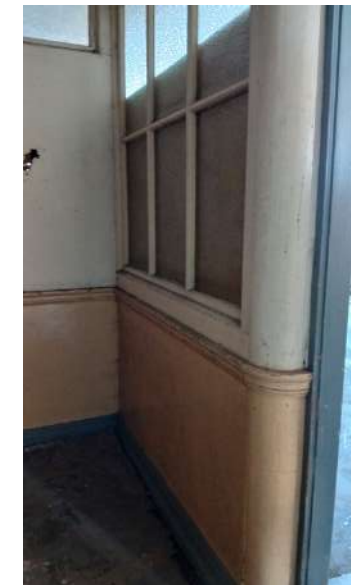
Plate 62: Original partition walls, with curved corner detail.
