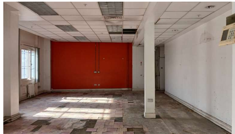
Plate 57: Level 2 has been extensively modernised to create an open plan office space. Contemporary wall linings and suspended ceiling. Original window fabric.
