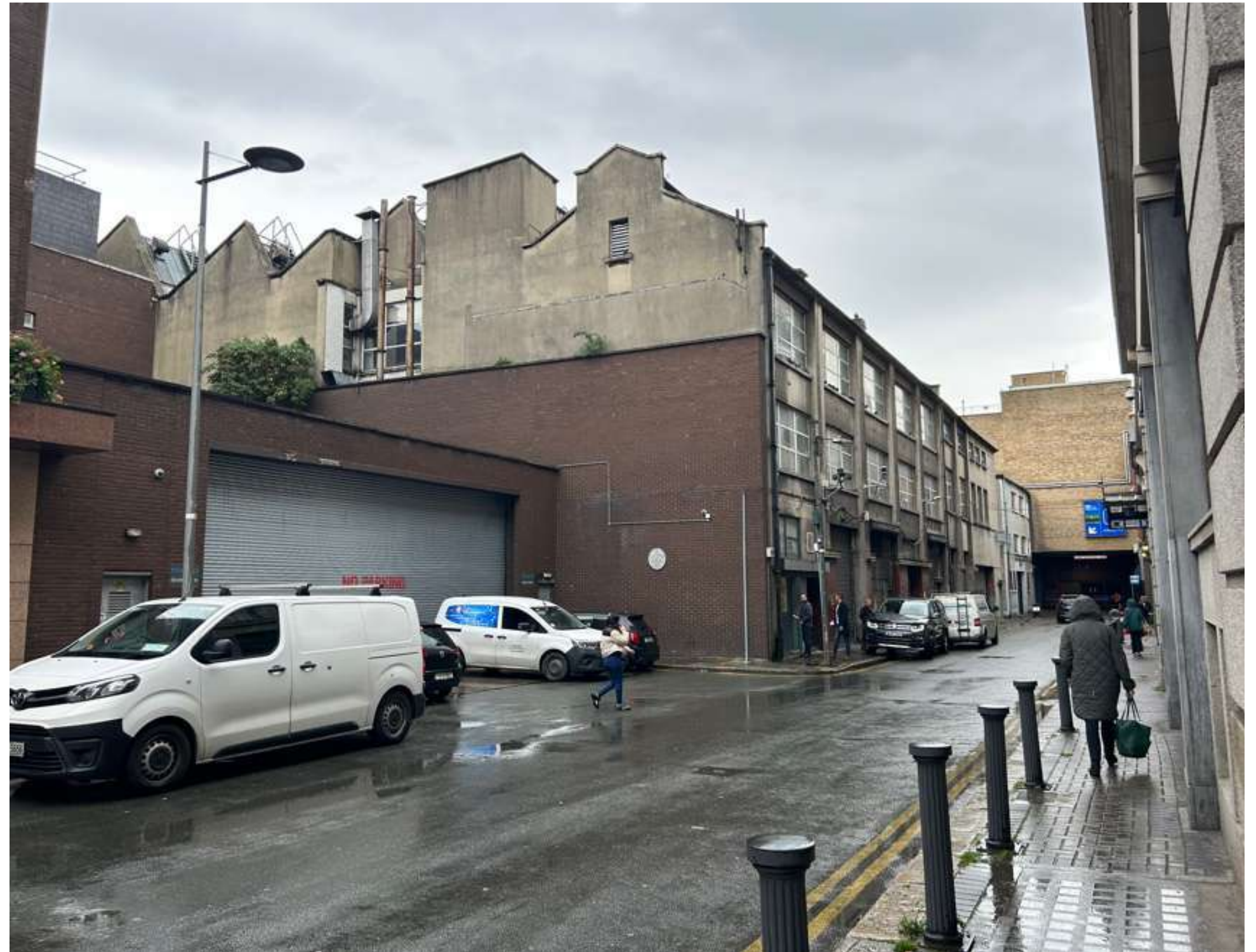
Plate 211: View facing west down Prince's Street North. The north-east corner of the rear building range. Sawtooth roof profile of rear building range Zone 4 visible. The contemporary red brick gable constructed against the gable wall is part of the adjacent 'Pennys' site. A plaque commemorating the site of The Capital Cinema is mounted on the later wall.
