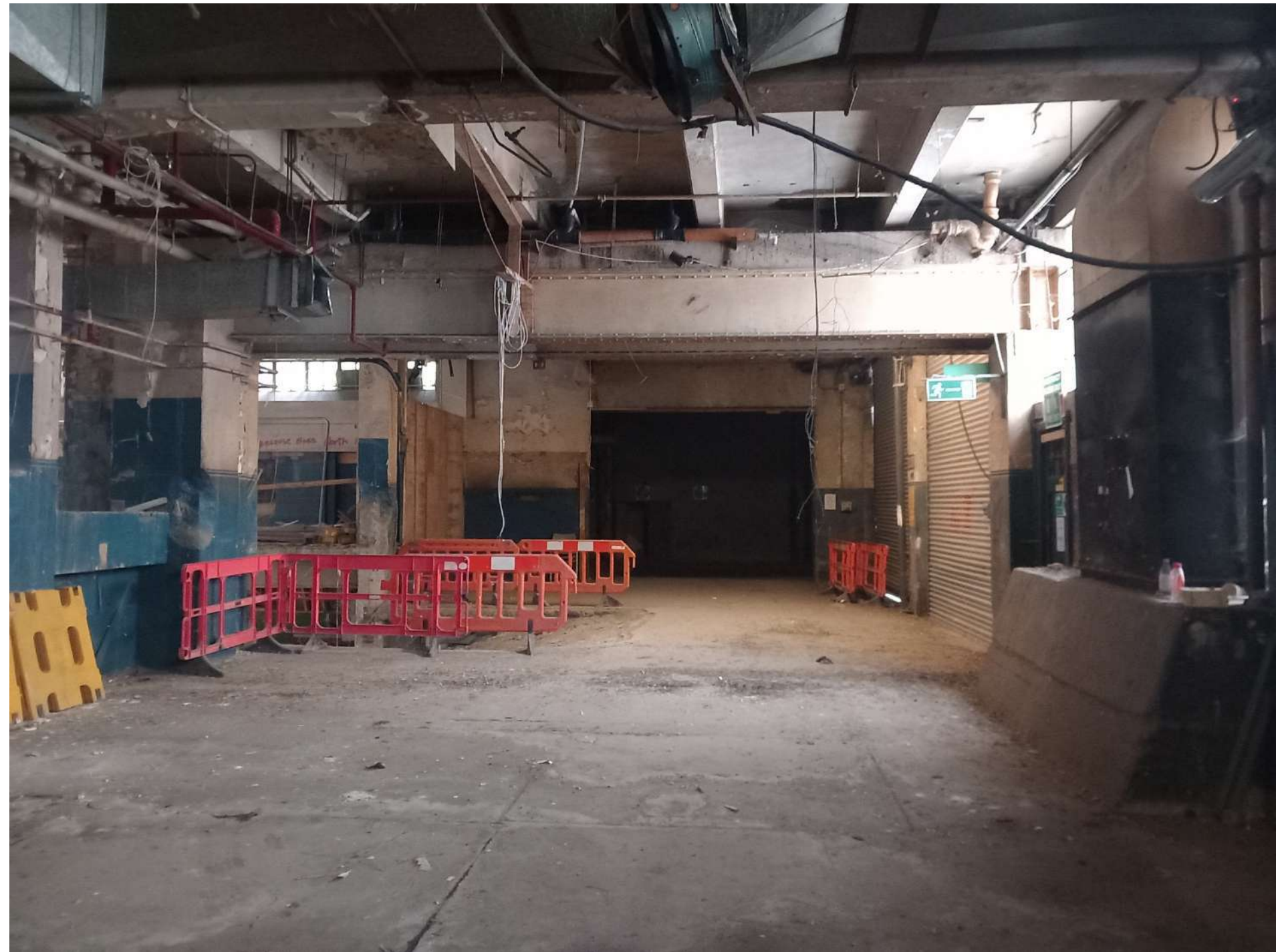
Plate 236: Zone 4, Ground Floor level, facing west. Steel girders spanning in an north-south direction, with concrete beams spanning east-west direction over.
