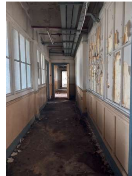
Plate 61: Original partition walls on either side of spine corridor with panelled wainscoting to lower level and multipaned glazed screens over. Panelled cross-corridor doors.
