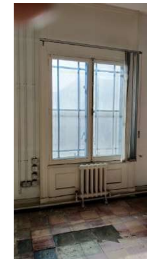
Plate 55: Original metal frames windows with margin lights externally, and timber-framed secondary glazing system with original ironmongery. Moulded architraves with panelled window apron.
