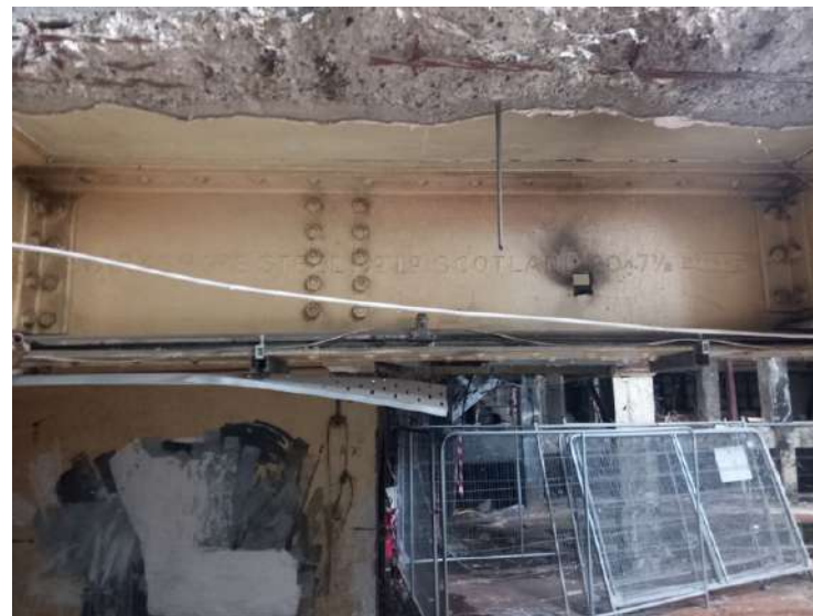
Plate 207: 'Lankarkshire Steel Co. Ltd., Scotland 20 x 7 1/2' marking on steel girders in Printing Hall.
