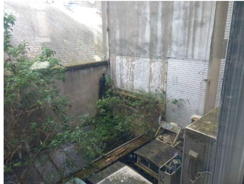
Plate 118: A series of lightwells introduce daylight between the rear range of buildings. The external walls are typically faced in a glazed white brick. This lightwell is positioned to the west of the return of Independent House, between the rear (south) wall of the Machine Room and 87-90 Middle Abbey Street.
