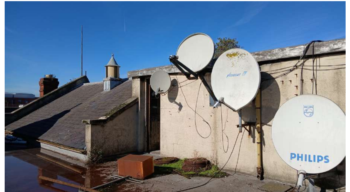
Plate 30: Roof access, at the top of the stairs, flanked by steeply pitched roof, having patent glazing on the north-facing pitch.
