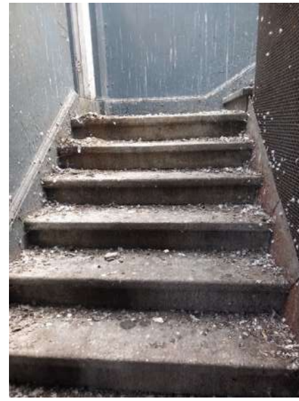
Plate 146: Granite threads to main stairs, with moulded timber skirting. Original lift, enclosed in steel cage positioned in central stairwell.
