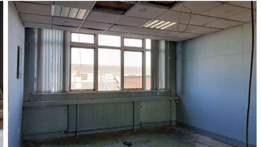
Plate 92: Replacement windows, contemporary wall linings and suspended ceiling at level 4.
