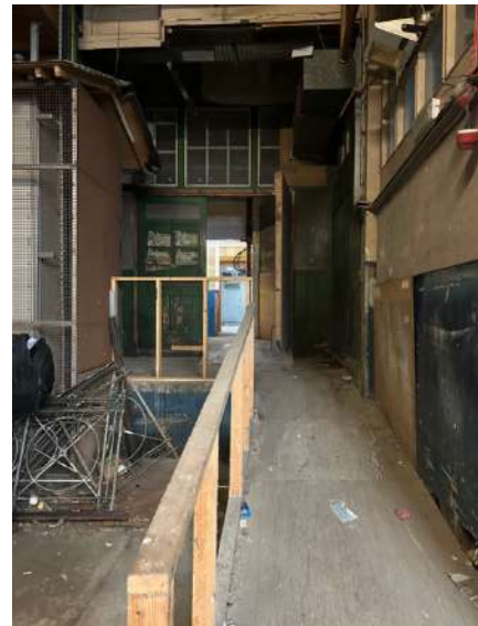
Plate 239: View of internal ramp, facing south. Original internal clerestory windows, and multiple contemporary interventions.
