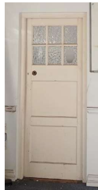
Plate 10 Typical original door: The original narrow panelled doors comprise of three panels, with six glazed panes in the upper panel. Circular brass knobs.
