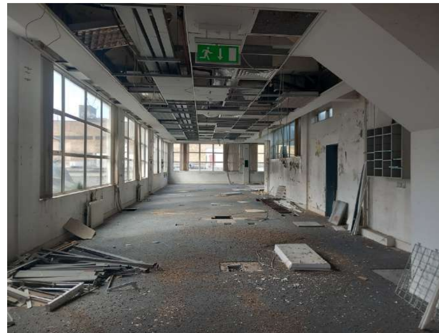
Plate 276: View facing west. uPVC windows, raised access floor, contemporary lay-in ceiling tiles.
