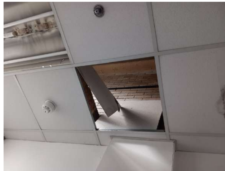
Plate 256: Detail of glazed brick finish to wall visible above contemporary suspended ceiling fabric in WCs.
