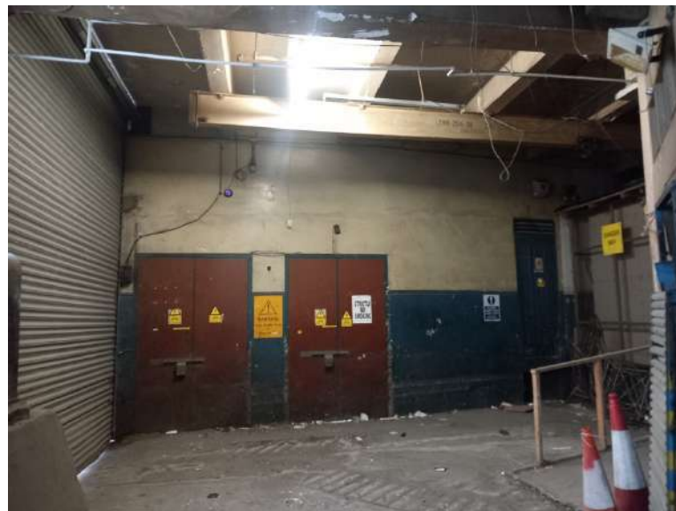
Plate 235: Zone 4, Ground Floor level, facing east. Former loading bay. Contemporary security shutter to Prince's Street. Girder is stamped 'Frodingham Iron and Steel Co Ltd. England.'
