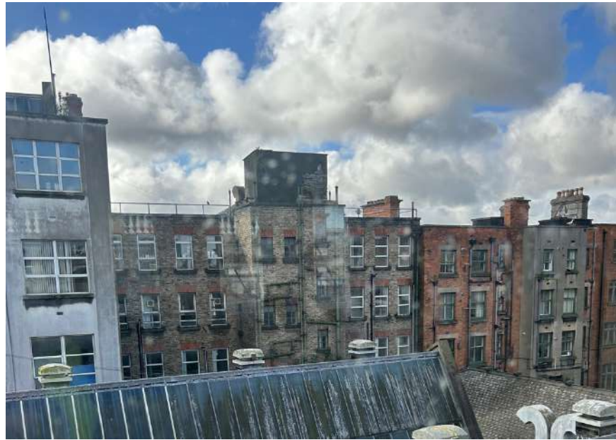
Plate 117: Rear façade of 87-90 Middle Abbey Street comprised of buff coloured brick with contrast red brick lintels. The rear windows have been replaced with contemporary frames throughout, except for the bathrooms on the return which have original steel multipaned frames.
