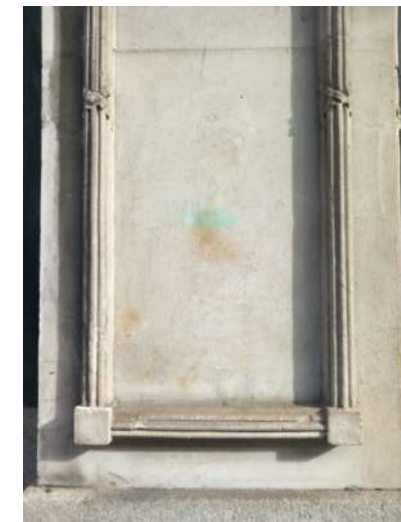
Plate 10: Detail of Portland Stone carving reeded panels with cable moulding and square blocks at junctions.
