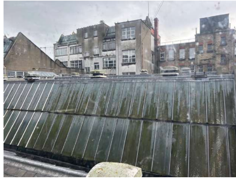
Plate 19: Rear façade of Independent House, with sawtooth profile roof of Machine Room in foreground.
