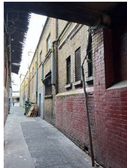
Plate 174: Stock brick wall finish, with contemporary windows on upper level.
