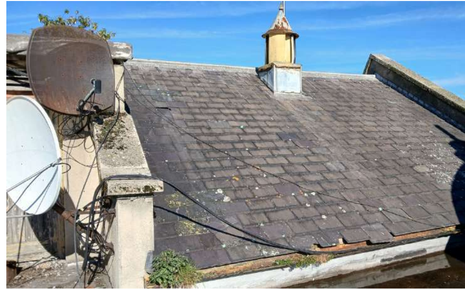
Plate 23: Steeply pitched roof to rear, east of roof access. Slate roof with rolled lead ridge and lead flashings. Original cone-topped vent.
