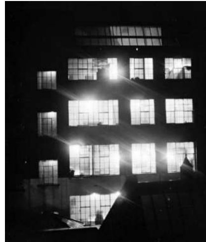
Plate 40: 1935 Photograph of the rear elevation of Independent House depicting the original thin frame metal windows with pivot opening sections, National Library of Ireland.
