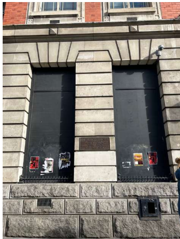
Plate 15: Detail of rusticated plinth, with inset postal box.
