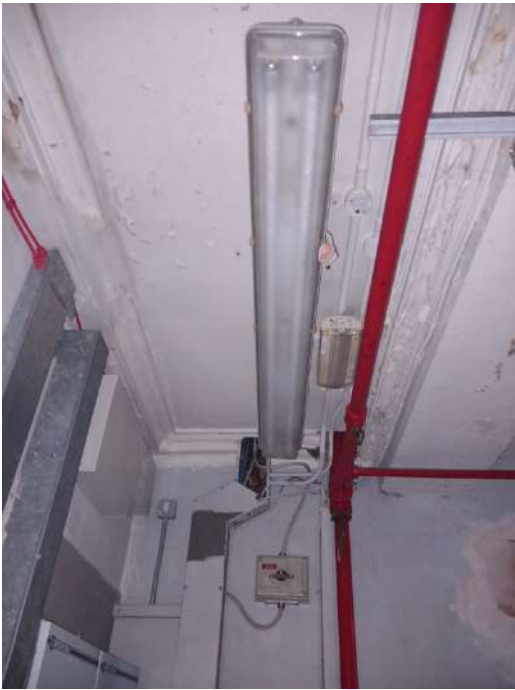
Plate 166: Plain run cornice on stair landing, interrupted by proliferation of later services.
