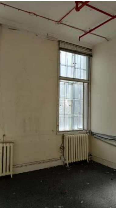
Plate 164: Cellular office. Plain run cornice, original metal windows with contemporary secondary glazing, surface mounted services. Later partition walls subdividing spaces.
