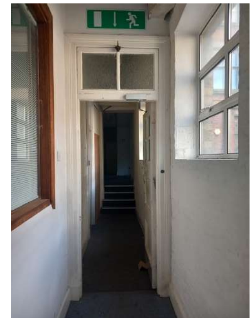
Plate 184: Original panelled door with 2 panelled pivot opening transom light over. Connection to rear of 91-92 Middle Abbey Street via steps beyond.
