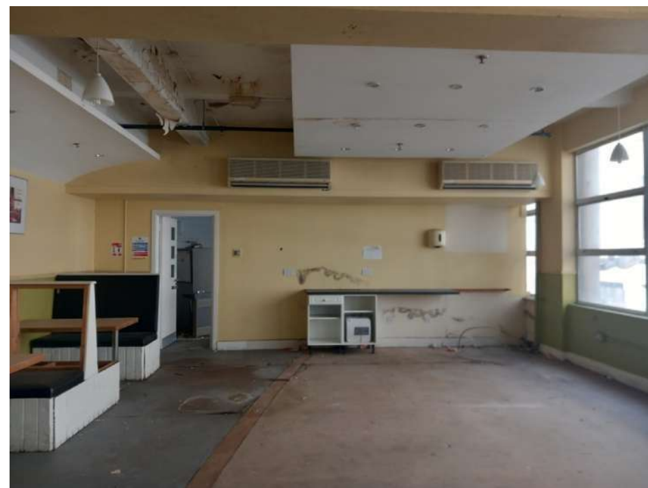
Plate 250: Zone 4. No historic architectural features of interest. uPVC windows, contemporary partitions, joinery and fixtures and plasterboard ceiling.
