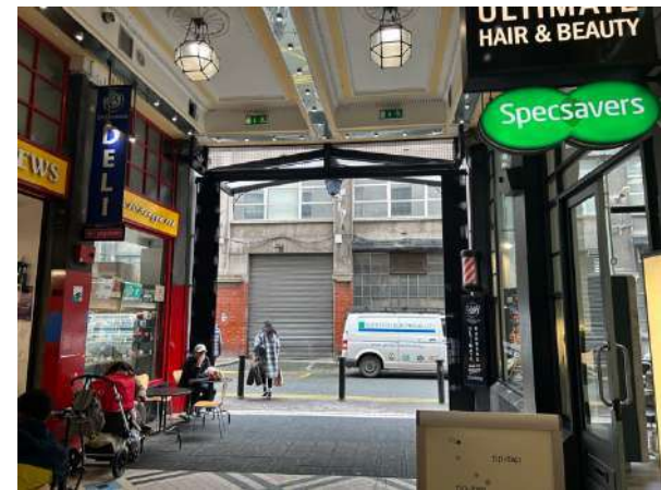
Plate 222: View of north façade of Zone 4 as viewed from within the GPO Arcade.
