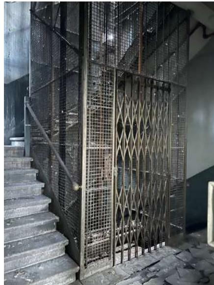
Plate 145: Projecting nosings on granite stair treads. Passenger lift with traditional cage structure rising through stairwell by Waygood Otis Ltd. Circular profile handrail fixed to lift enclosure.
