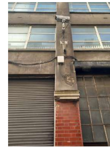
Plate 45: It is noted that the piers appear to be comprised of brick, with a render finish applied above. Surface mounted fixtures and fittings will be removed. The upper floors will be re-rendered, and the stepped lintels will be reinstated in their original location above the vehicular entrance.
