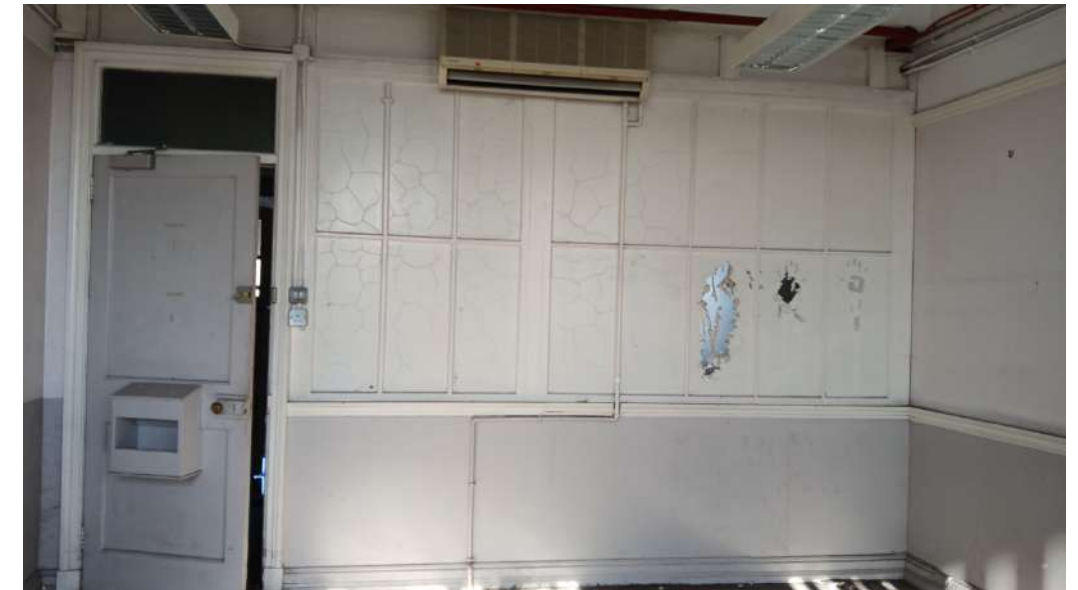
Plate 72: Typical cellular office facing south onto Middle Abbey Street. Original metal window frames. Original skirting, dado and picture rails. Evidence of water damage internally.
