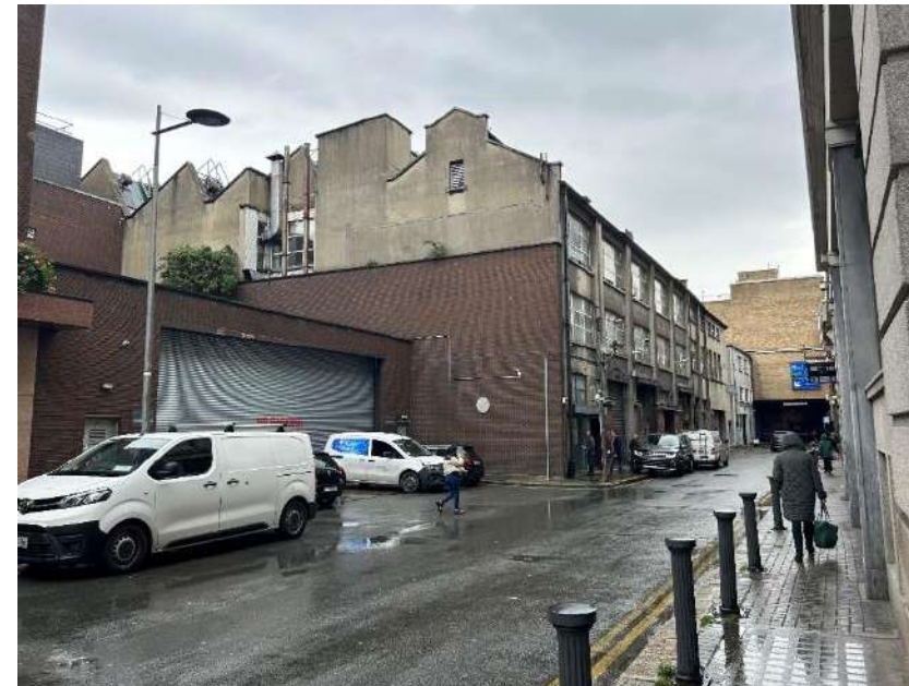
Plate 30: View of the building range from within Princes Street North
