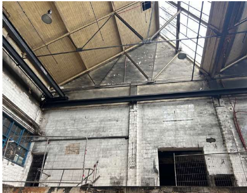
Plate 191: View from lower ground level, at south-western end of Printing Hall facing west towards upper ground level gallery. Masonry columns clad in white glazed tile supporting steel trusses of sawtooth roof.
