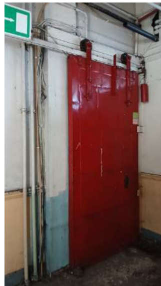
Plate 63: Typical steel fire door, on sliding mechanism, separating Independent House and Emerald Chambers.
