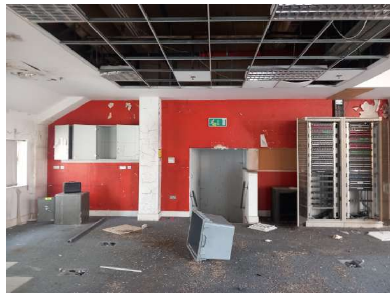
Plate 271: View facing east. uPVC windows, raised access floor, contemporary lay-in ceiling tiles. Former open plan office space.
