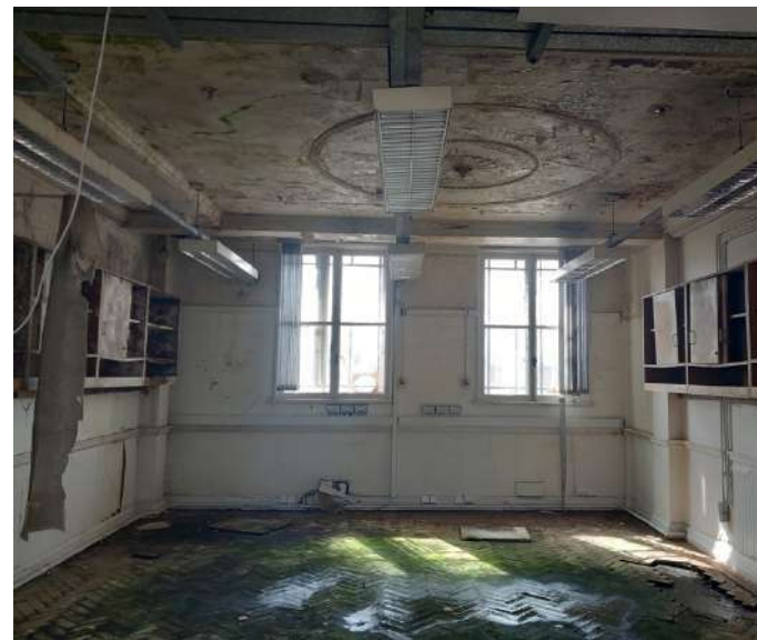
Plate 79: View facing north in former boardroom. Original secondary glazing system on Middle Abbey Street. Timber casements internally with cast iron frames externally, all with original ironmongery. Moulded timber skirting, dado and picture-rail. Neo-classical plasterwork to ceiling in regency style. Original parquet floor, damaged by water ingress. Exposed contemporary services throughout.
