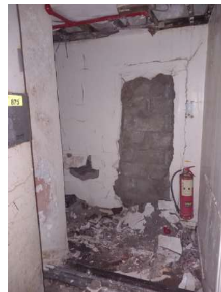
Plate 142: Rear ground floor of 87-90 Middle Abbey Street. Blockwork infilled opening.
