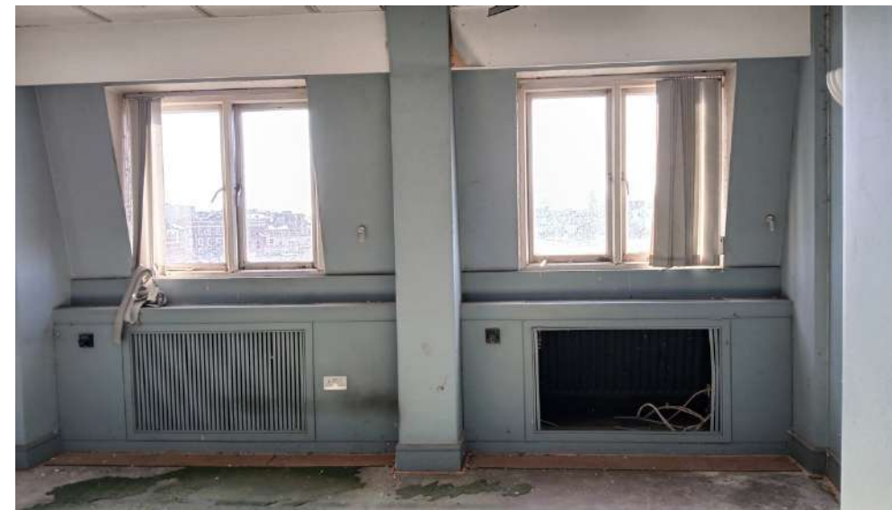
Plate 88: Replacement timber windows at fourth floor level. Contemporary wall linings.
