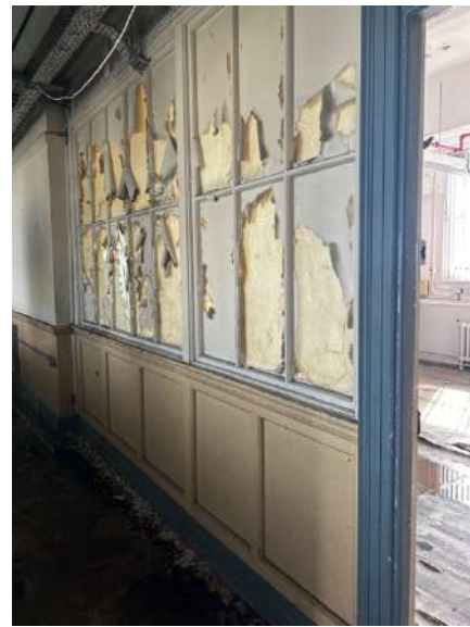
Plate 60: Original partition wall in corridor with panelled wainscoting to lower level and multipaned glazed screens over. Original moulded timber architraves and skirtings.
