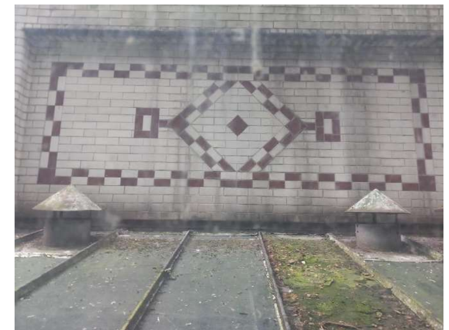
Plate 20: This eastern face of the machine hall is clad in glazed white brick and features a decorative geometric pattern on the panels between the piers.
