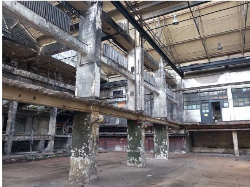
Plate 199: View from western side of Printing Hall towards south east. The central row of masonry column subdivide the hall; cartographic research suggests that the western side of the hall was a later addition. The columns supported a gallery at upper ground level, now demolished.
