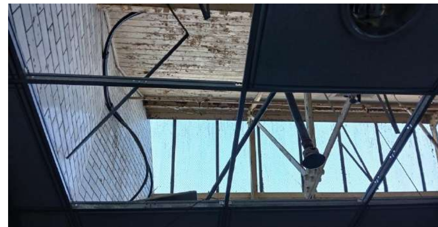
Plate 43: The patent glazing with wired glass on the main roof will be replaced with a new glazing system. The metal truss structure and slate linings on the south slope will be retained and repaired and the contemporary suspended ceiling will be removed.
