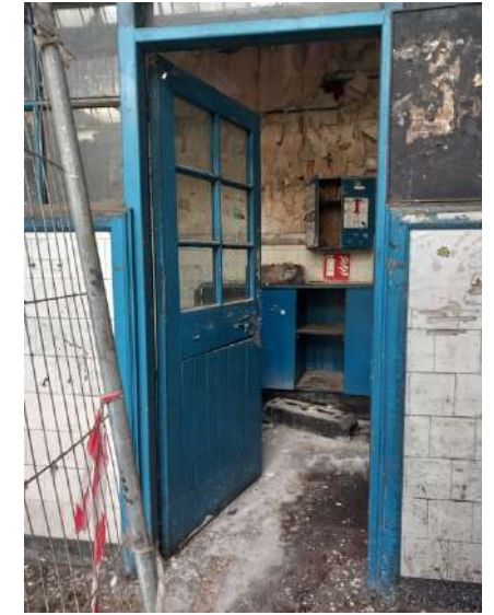
Plate 205: Original timber doorset with vertical boarded to lower panel and glazed upper panel, subdivided into six panes. Internal walls lined with square format glazed white tile.
