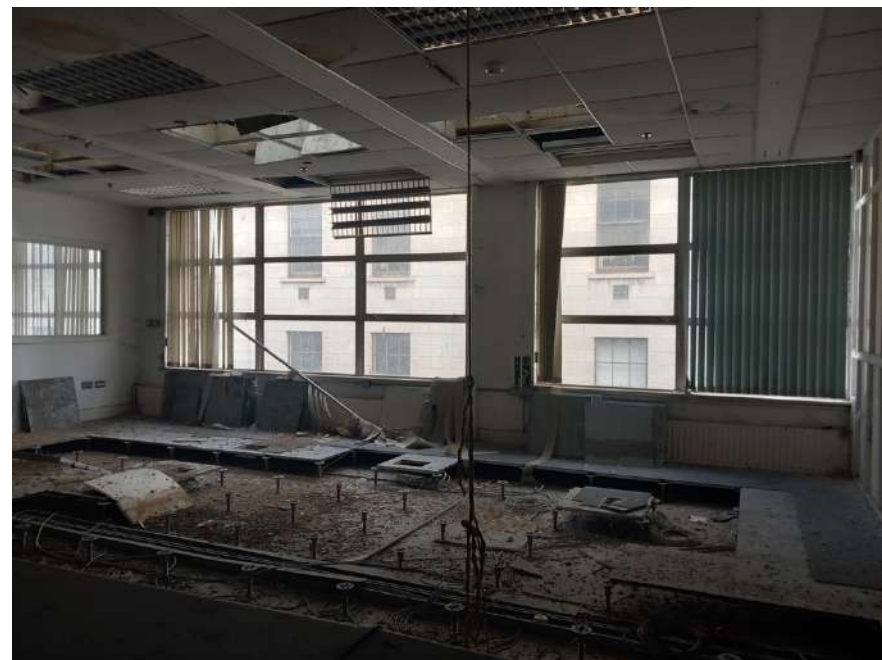
Plate 265: Facing north towards GPO on opposite of Prince's Street North. Contemporary finishes throughout; uPVC windows, suspended ceiling, raised access floor.
