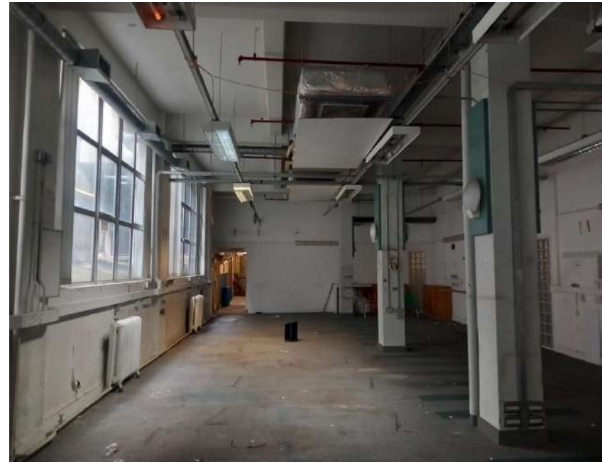
Plate 22: Typical open plan floor within Area 4
