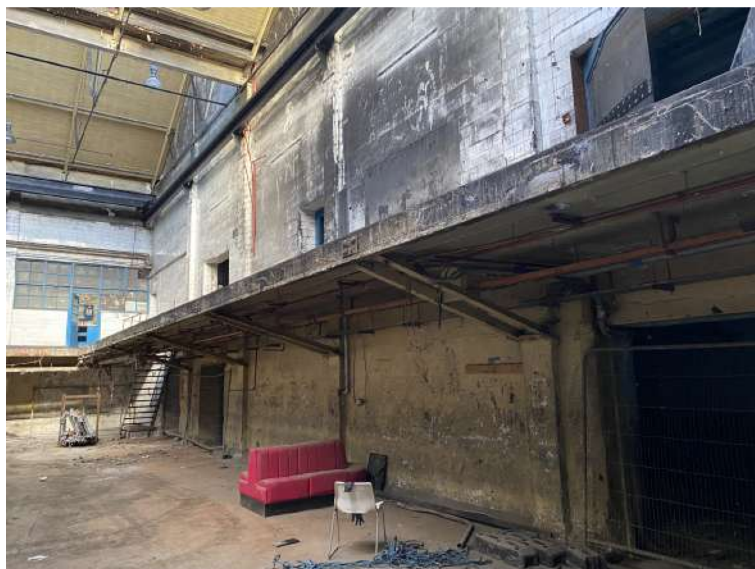
Plate 3: Western section of main basement, facing southwest
