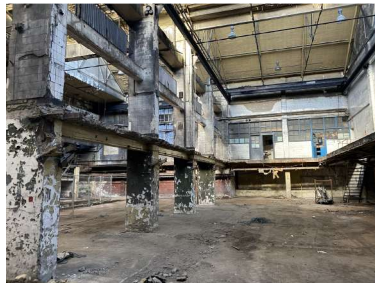
Plate 4: Eastern section of the basement, facing south
